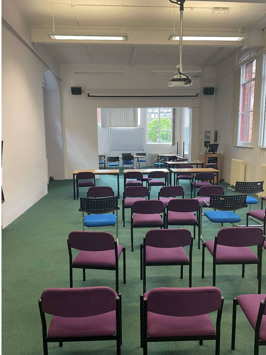
Photo 1. Opening in internal wall in G.046 G.046A, from G.046 side
