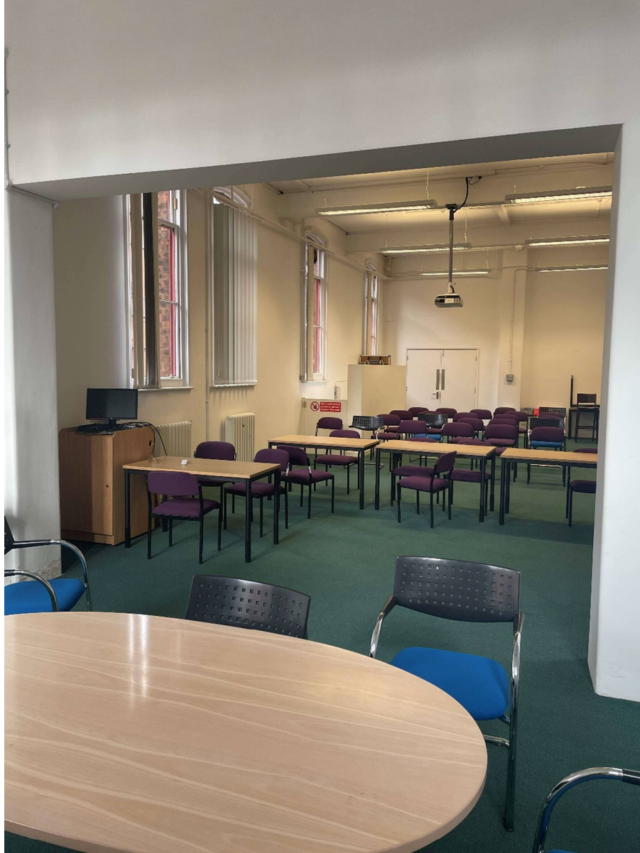
Photo 2. Opening in internal wall in G.046 G.046A, from G.046A side
