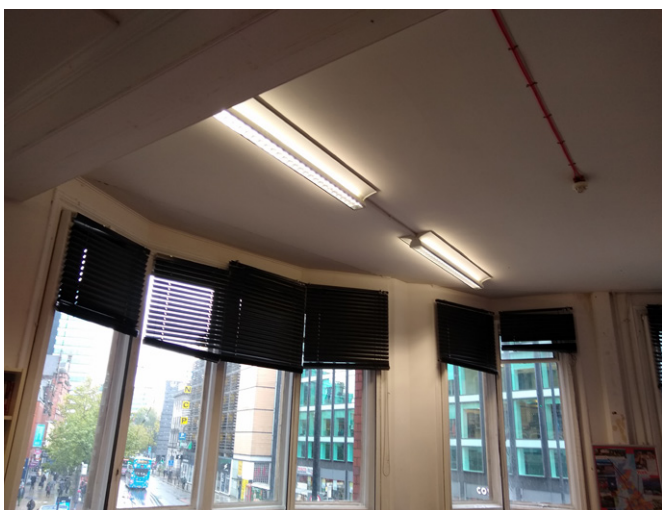
Images 19, 20, 21: Showing typical sash windows (upper floors), example of internal windows from stair well to inner office, and view of later date metal framed windows at first floor (to be replaced).
