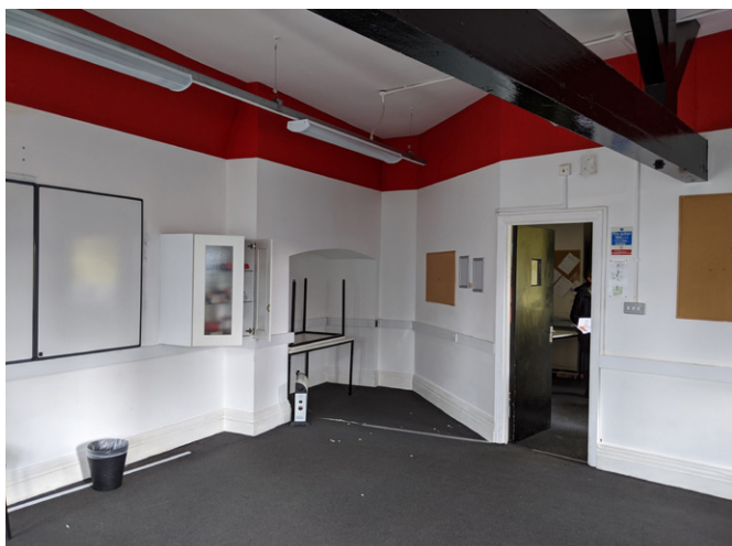
Image 12: Photograph of fourth floor showing exposed timber roof structure. Raised floors will allow ceilings to remain exposed.
