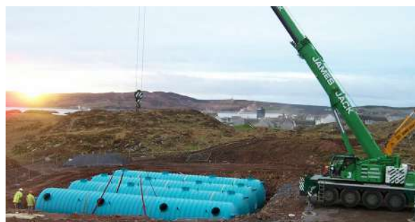
SPEL Septic Tanks 600 Series 240,000 litre Port Ellen, Islay, Western Isles
