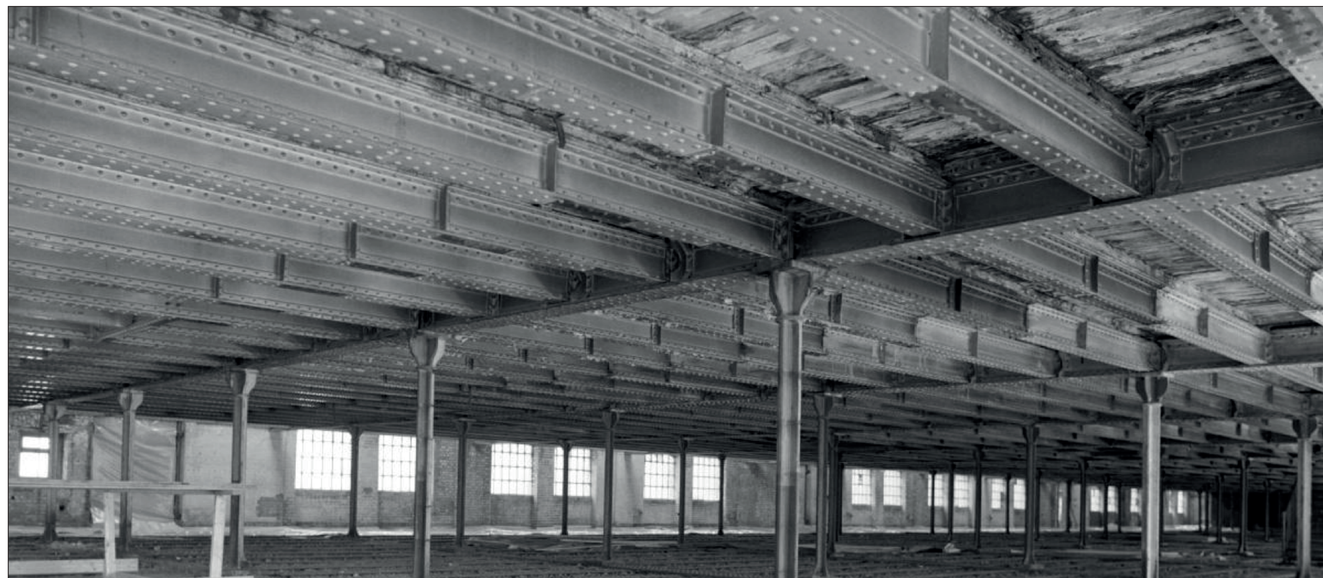
Image 51: View of interior of New Warehouse showing structural elements, prior to redevelopment as museum, 1980s.
