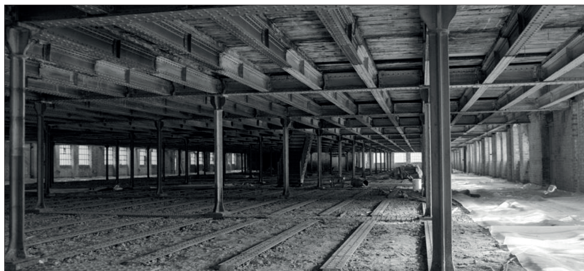
Image 7 (above): Showing example interior of New Warehouse on upper floor, refurbished and currently used as venue space.
