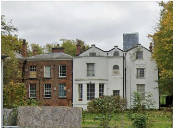
5. Hulme Barracks - rear facade facing the site
