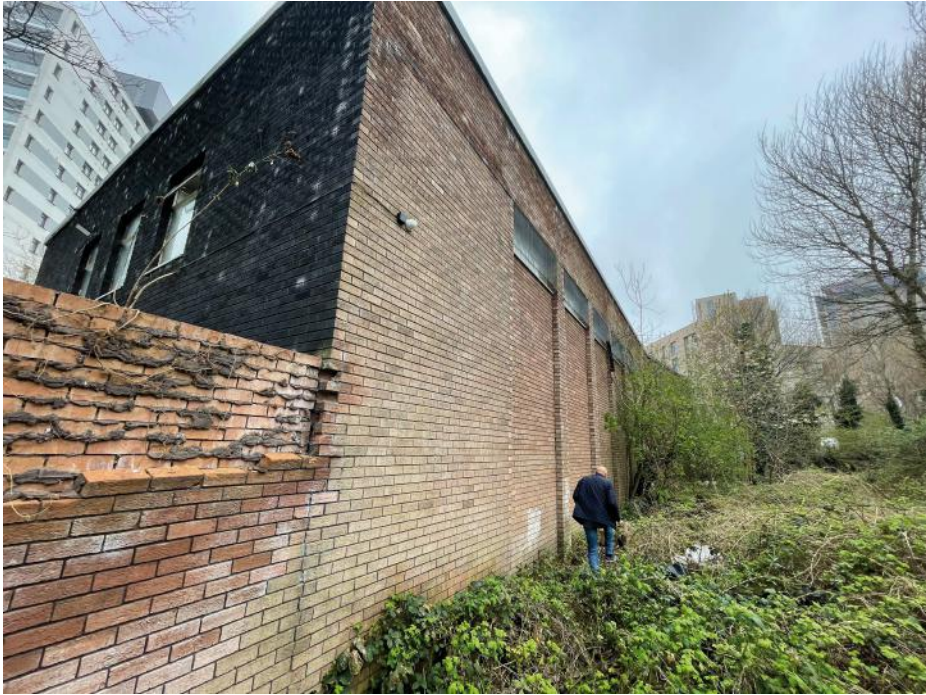
6. Rear wall of Palmer House from southeast
