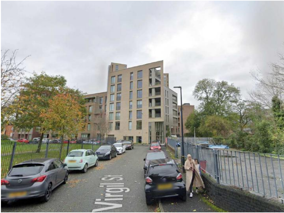
2. View towards northwest along Virgil Street towards Botanica apartments
