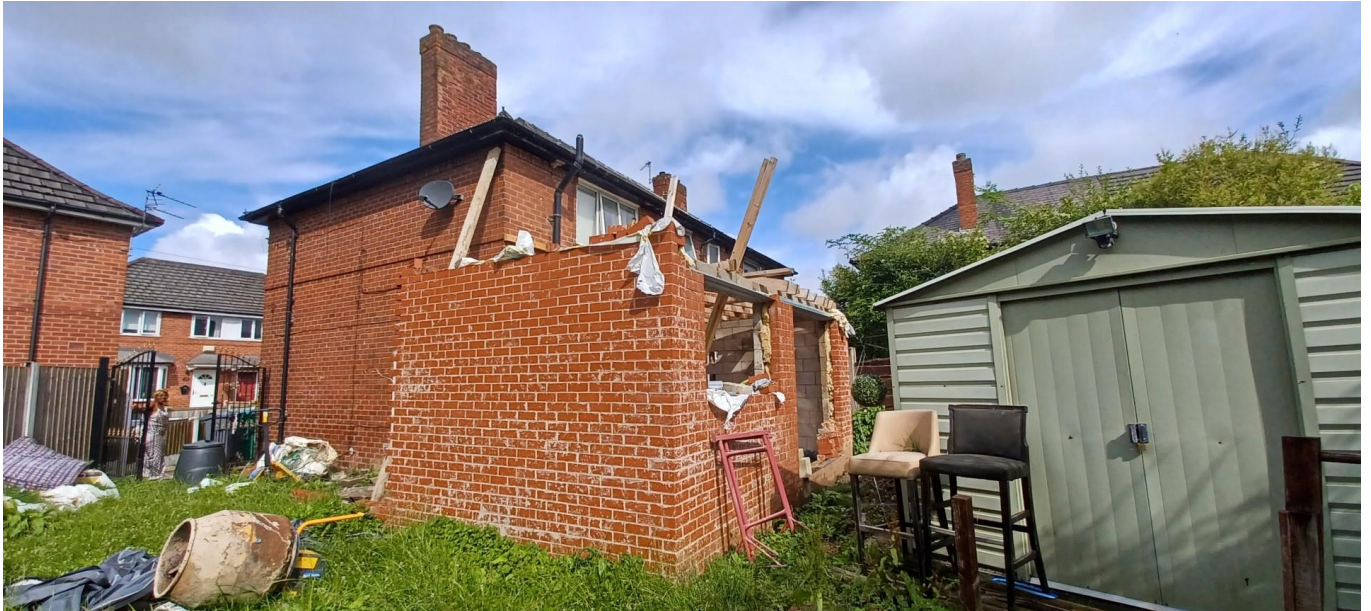
Figure 2. Rear of property.
