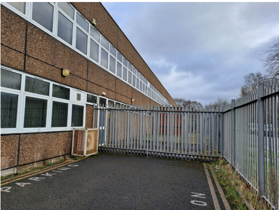
5. Internal View - Wavell Road elevation, palisade fencing
