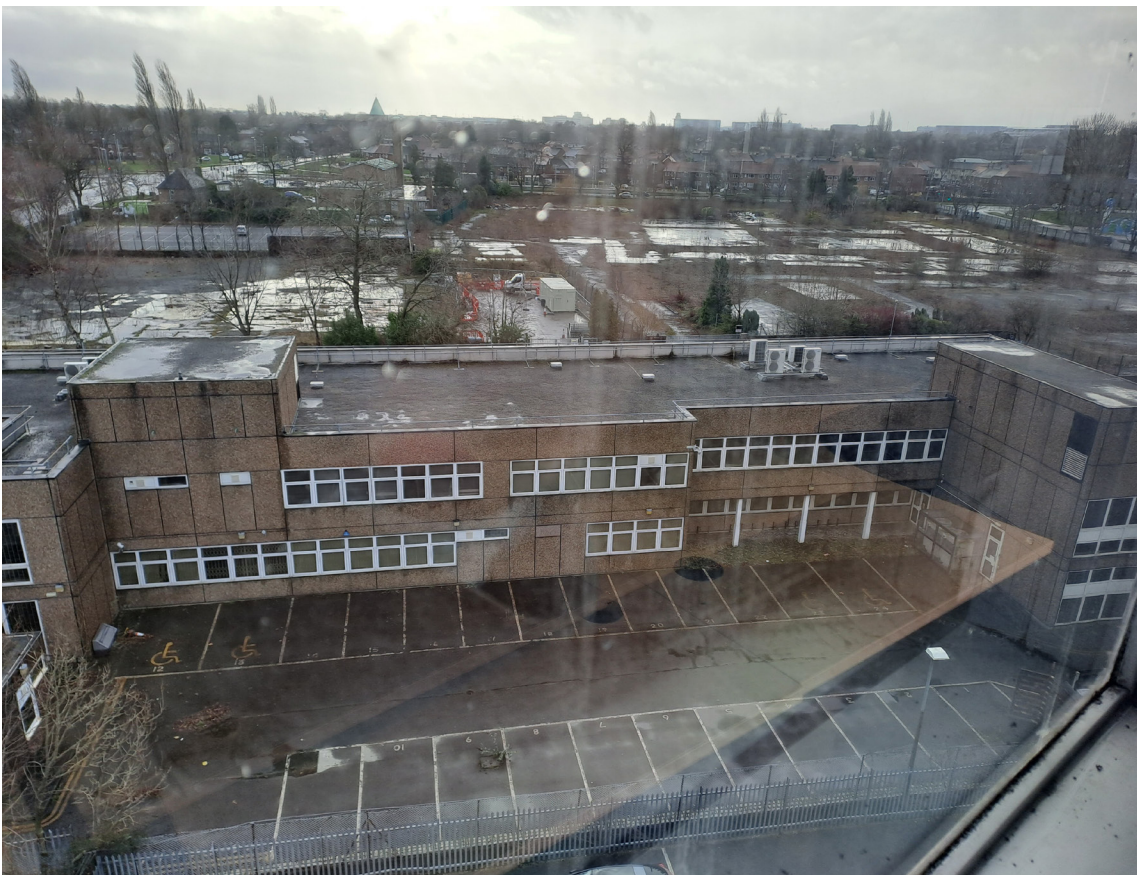
6. Internal View - from Delta House towards Simon House and vacant site off Wavell Road
