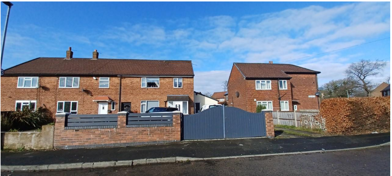
Figure 1. Principal elevation of No.65 Crowland Road.
