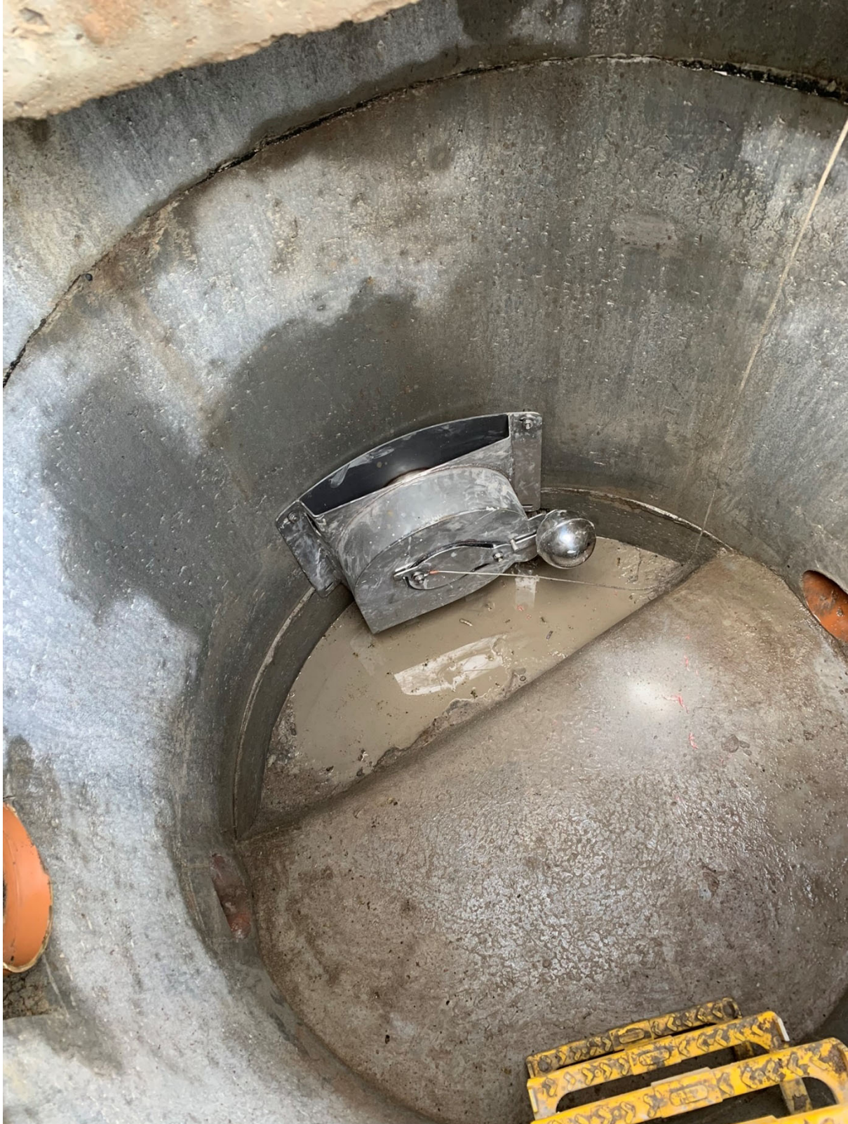
Hydrobrake installation
