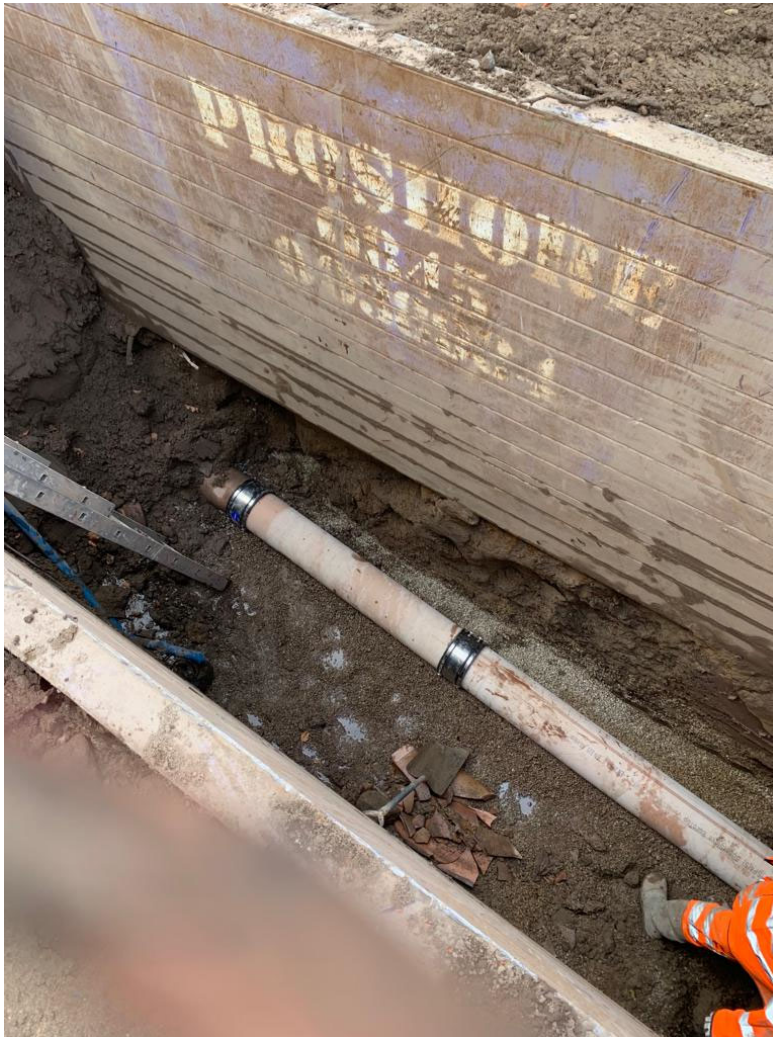
Picture 1 – installation of the pipe works and concrete ring manholes
