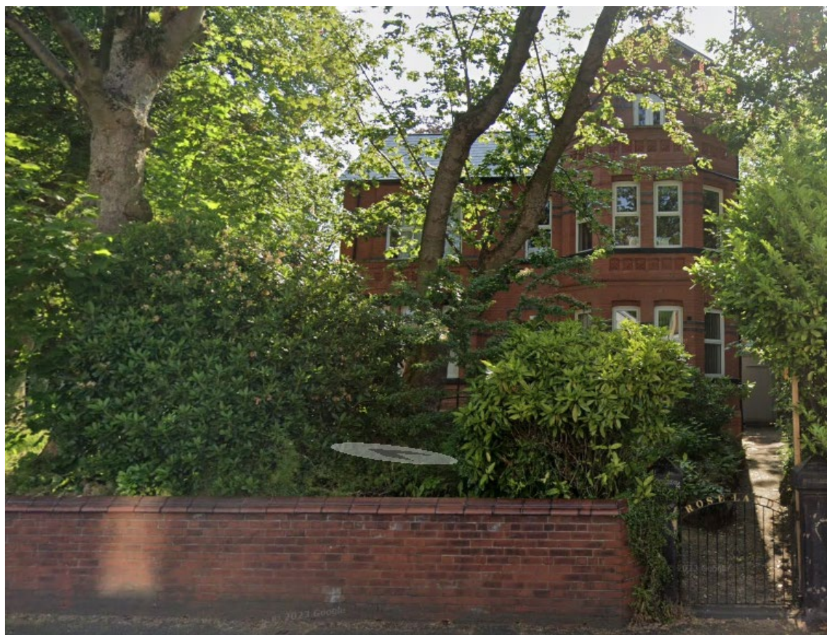
1 View of the front of the main building from Middleton Road
