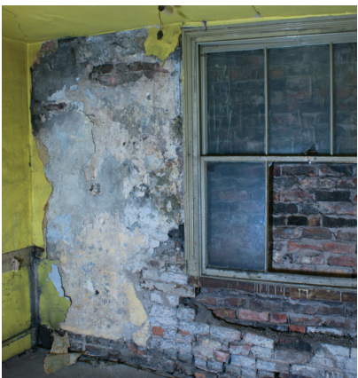
06 EXISTING REAR WALL AND WINDOW. THE WINDOW OPENING, WHICH HAS BEEN BRICKED UP PREVIOUSLY, IS PROPOSED TO BE REIN- STATED WITH THE EXISTING HISTORICAL WINDOW TO REPAIRED TO MATCH THE ORIGINAL DESIGN INTENT
