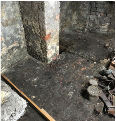
04 ORIGINAL BRICK FLOORING IS VISIBLE THROUGH THE DIRT FLOOR. UPON INSPECTION, THE BRICKWORK IS SATURATED WITH WATER AND BREAKS APART EASILY SO IS UNFORTUNATELY UNSUITABLE FOR RE-USE. BRICK FLOORING WILL BE CHOSEN TO REPLICATE THE ORIGINAL INTENT / LAYING PATTERN.
