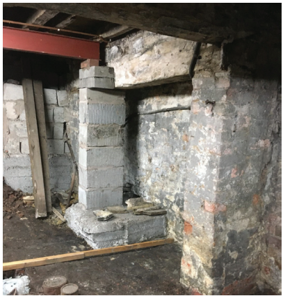
03 ORIGINAL STONE RANGE, WHICH IS PROPOSED TO BE LEFT AS EXISTING IN THE FINAL SCHEME
