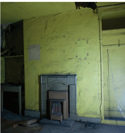
05 1950s MOCK FIRE SURROUND, WHICH IS DEEMED AS MEDIUM SIGNIFICANCE DUE TO IT NOT BEING AN ORIGINAL FEATURE OF THE BUILDING, IS PROPOSED TO BE REMOVED AND REPLACED WITH A RECLAIMED CAST-IRON SURROUND.
