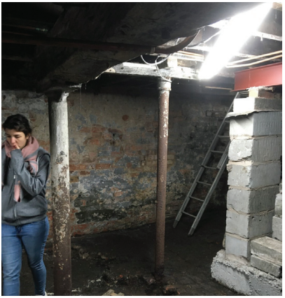
02 THERE ARE 3NO. ORIGINAL CAST IRON COLUMNS PRESENT AT BASEMENT LEVEL. ALL COLUMNS ARE PROPOSED TO BE LEFT EXPOSED IN THE FINAL SCHEME (STRIPPED AND PAINTED WITH INTUMESCENT PAINT FOR COMPLIANCE WITH BUILDING REGULATIONS)
