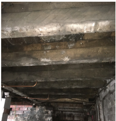
05 THE LEVEL 00 FLOOR / BASEMENT CEILING IS ALL ORIGINAL WOODWORK INCLUDING BEAMS AND FLOORBOARDS. THIS WILL BE RETAINED AND SUPPORTED FROM NEW STRUCTURAL ELEMENTS WHERE REQUIRED AND LEFT EXPOSED IN THE FINAL SCHEME.
