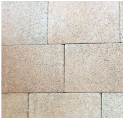
Concrete paving to primary routes
