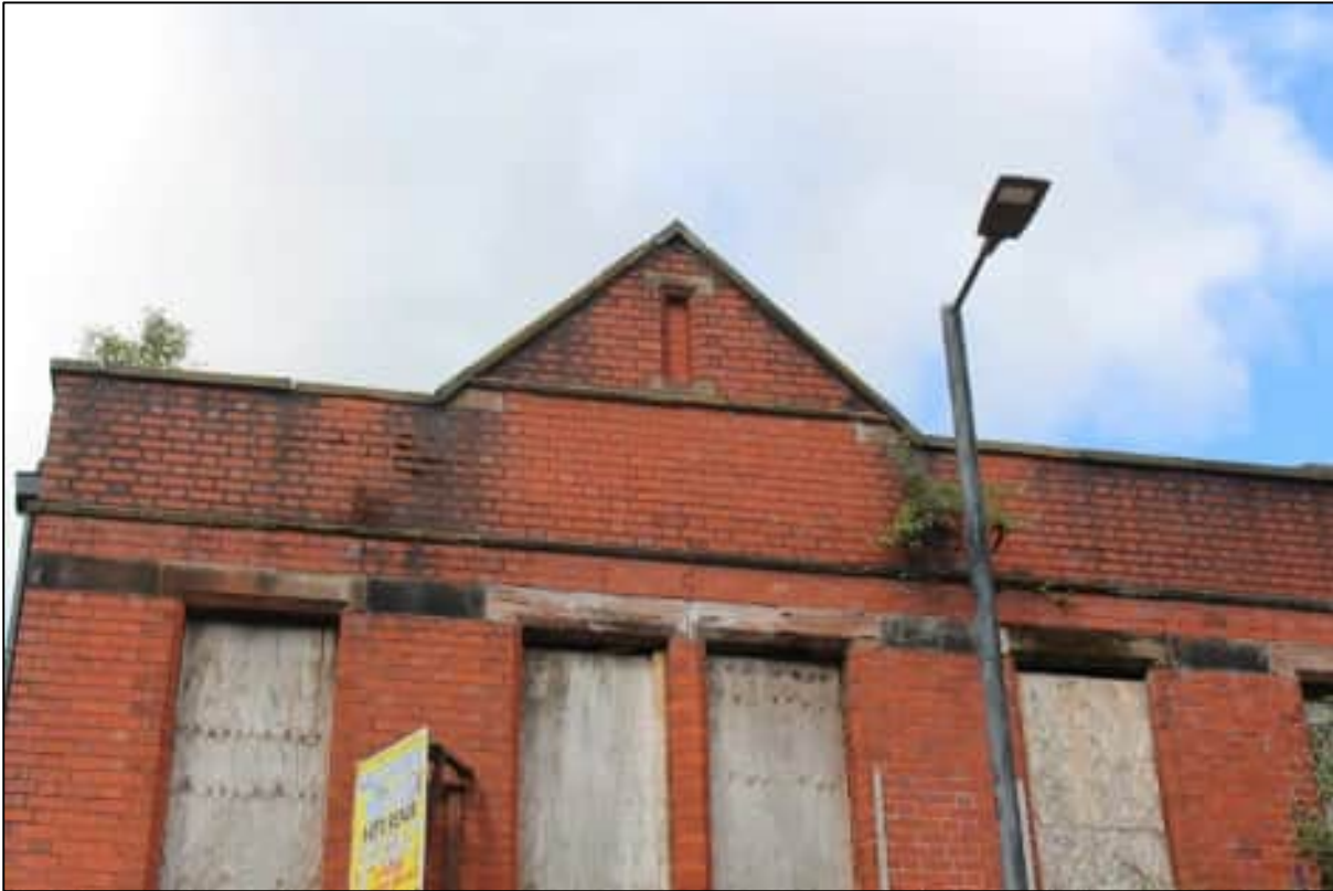
Plate 11: Detail of the gablet to the original office buildings eastern elevation, looking west
