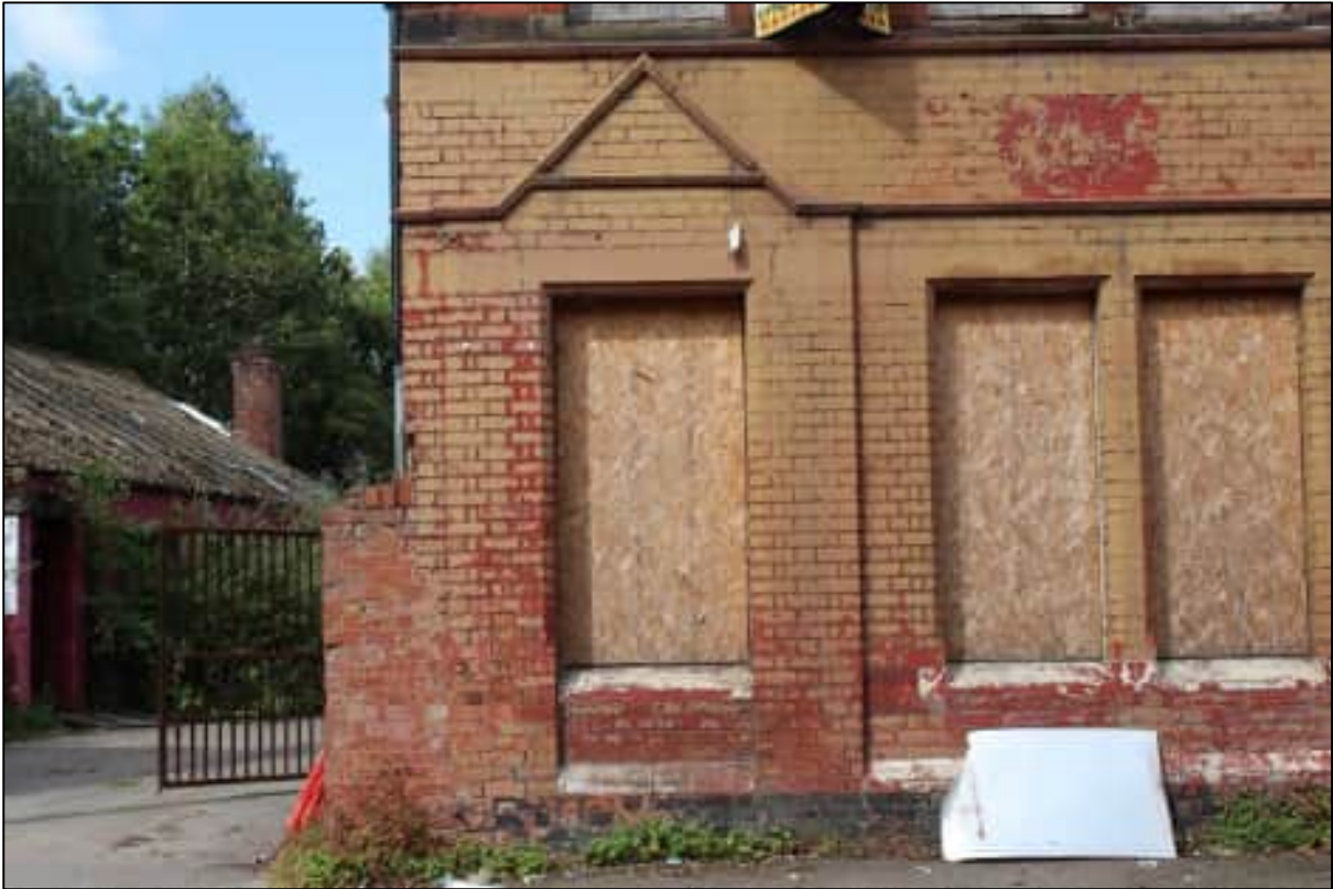
Plate 8: Detail of the southern ground floor window of the office building, looking west
