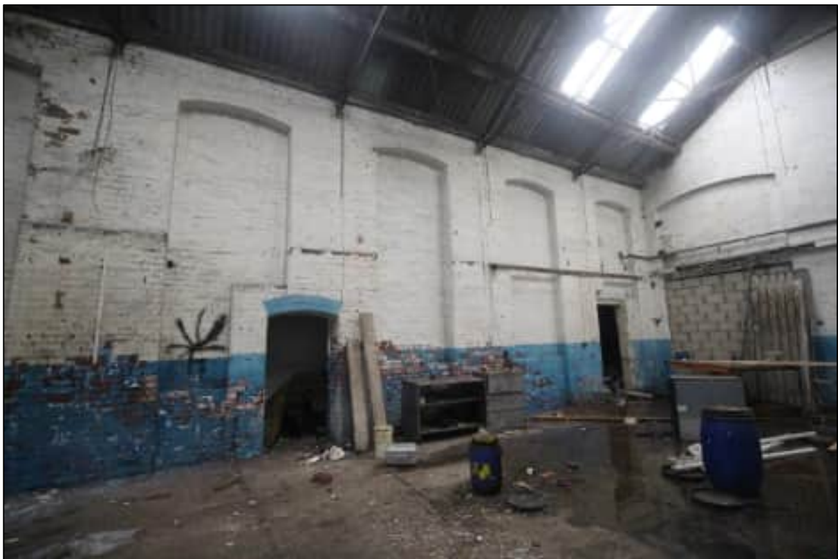
Plate 64: The northern wall of the 1903 extension, looking north-east
