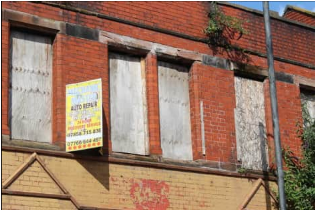
Plate 10: Detail of the first floor windows to the eastern elevation of the original office building, looking north-west
