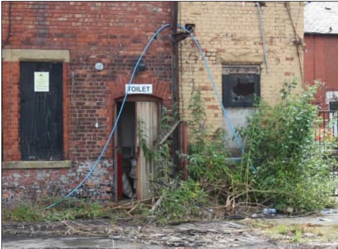
Plate 24: The doorway to the southern end of the western elevation of the 1892 office building, looking east
