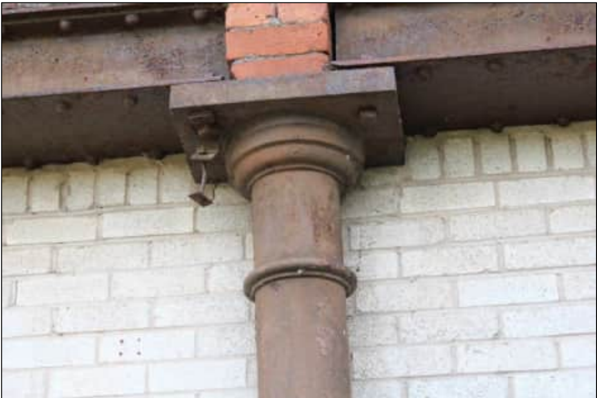
Plate 28: Detail of the column capital to the ground floor bays
