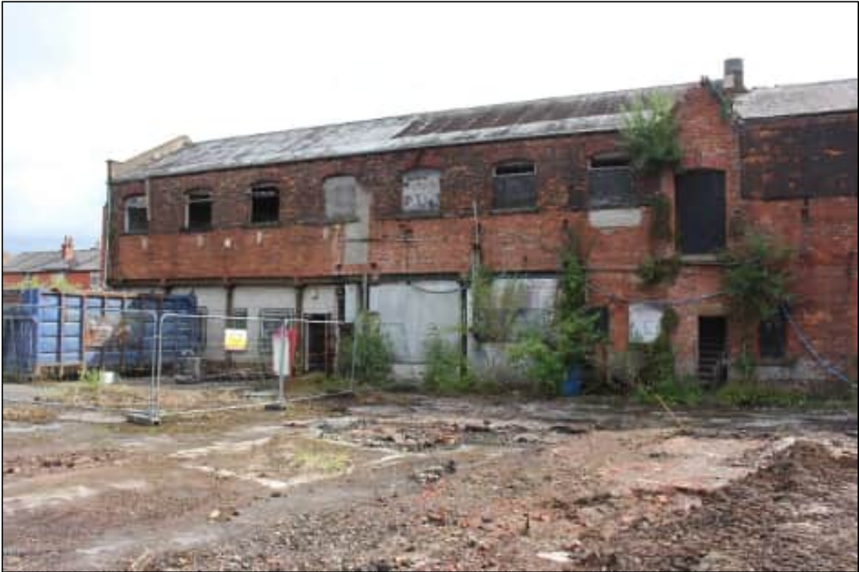
Plate 27: The western elevation of the 20 th -century extension, looking north-east
