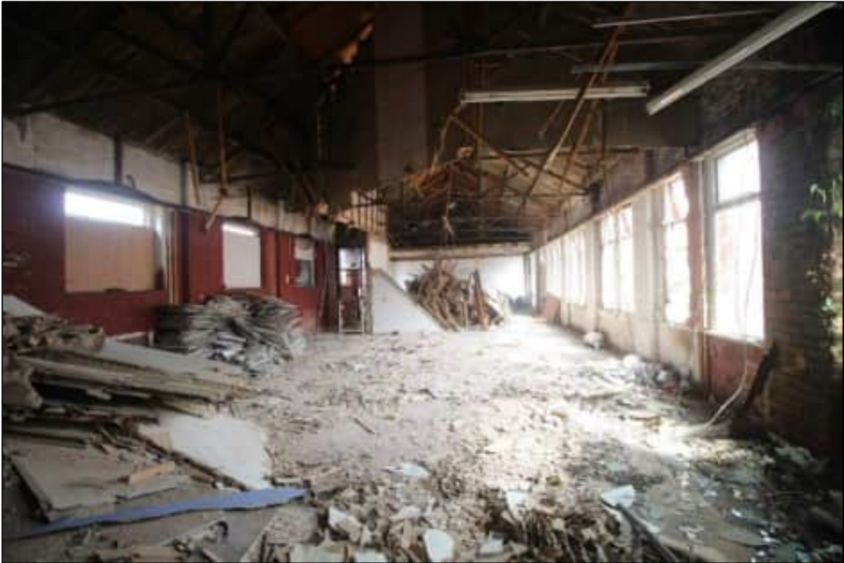
Plate 40: General view of the first floor of the 20 th -century extension, during the soft strip, looking north
