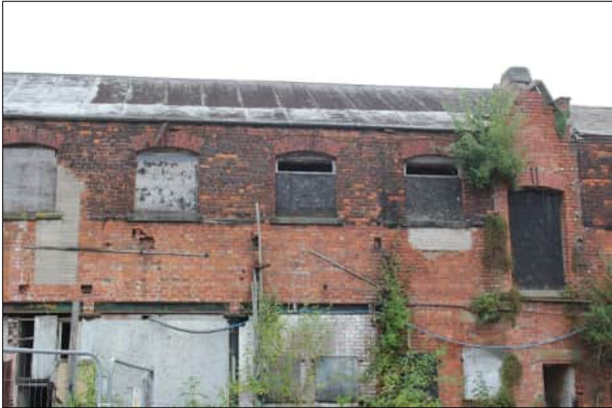
Plate 26: The first floor windows on the western elevation of the office building extension, looking east
