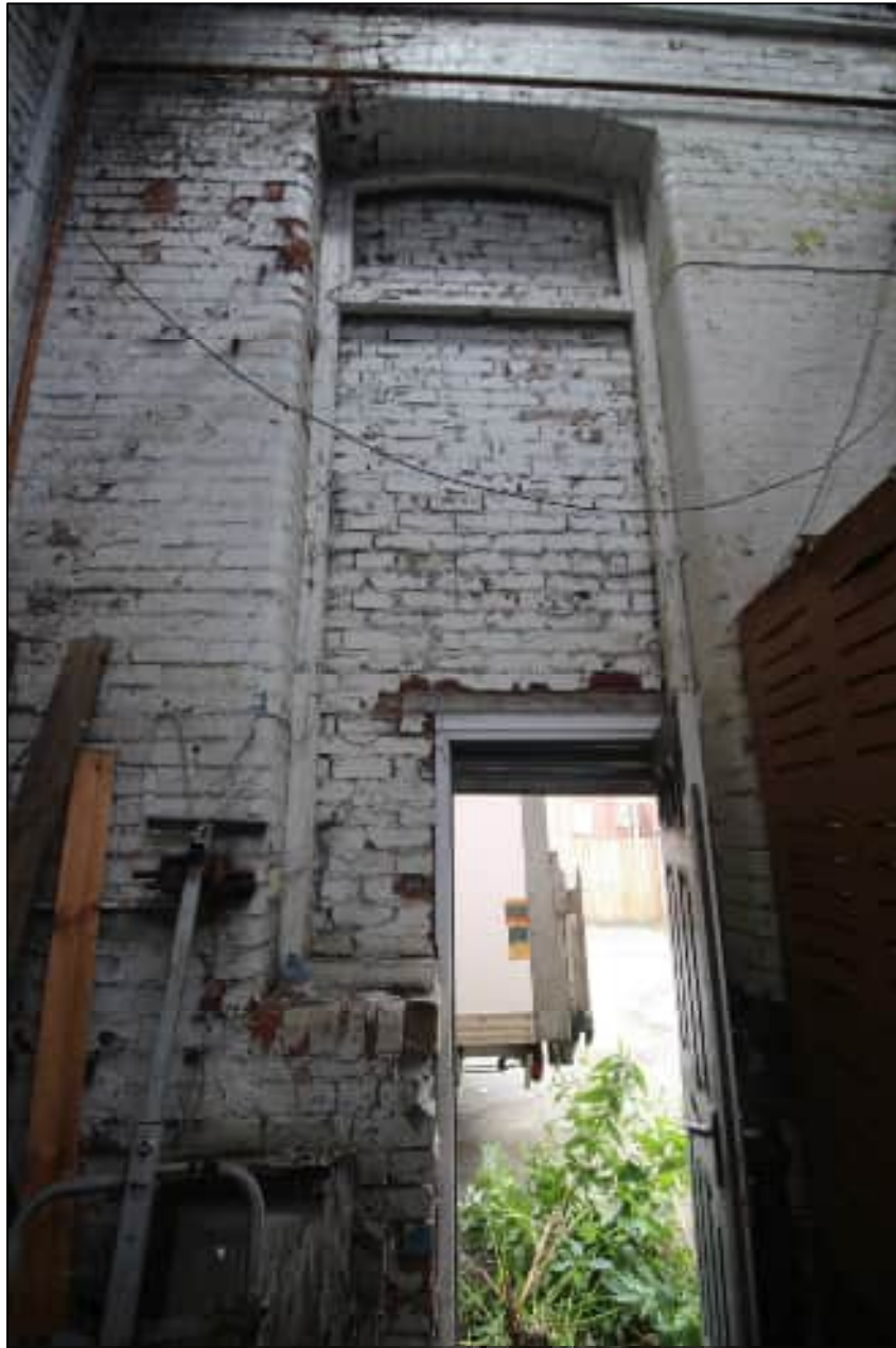
Plate 59: The remodelled northern window within the eastern wall of Room 1, looking east
