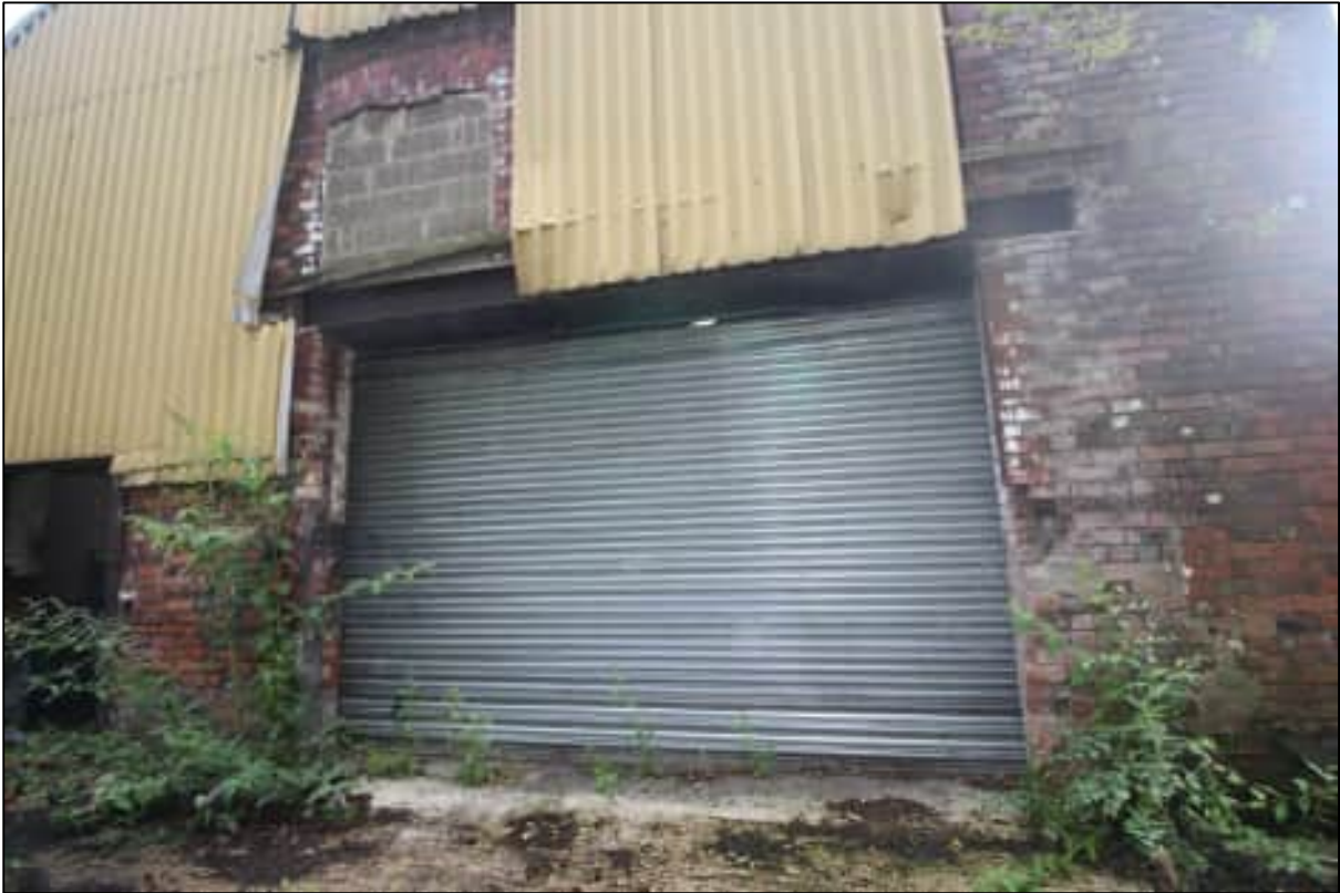
Plate 51: The southern gable detailing the later inserted vehicle doorway with the blocked window aperture above, looking east
