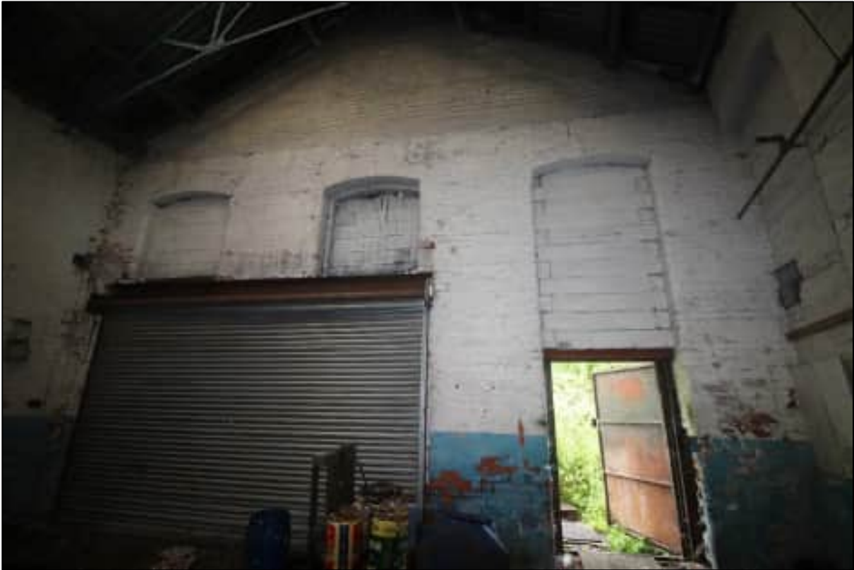
Plate 67: The western wall of the 1903 extension, looking west
