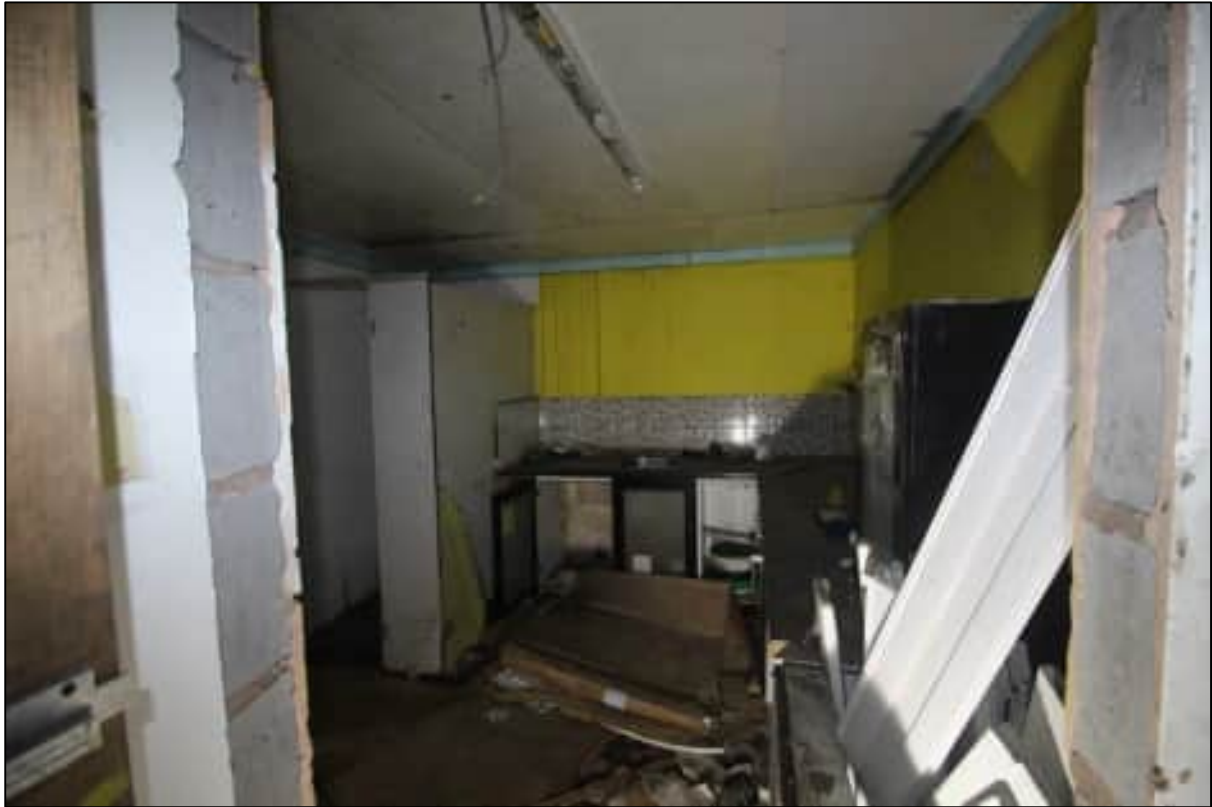
Plate 61: General view of Room 2, looking north
