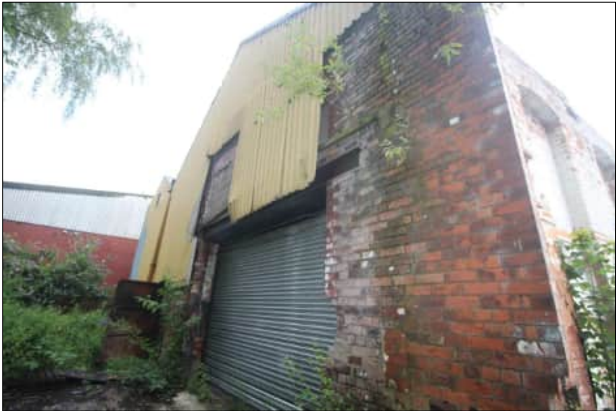
Plate 50: General view of the western elevation, looking north-east
