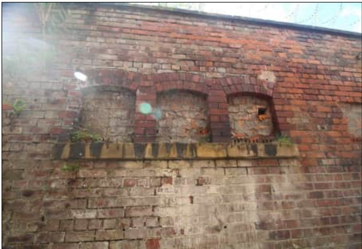
Plate 53: Detail of the blocked windows to the northern elevation of the original workshop, looking south
