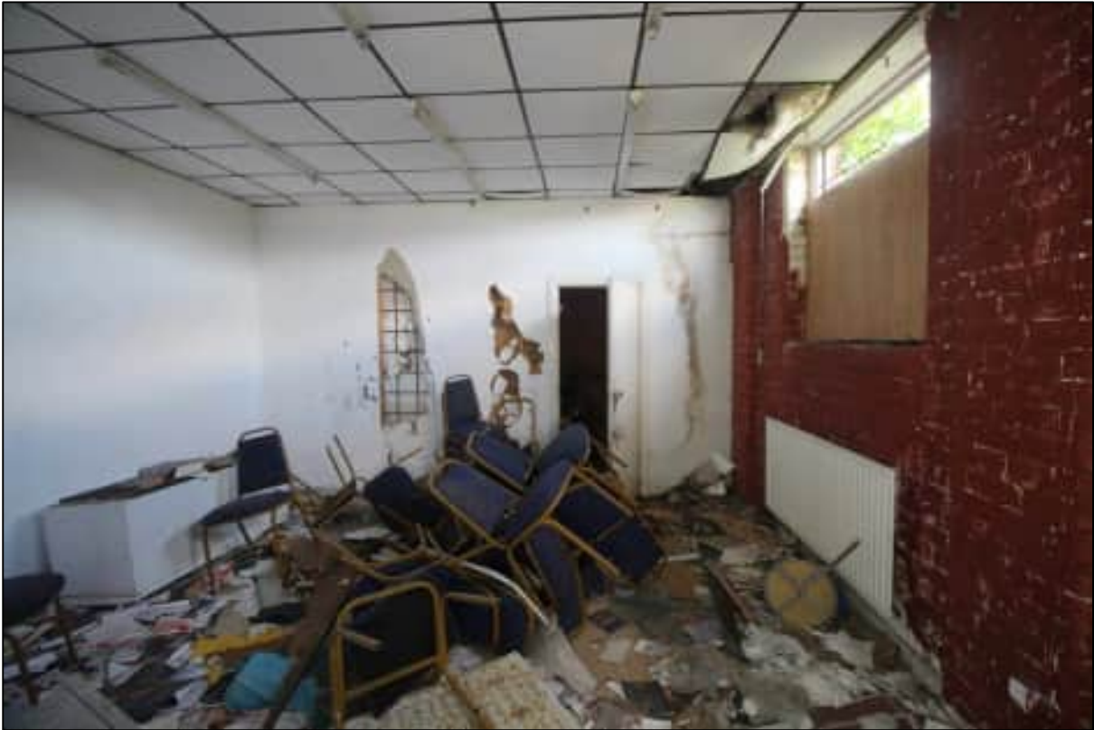
Plate 39: General view of Room 18, prior to the soft strip, looking south
