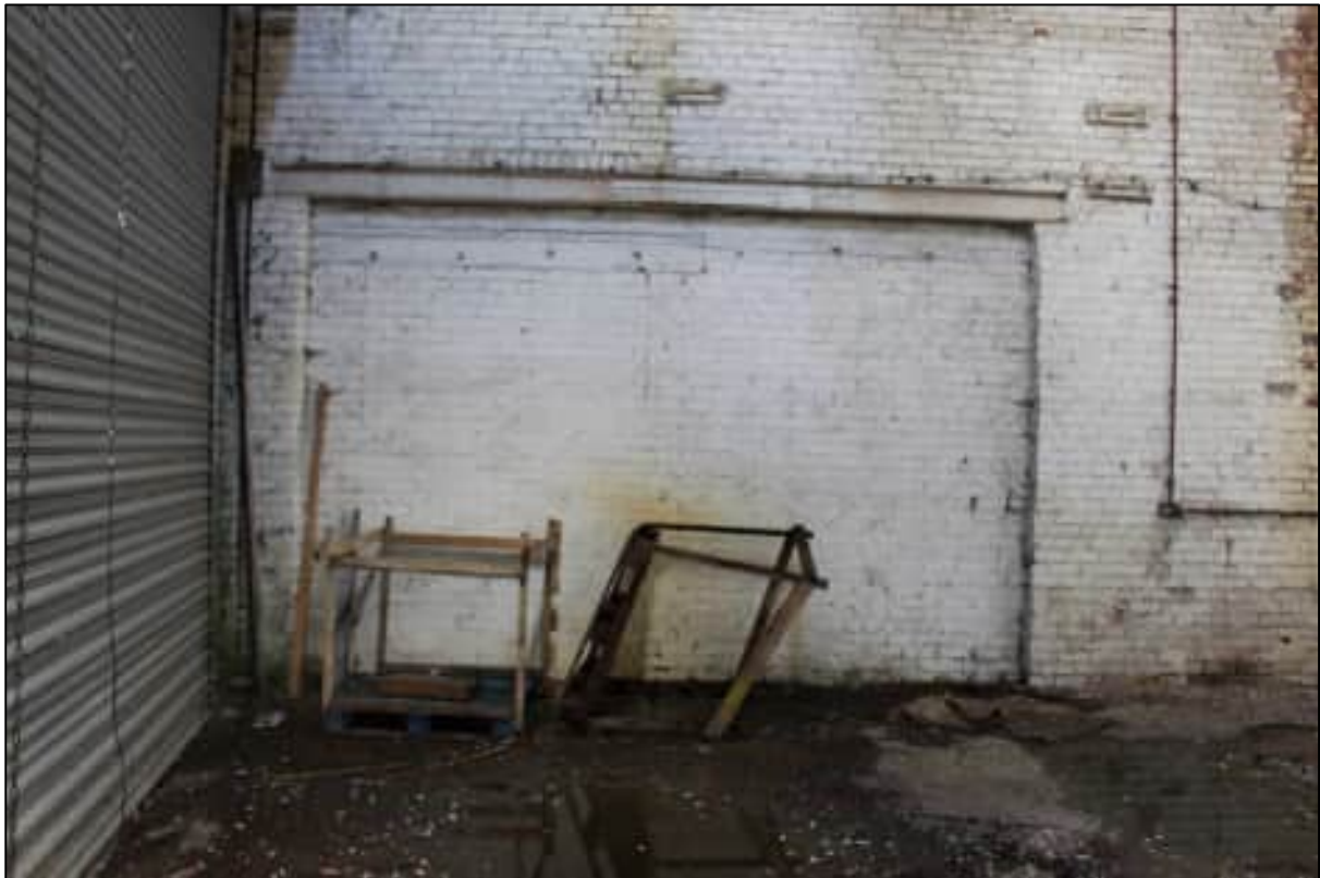
Plate 56: The blocked doorway to the eastern end of the southern wall, looking south
