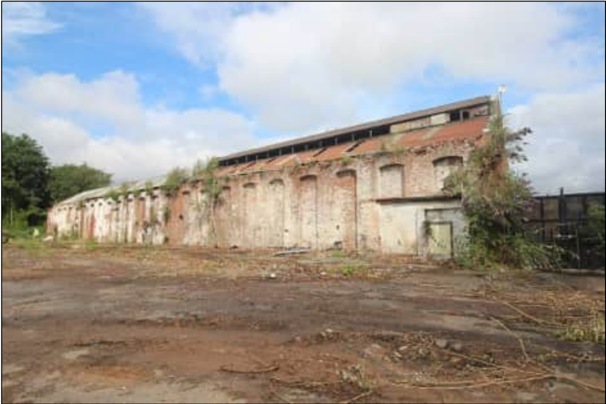
Plate 46: General view of the southern elevation of the former casting and pattern store, looking north-west
