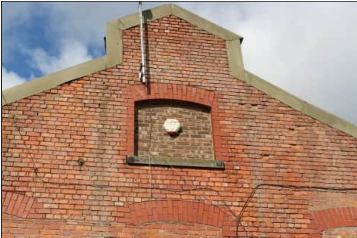
Plate 45: Detail of the blocked window and parapet wall to the lantern roof
