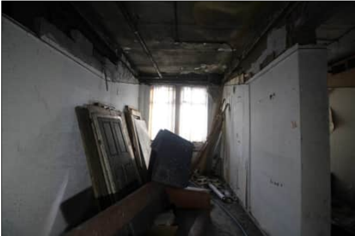
Plate 33: General view of Room 2, looking east
