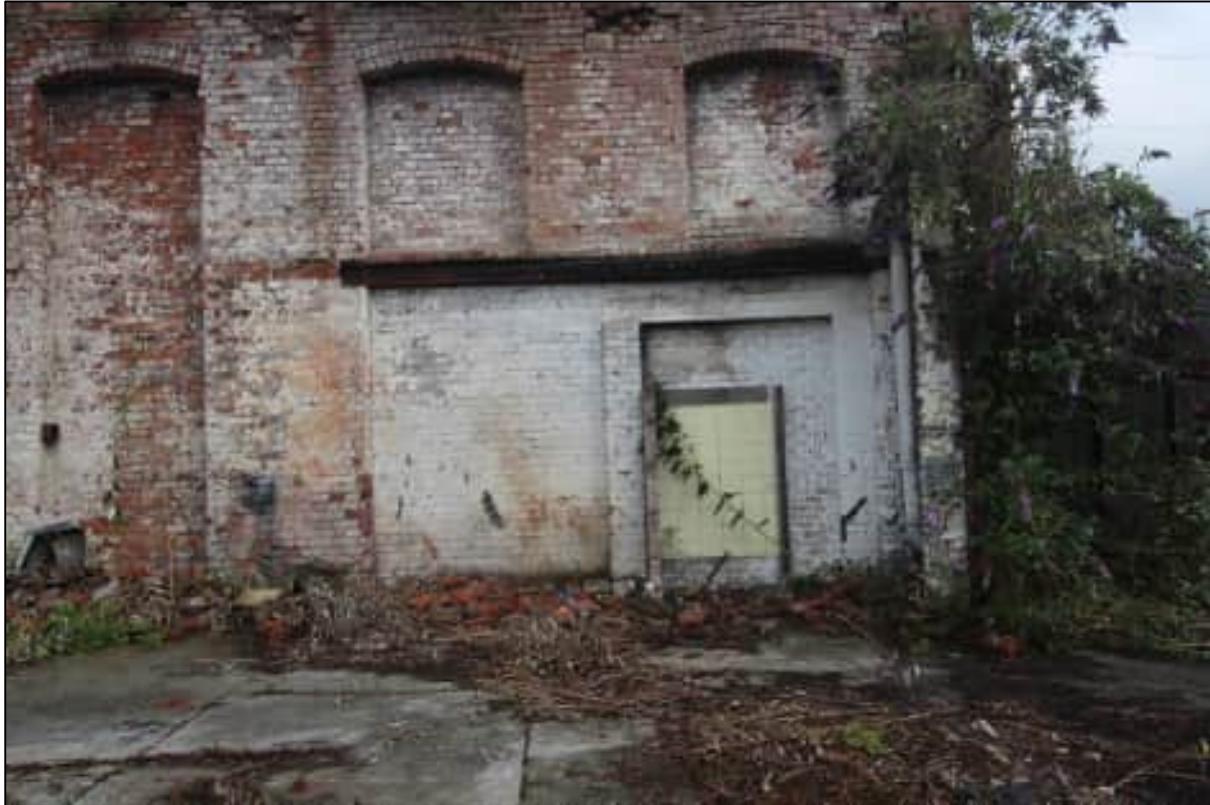
Plate 48: Detail of the remodelled doorway to the east of the southern elevation, looking north
