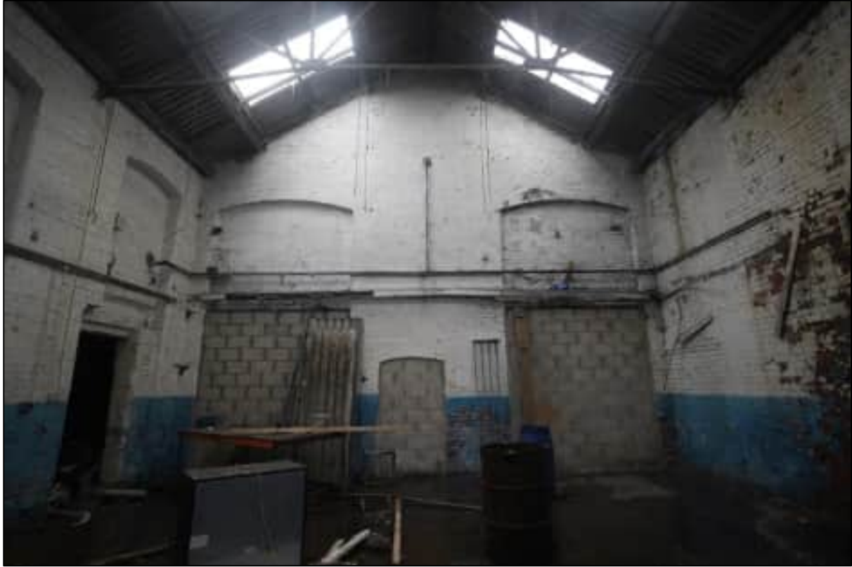
Plate 65: The eastern wall of the 1903 extension, looking east
