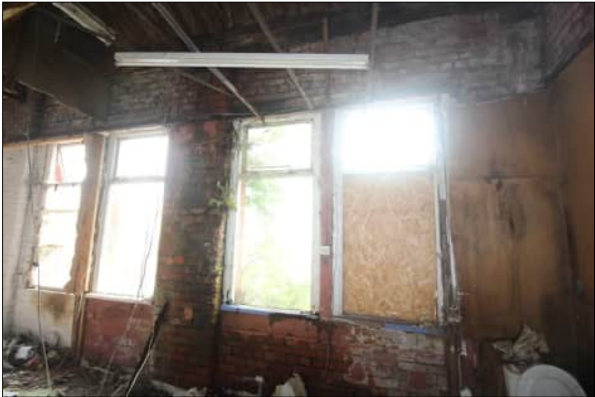
Plate 42: The windows to the eastern wall of the first floor
