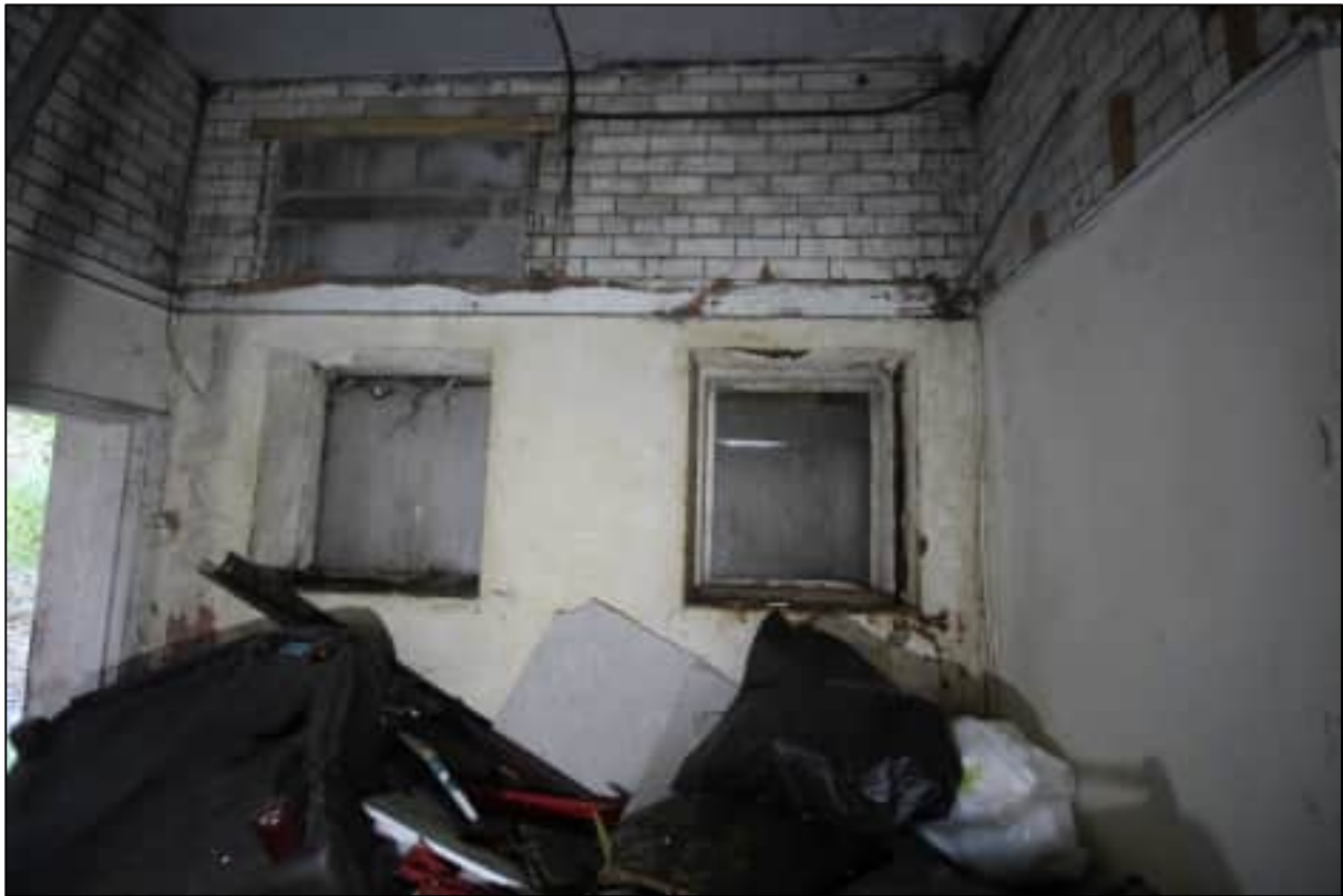
Plate 31: The western wall of Room 1, looking west
