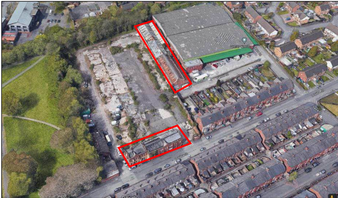
Plate 1: Recent aerial shot, showing the extant buildings to be investigated within the wider Site, looking west
