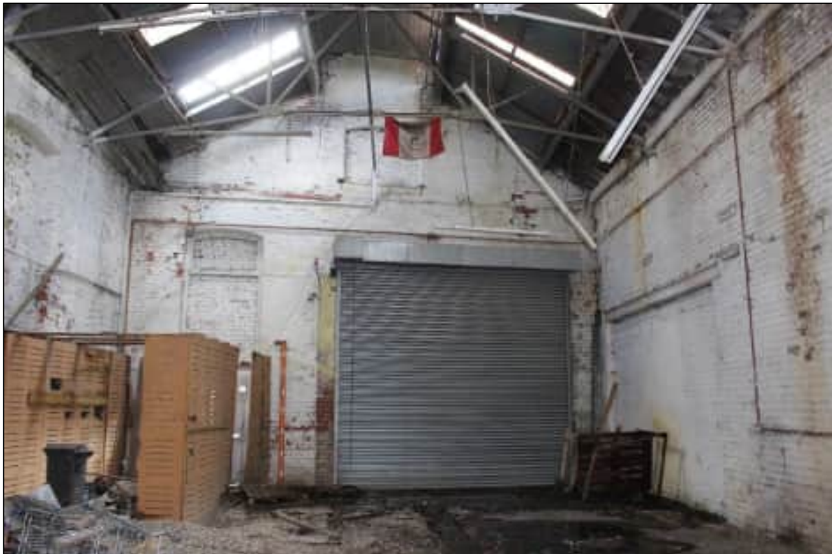
Plate 58: General view of the eastern wall of Room 1, looking east
