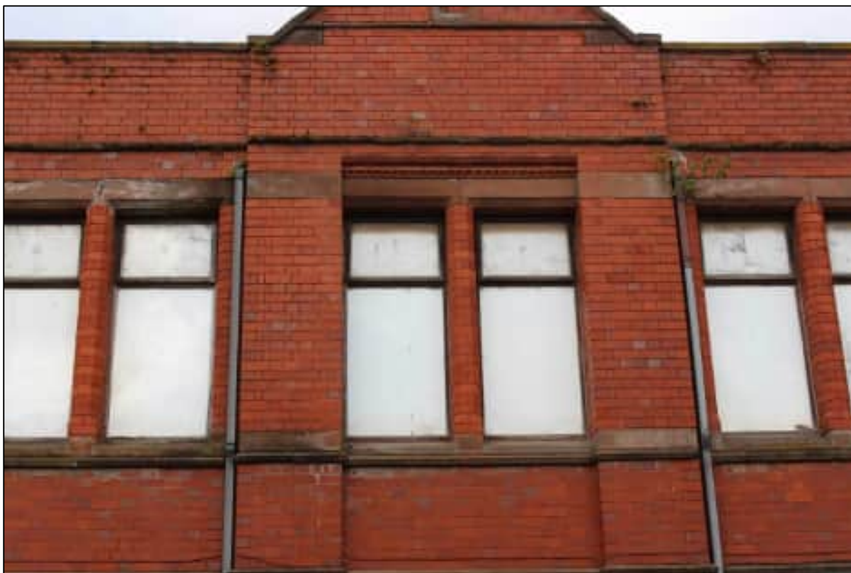
Plate 15: Detail of the first floor windows to the eastern elevation of the office extension, looking west
