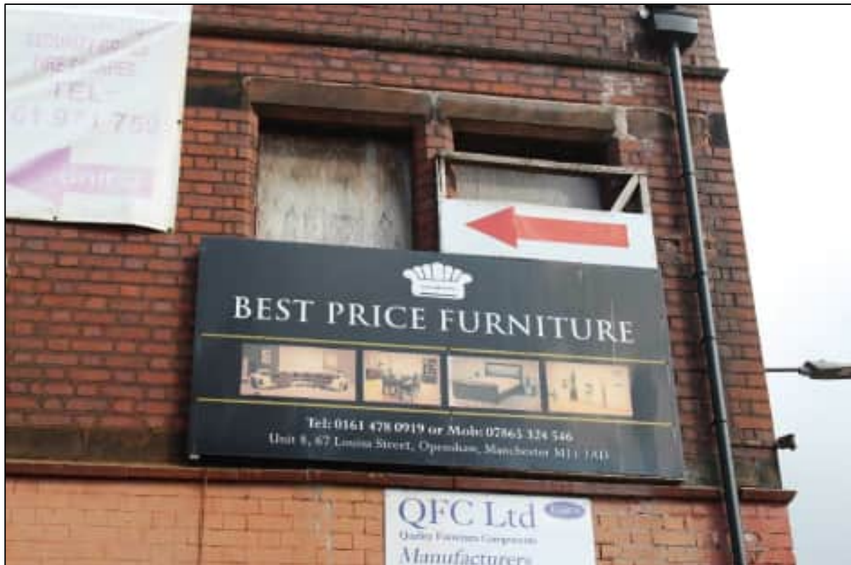
Plate 21: Detail of the blocked windows to the first floor of the elevation, looking north
