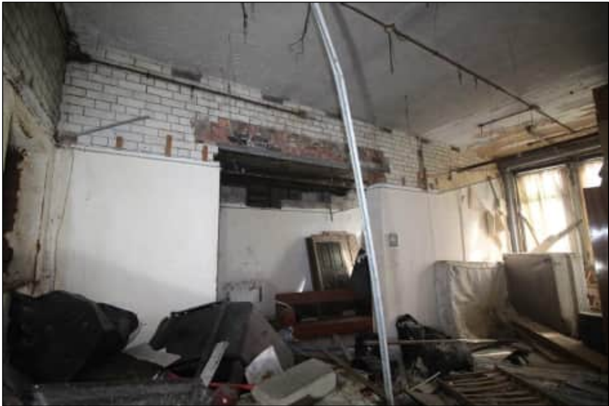
Plate 30: General view of Room 1, looking north
