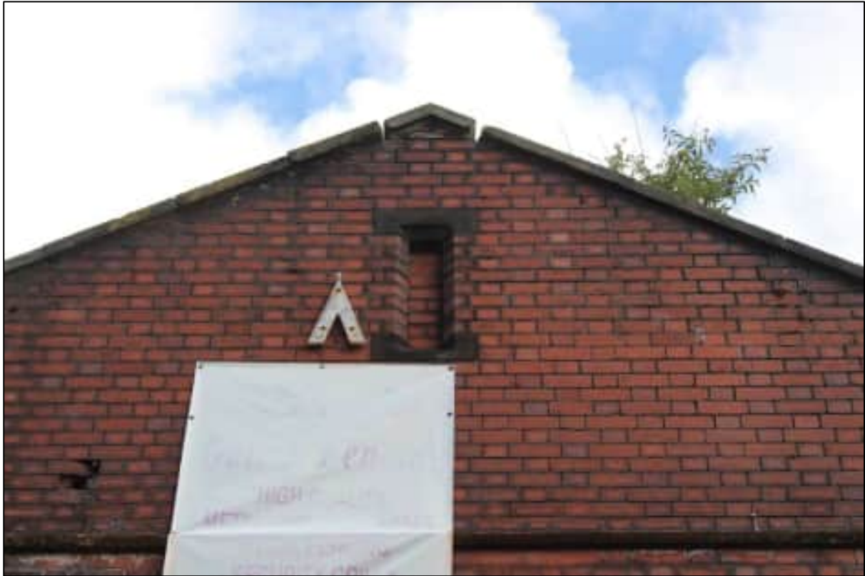
Plate 22: Detail of the blocked widow to the attic of the original 1892 office, looking north
