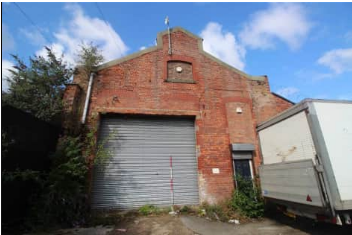
Plate 44: General view of the eastern elevation of the former casting and pattern store, looking west
