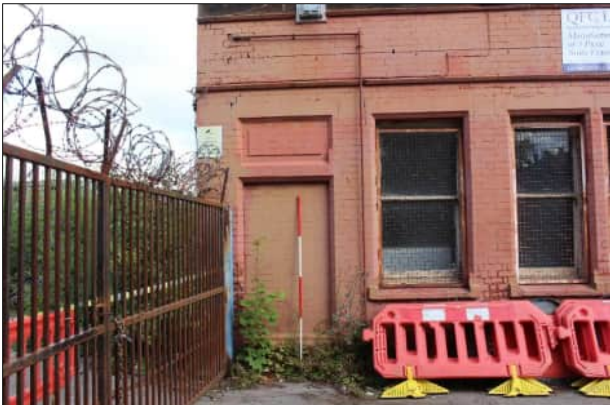
Plate 20: Detail of the blocked doorway to the western end of the southern elevation, looking north
