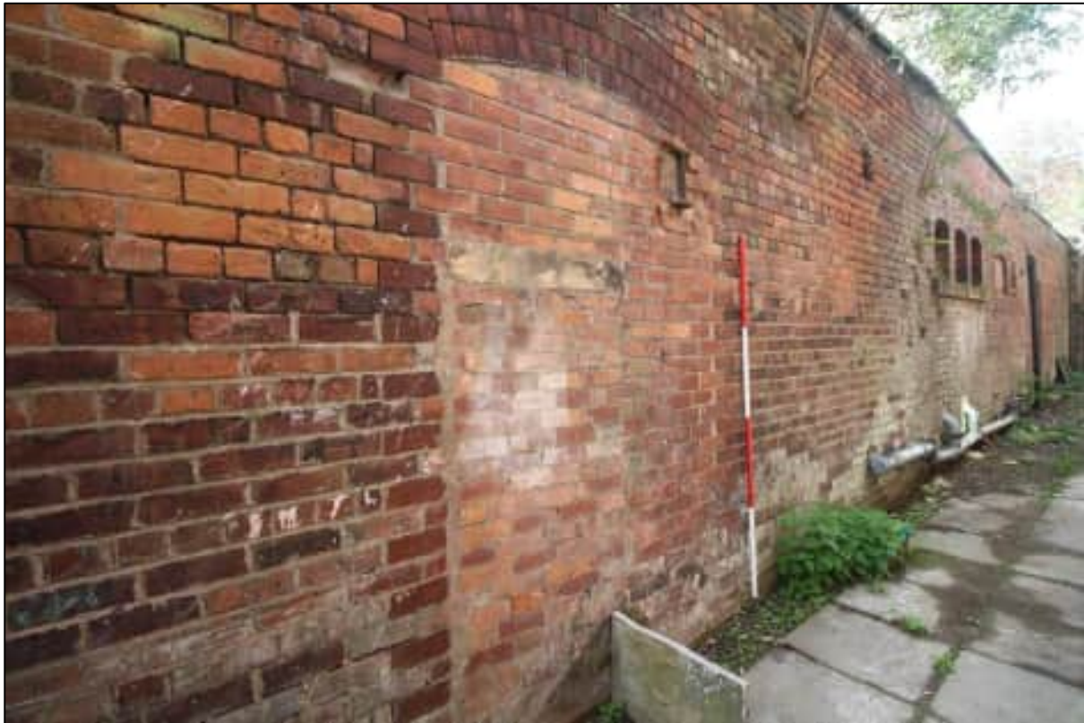
Plate 54: Detail of the blocked doorway to the northern elevation of the original workshop, looking south-west
