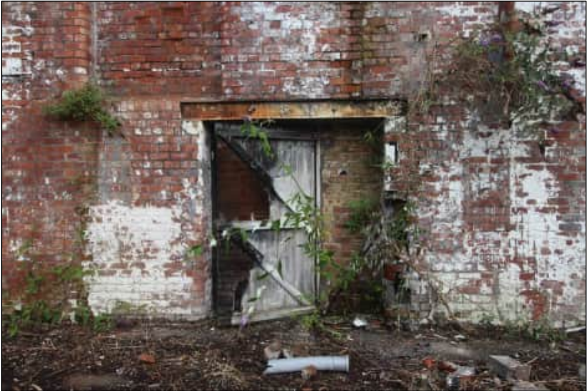
Plate 49: The westernmost doorway within the southern elevation, looking north
