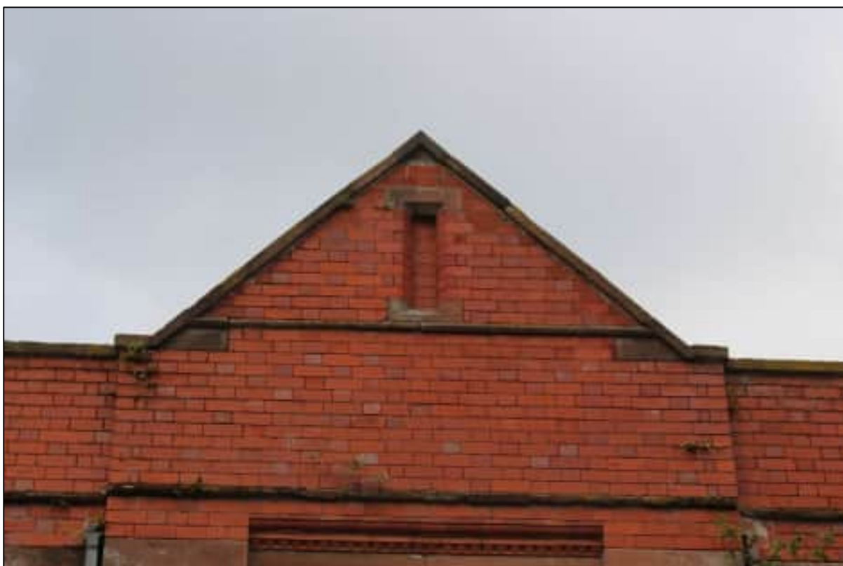
Plate 16: Detail of the gablet to the eastern elevation, looking west
