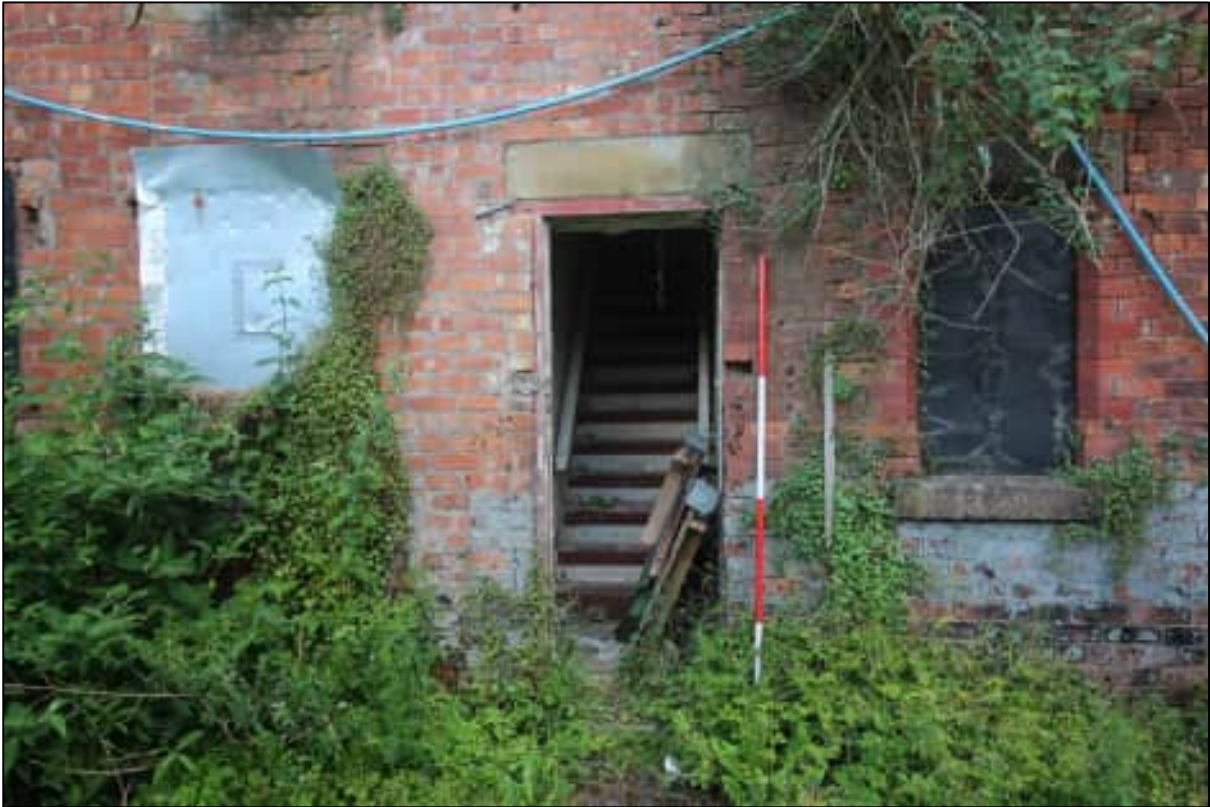
Plate 25: The doorway to the northern end of the western elevation, looking east
