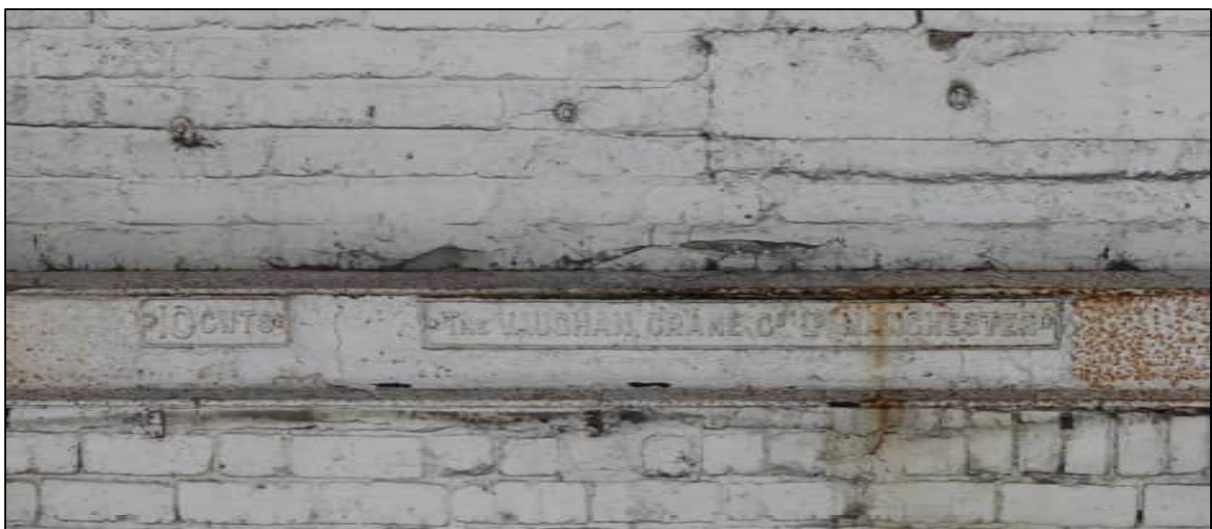
Plate 57: Detail of the rivetted makers sign to the web of the steel lintel
