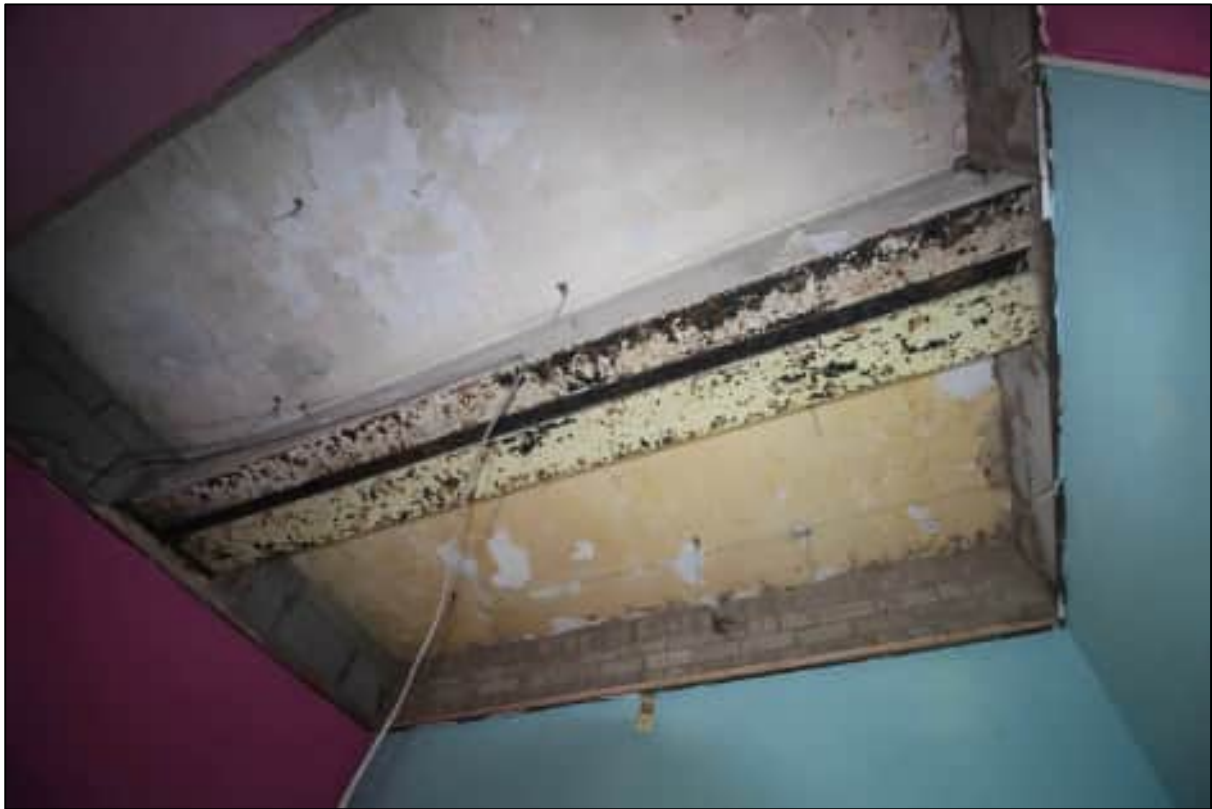
Plate 37: The rolled iron beam within ceiling of Room 9
