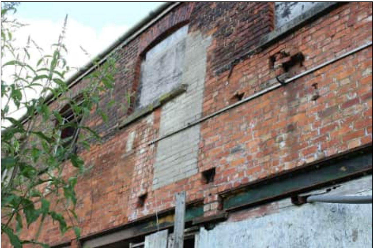
Plate 28: Detail of the blocked loading bay on the first floor of the western elevation
