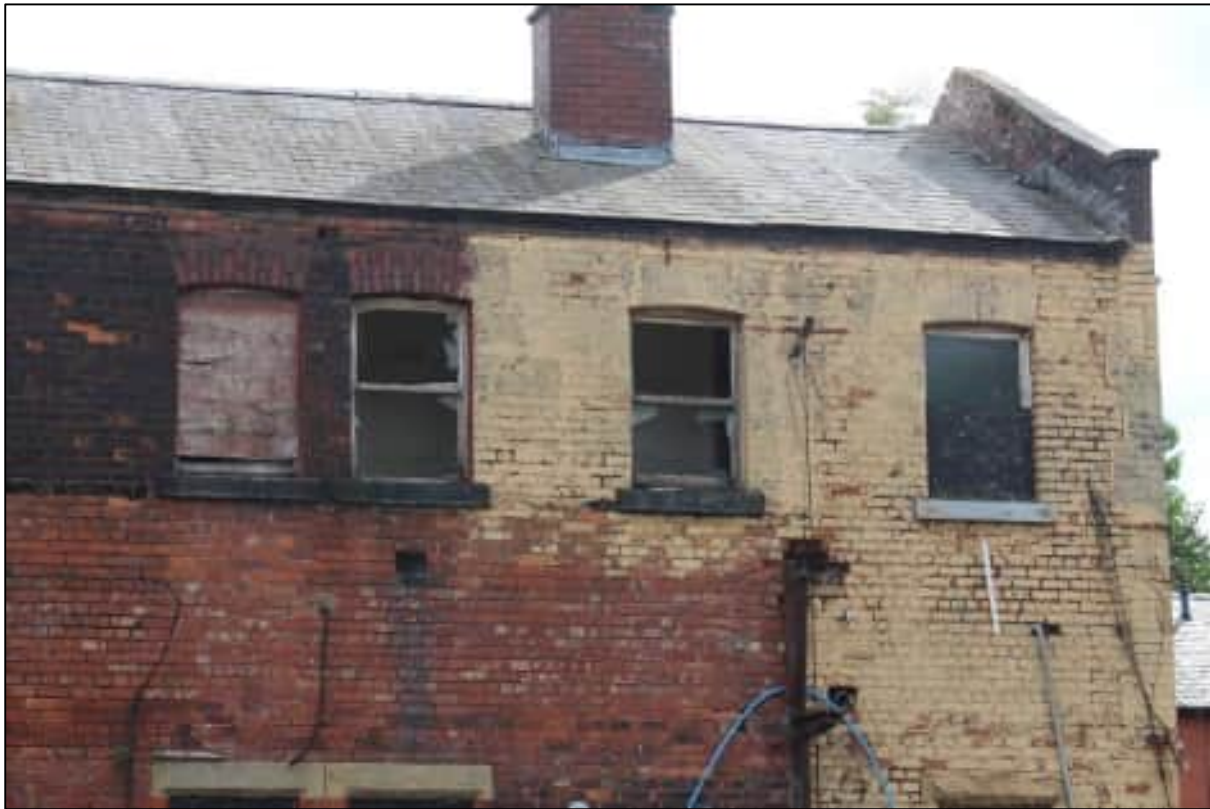
Plate 26: The first floor windows on the western elevation of the 1892 office building, looking east
