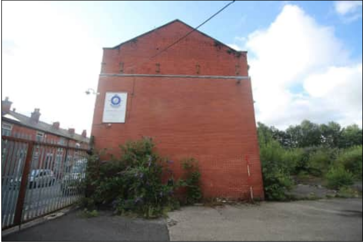
Plate 17: The northern elevation of the 20 th -century office extension, looking south
