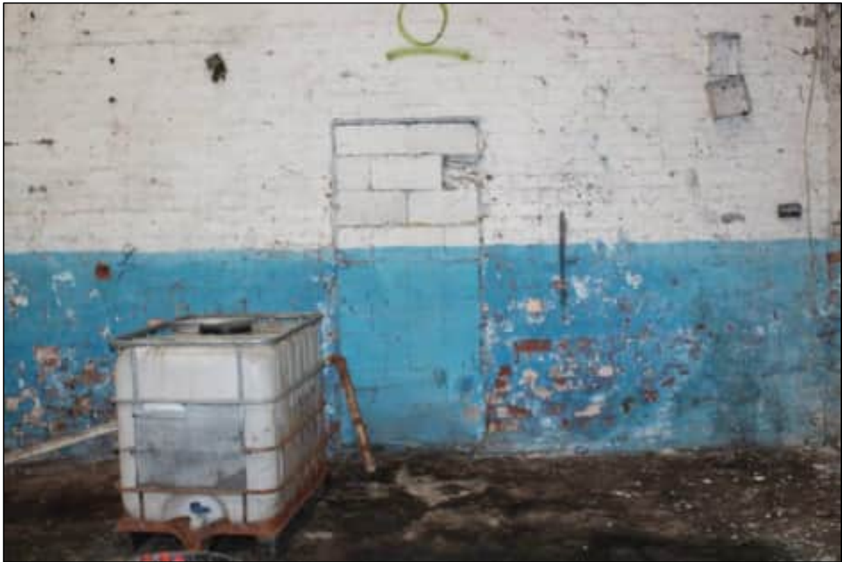
Plate 66: The blocked doorway within the southern wall, looking south
