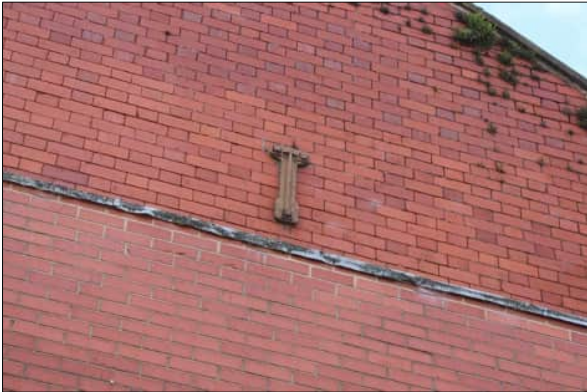
Plate 18: Detail of tie rod plates to the northern elevation
