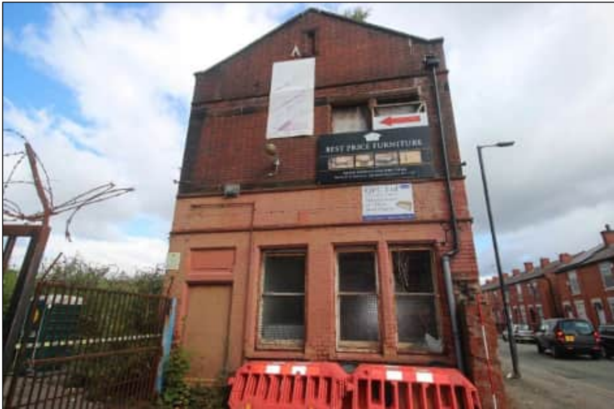
Plate 19: The southern elevation of the 1892 office building, looking north
