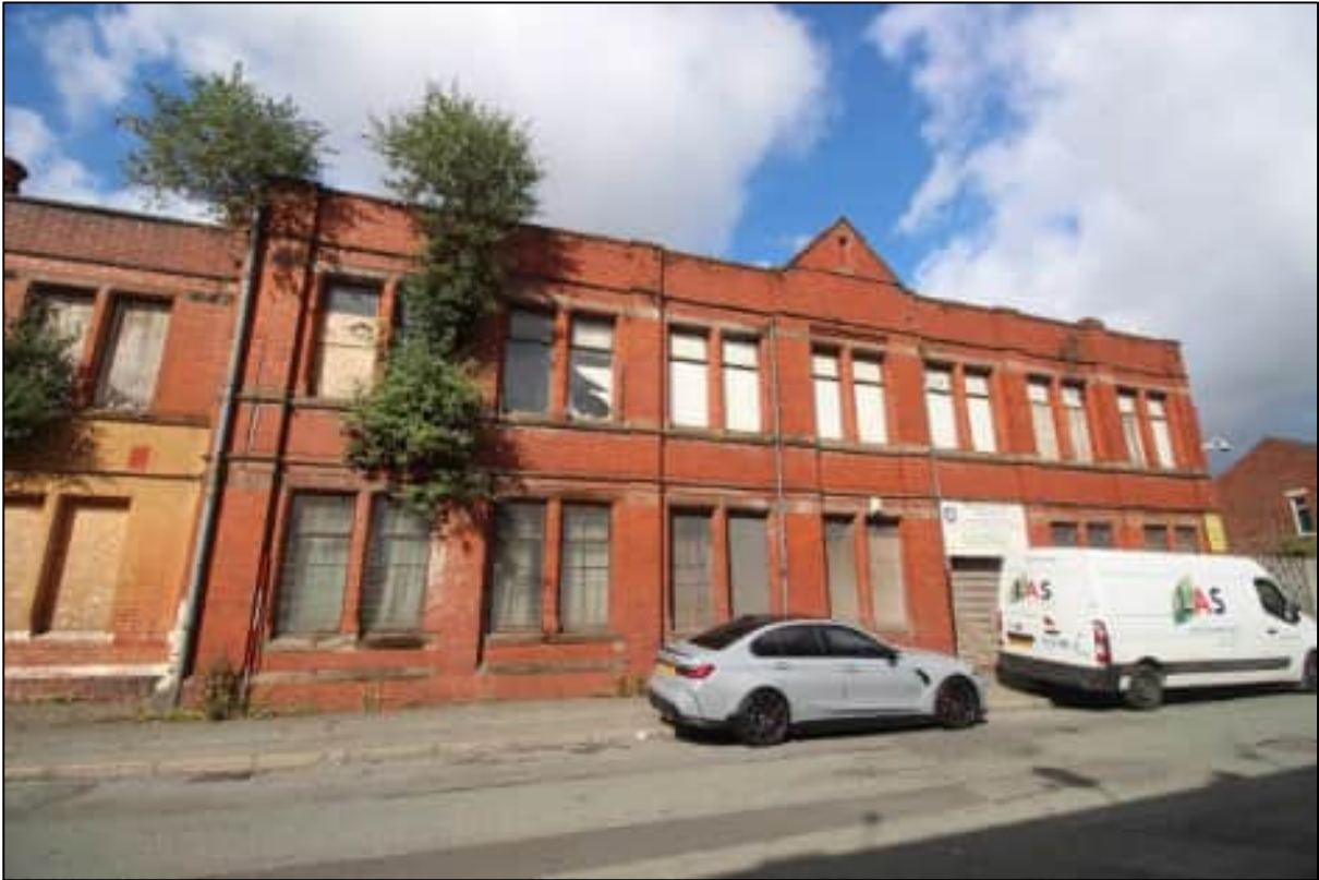
Plate 12: General view of the 20 th -century extension to the office building fronting Louisa Street, looking west
