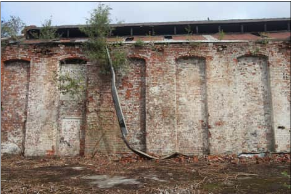
Plate 47: Detail of the blind bays forming the southern elevation, looking north
