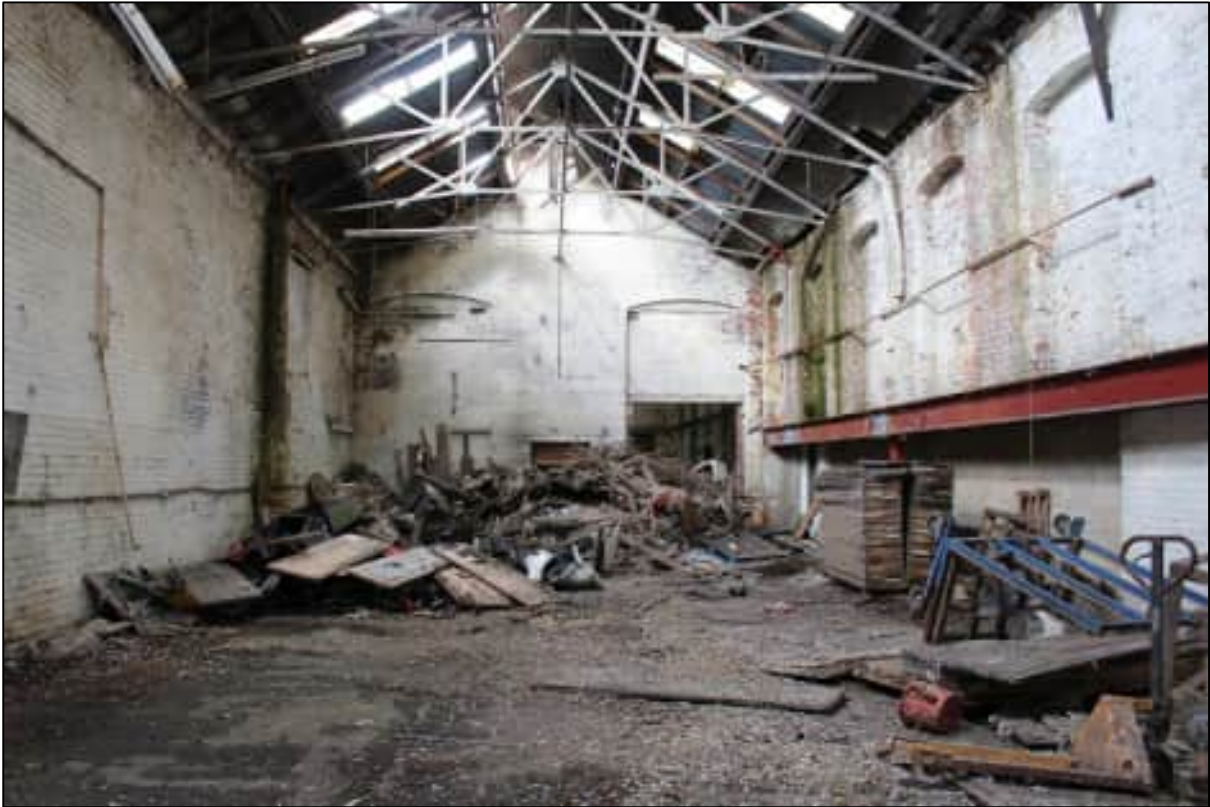
Plate 55: General view of Room 1 within the original casting and pattern store workshop, looking west
