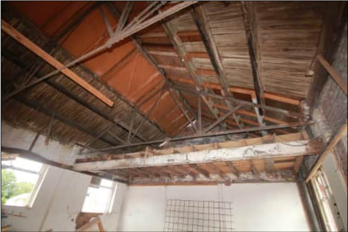
Plate 41: Detail of the original ceiling to the first floor of the extension
