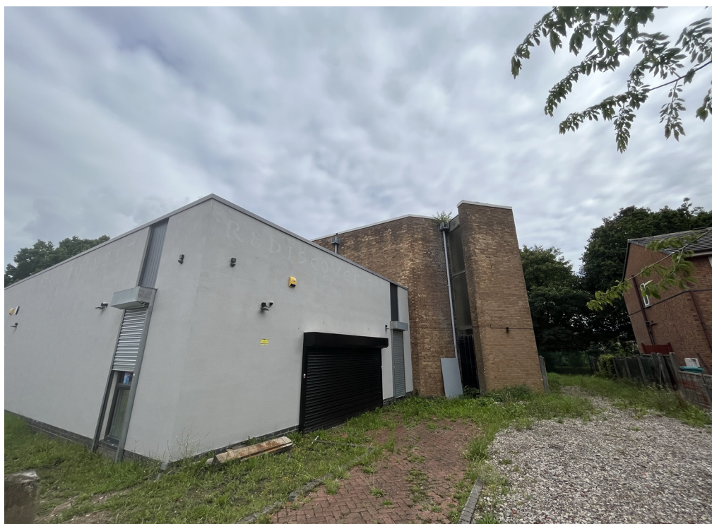
Figure 2. View from Chalford Road.
