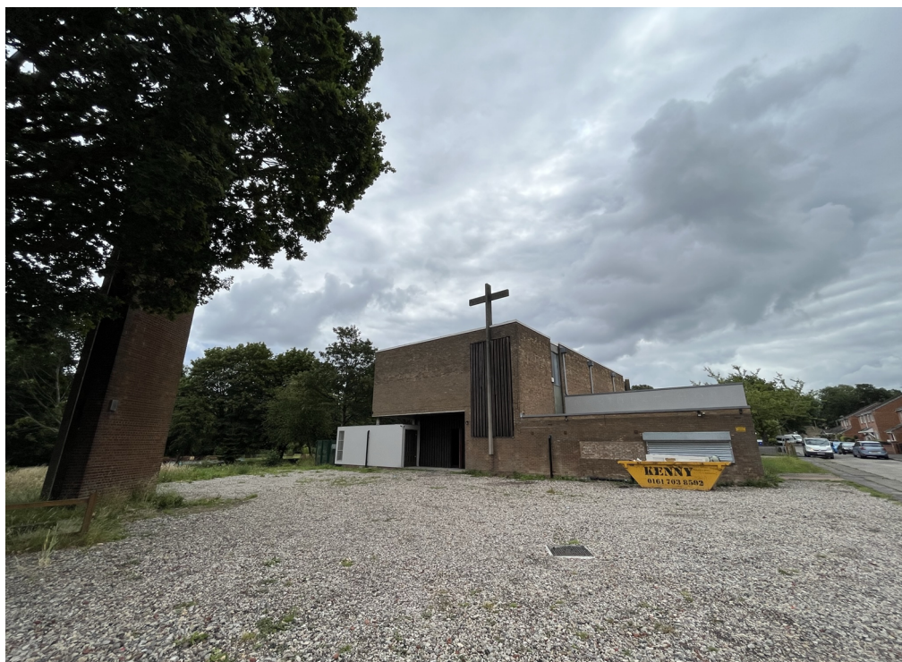
Figure 1. View from Greenbrow Road
