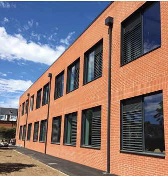
E. Anticlimb Rain Water Pipes
