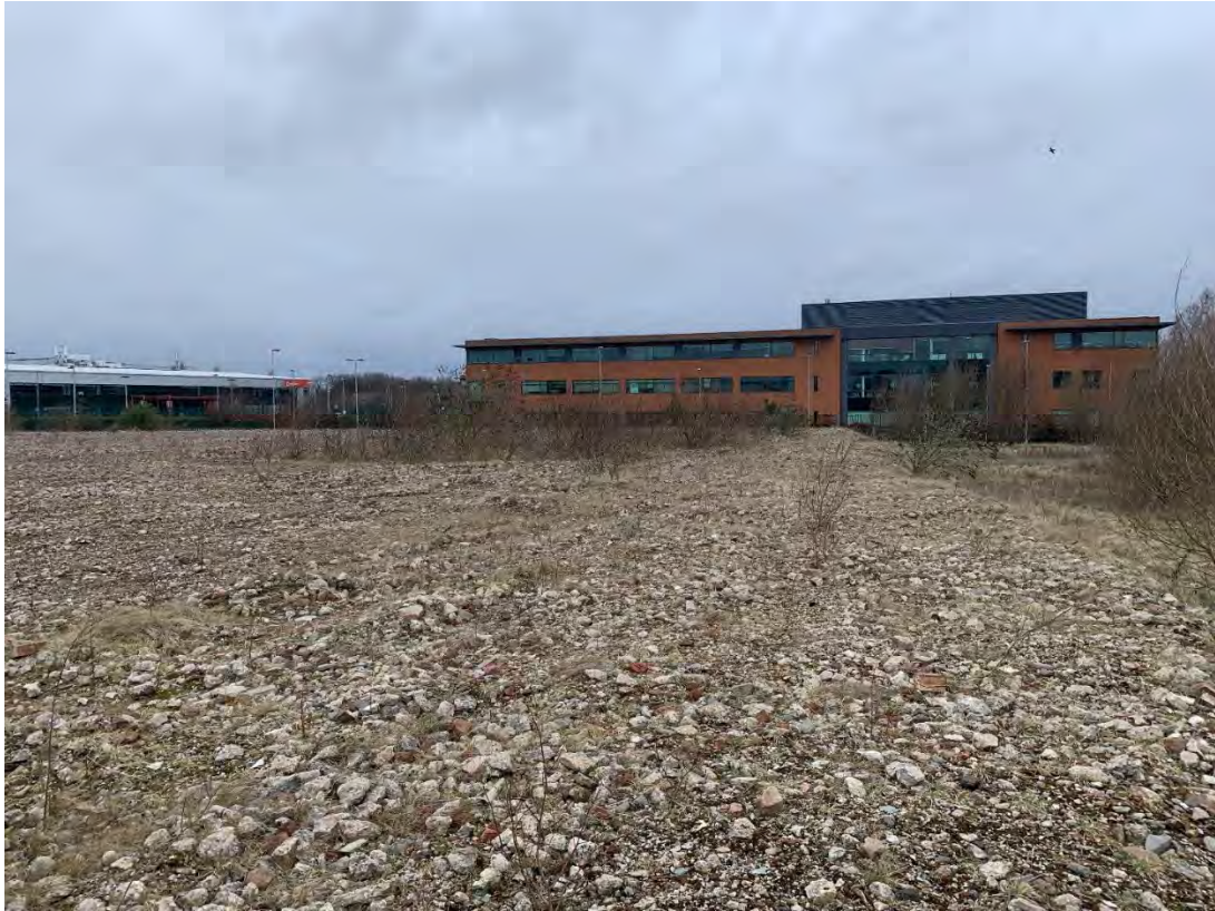
Photograph 11 - Demolition rubble in the western extent of the Site
