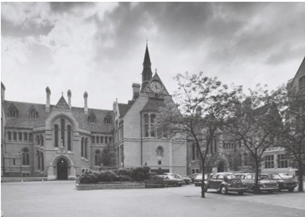
Figure 5.14: Undated, c 1965 showing raised bed and car parking.
