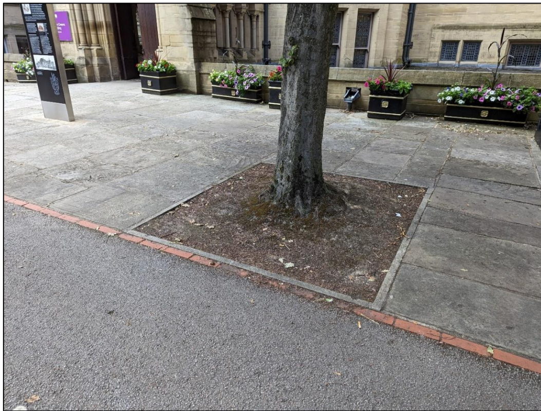
Figure 7.3: Terracotta detailing to flags and tarmac.
