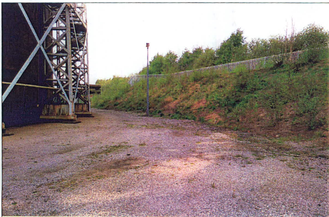
Plate 2: View looking south-west, embankment within gasholder compound on western boundary.
