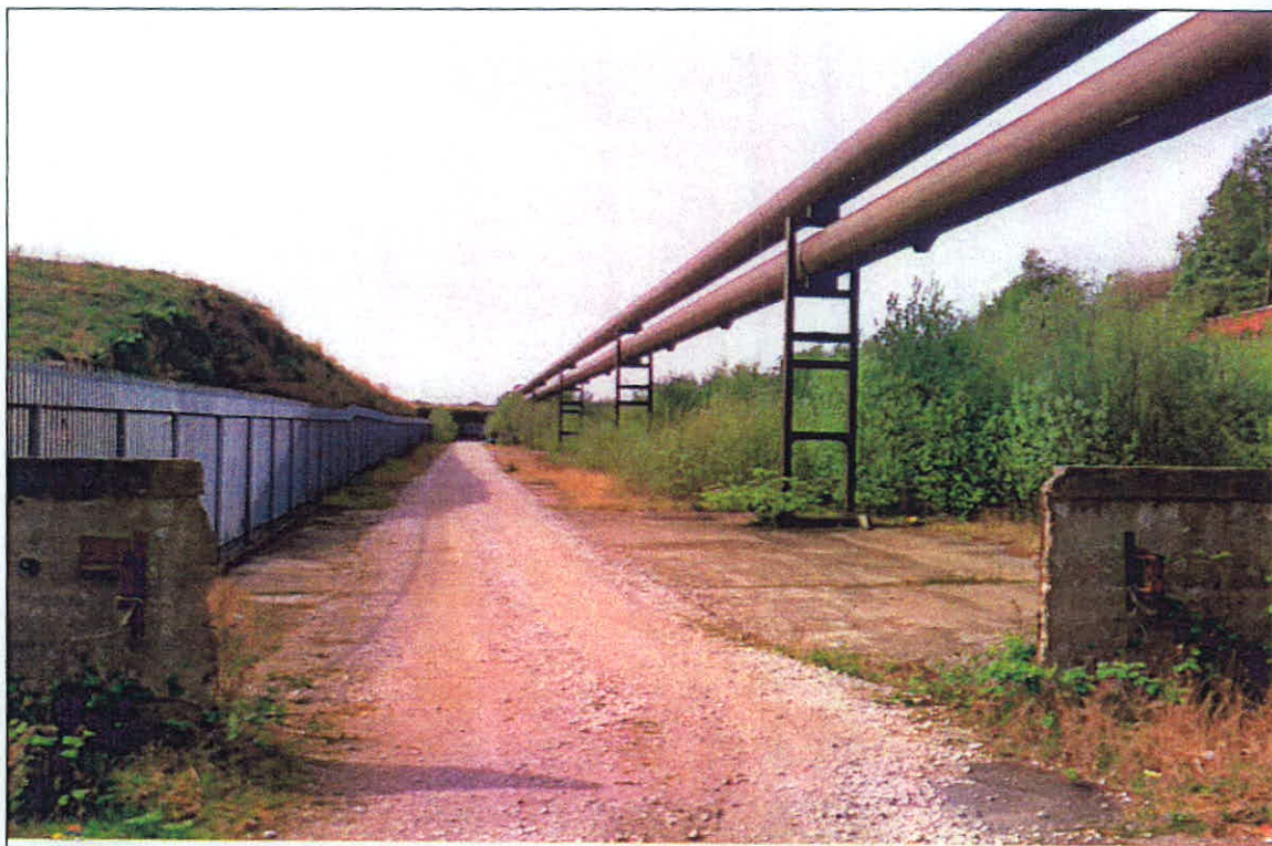
Plate 5: View looking south-west showing raised car parking in area of former gasworks and above ground gas mains.
