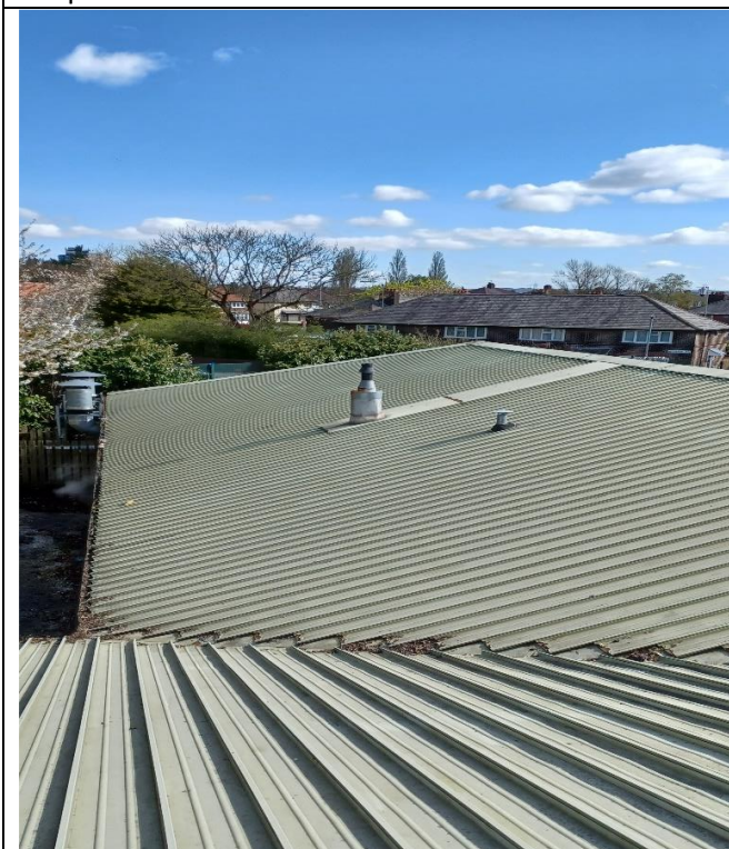
Roof, Rear Elevation
