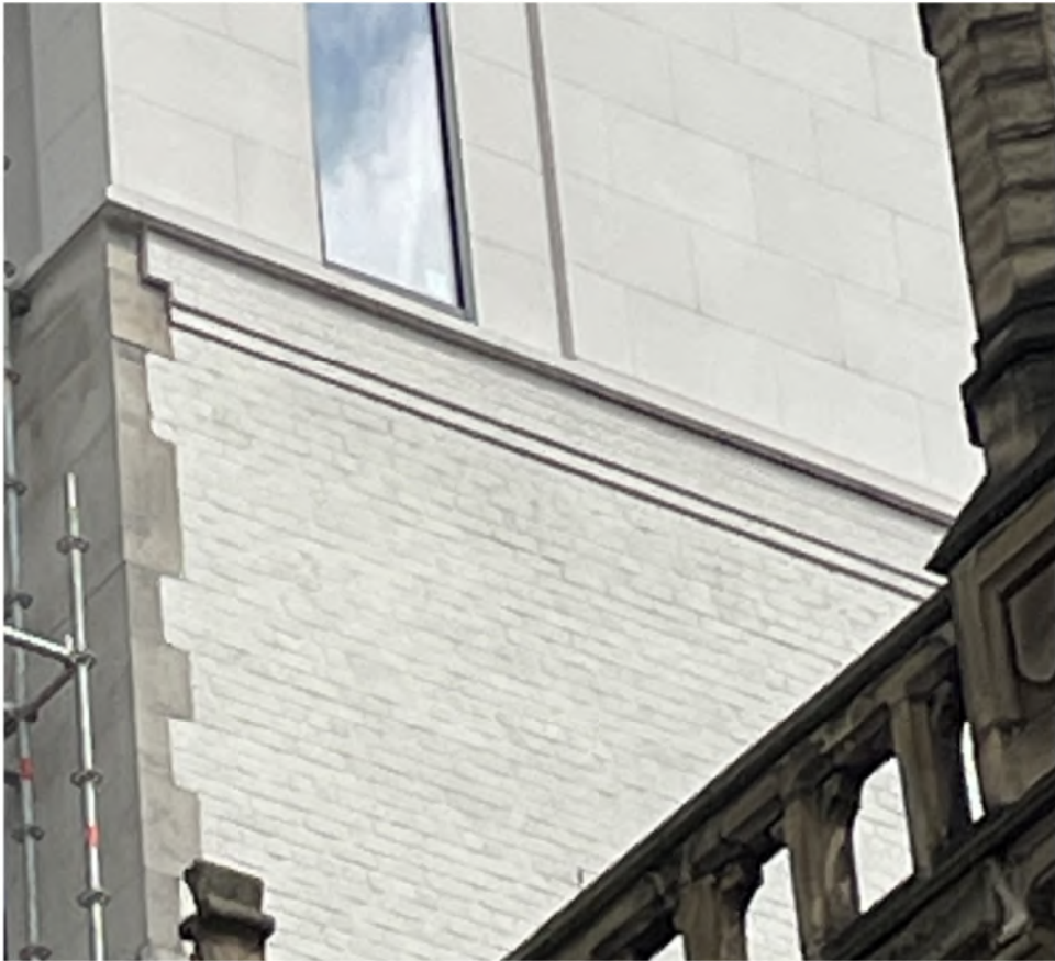
Item 4 New brickwork/masonry paint
