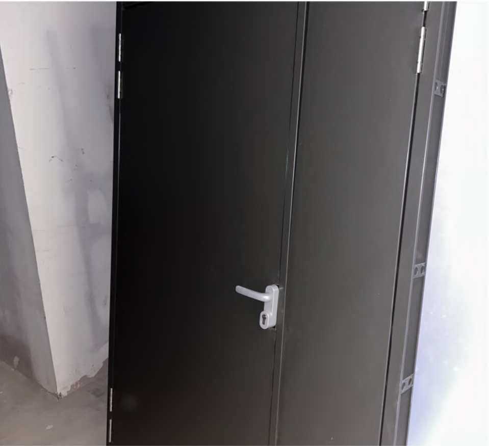
Item 6 New external doors
