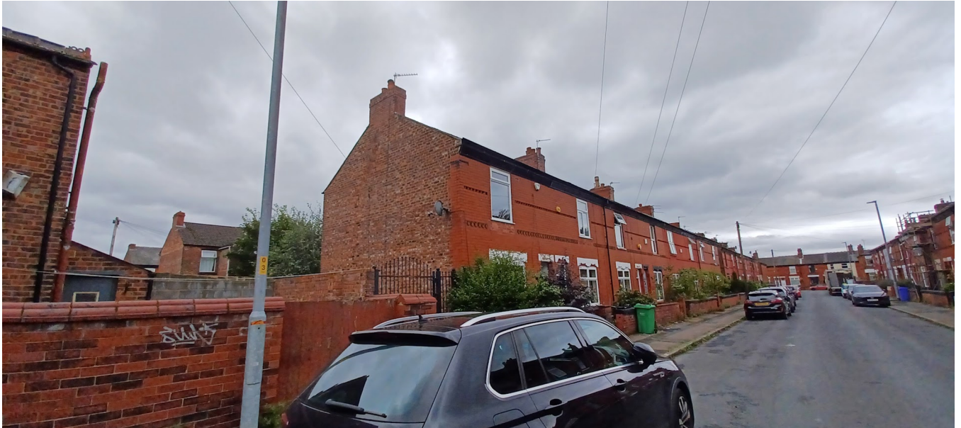
Figure 2. View of gable end from street.
