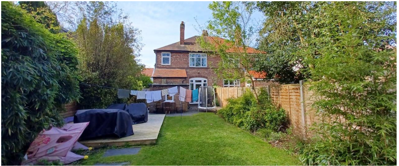
Figure 2. Rear view of property.
