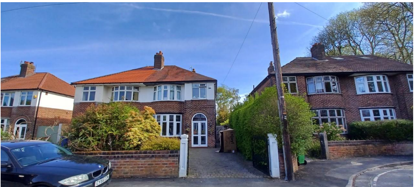
Figure 1. Principal elevation of No.23 Ferndene Road.
