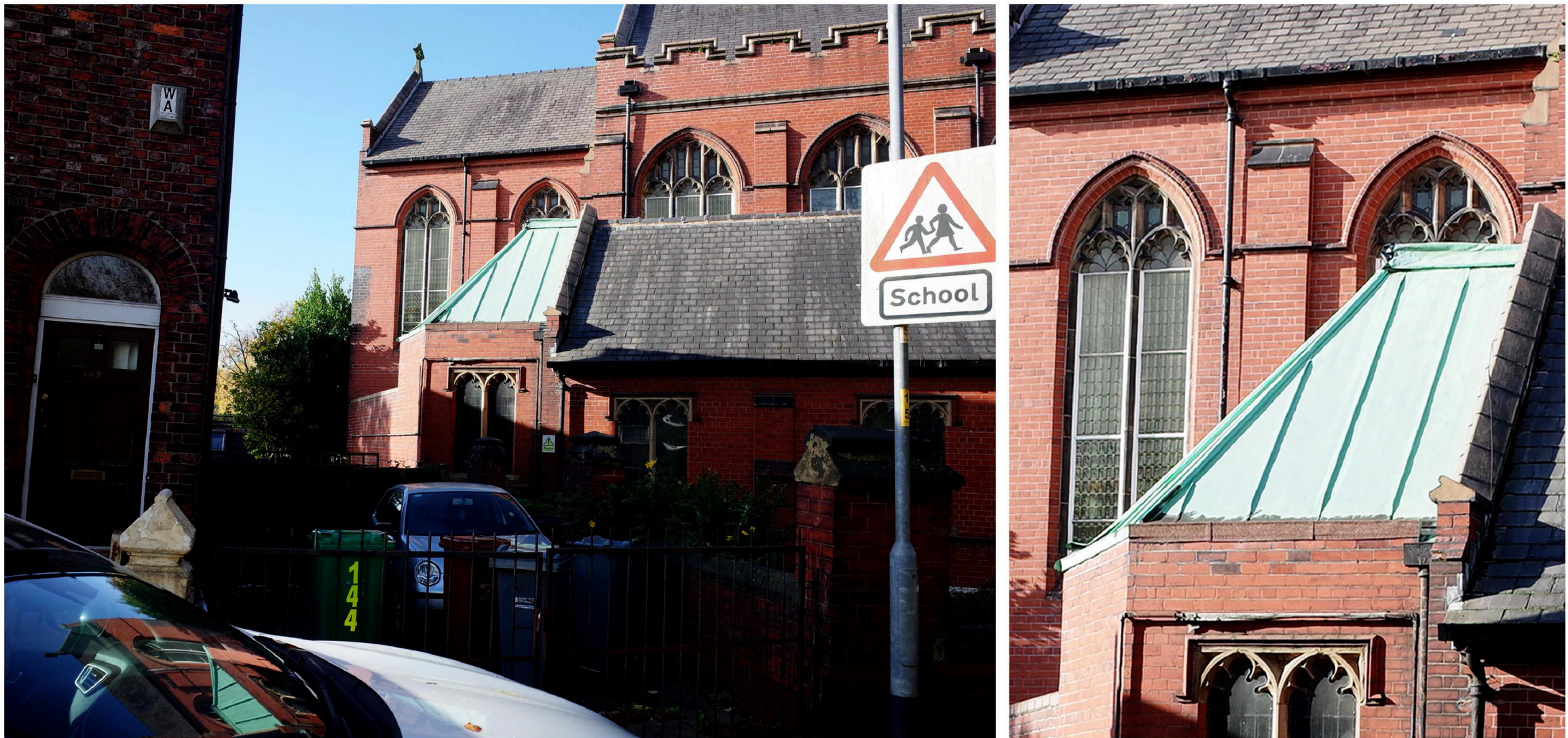
Existing Copper Apsidal Roof to Lady Chapel
