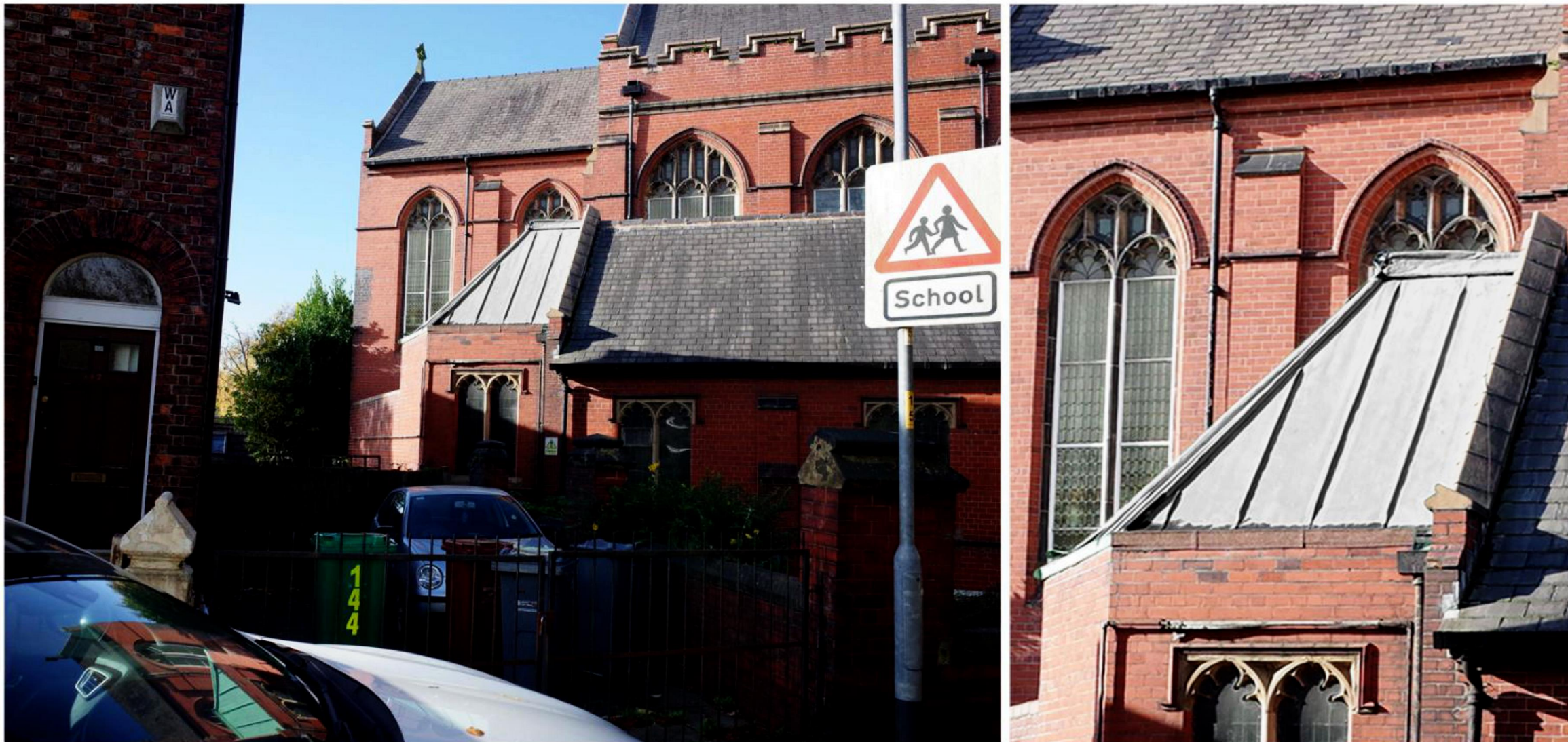
Proposed Terne Coated Stainless Steel Apsidal Roof to Lady Chapel
