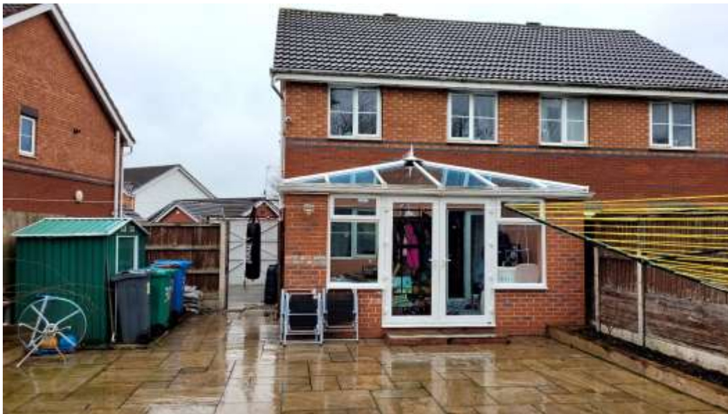
Above: Rear Elevation facing the property
