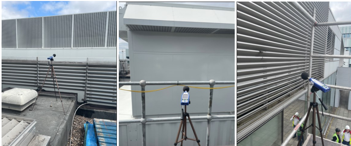
Figure 4 Photographs of generator measurement positions 1 (left), 2 (centre) and 3 (right)
