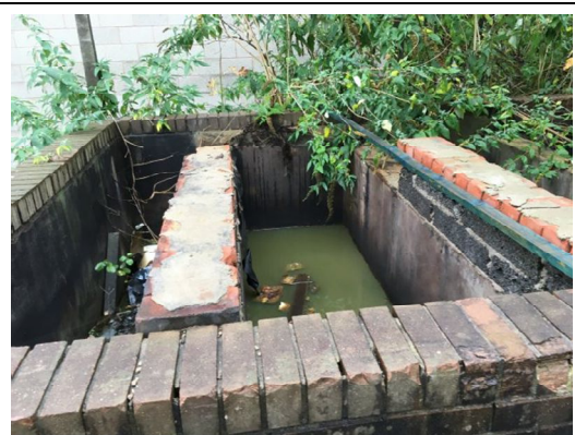
Photograph 6: Brick structure in the west of the site (possible tank storage area).
