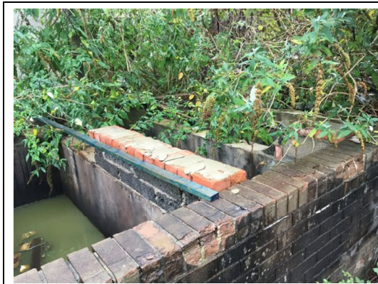
Photograph 5: Brick structure in the west of the site (possible tank storage area).
