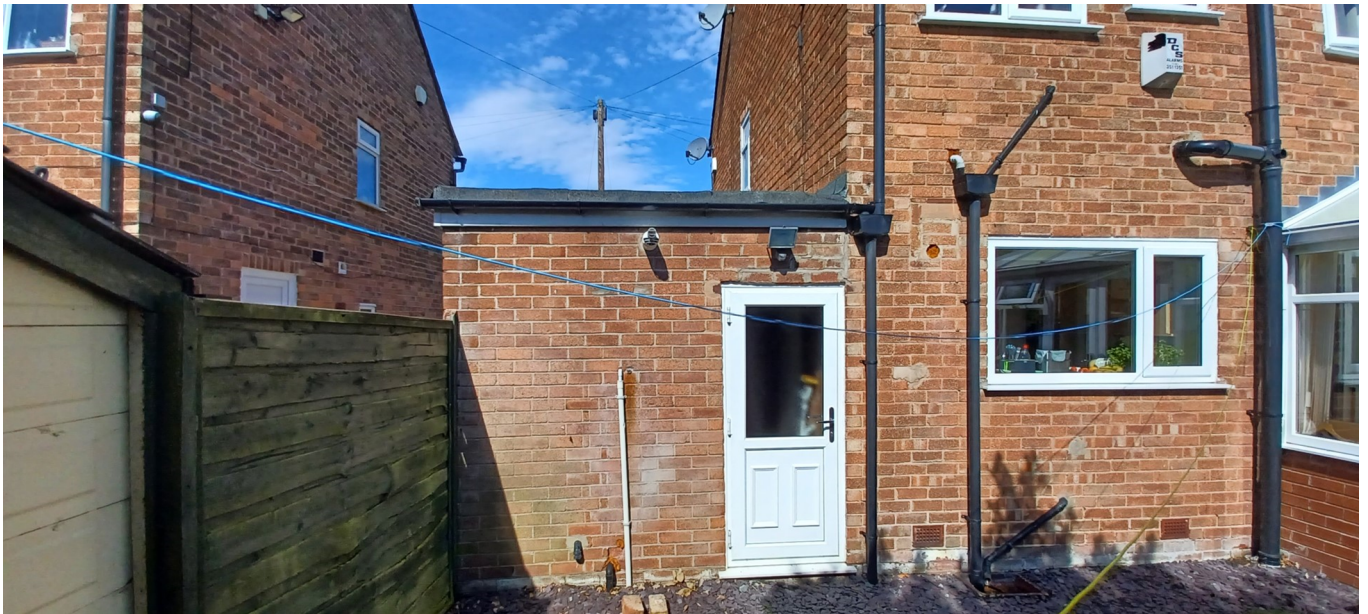
Figure 2. Existing attached garage.
