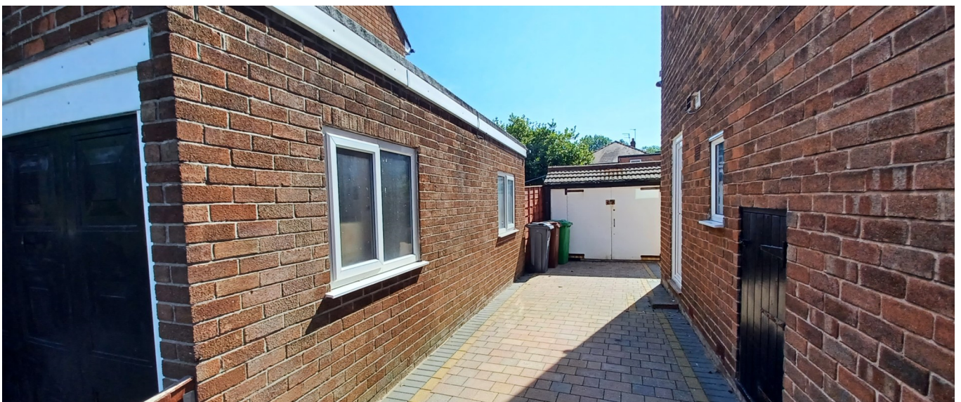
Figure 4. Existing windows along the side elevation of garage.
