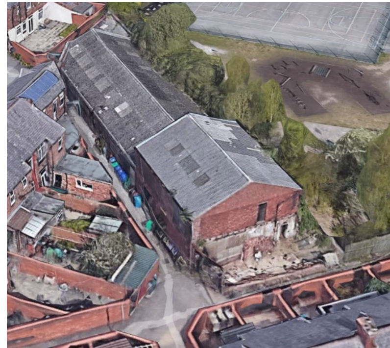
Existing single storey warehouse to north, with two storey structure to rear. The wall enclosing the yard at the end of the site has now become dilapidated. The line of the fence erected on Diocese land can be seen to the right. (Image source— Google Earth)
