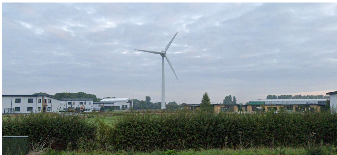
Green Park Business / Industrial Park, Newport
