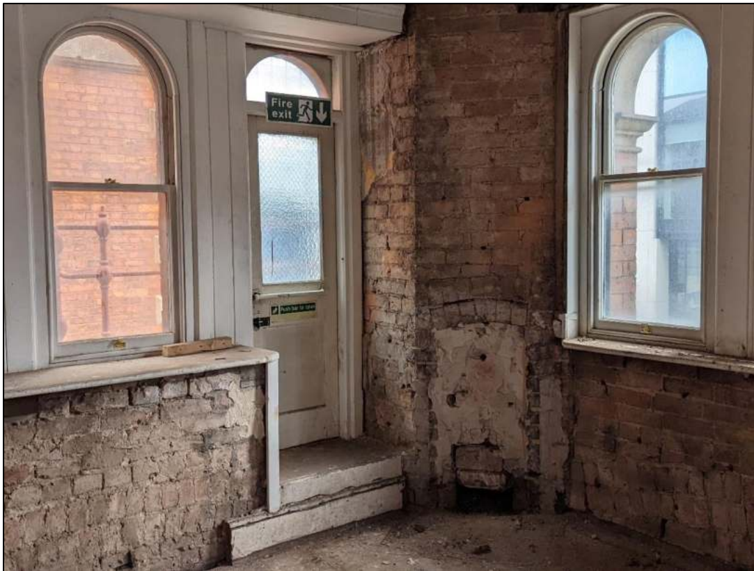
Plate 95: Inserted fire escape with blocked corner fireplace
