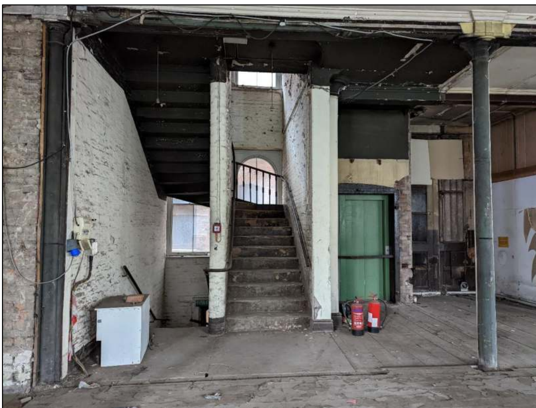
Plate 64: Staircase to second floor
