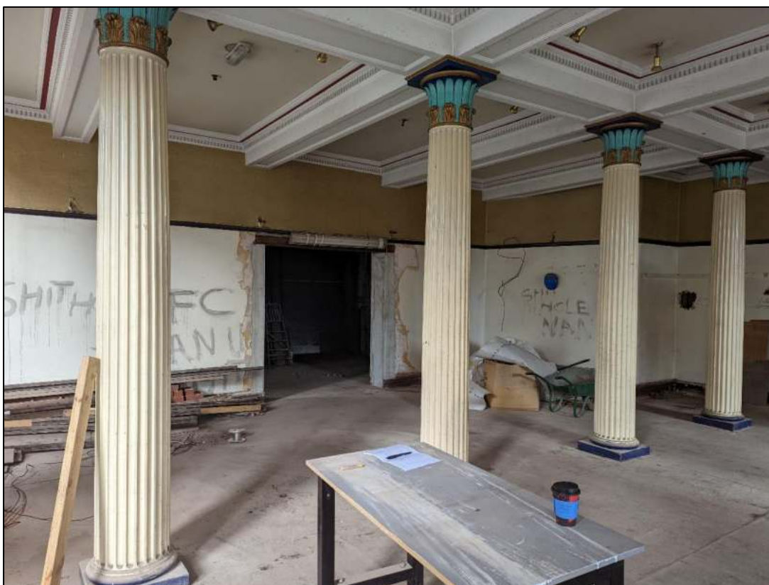
Plate 34: Inserted opening to south
