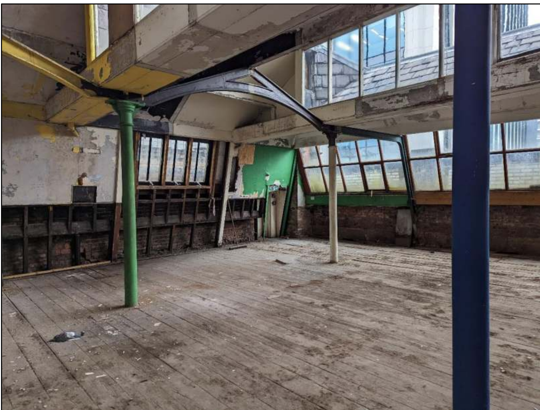
Plate 104: Northwest corner showing inserted fire escape
