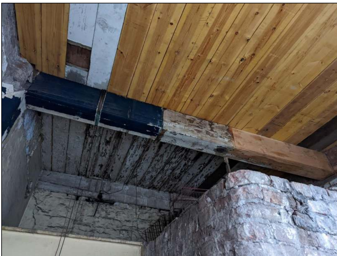
Plate 68: Ceiling showing original and modern timber boards
