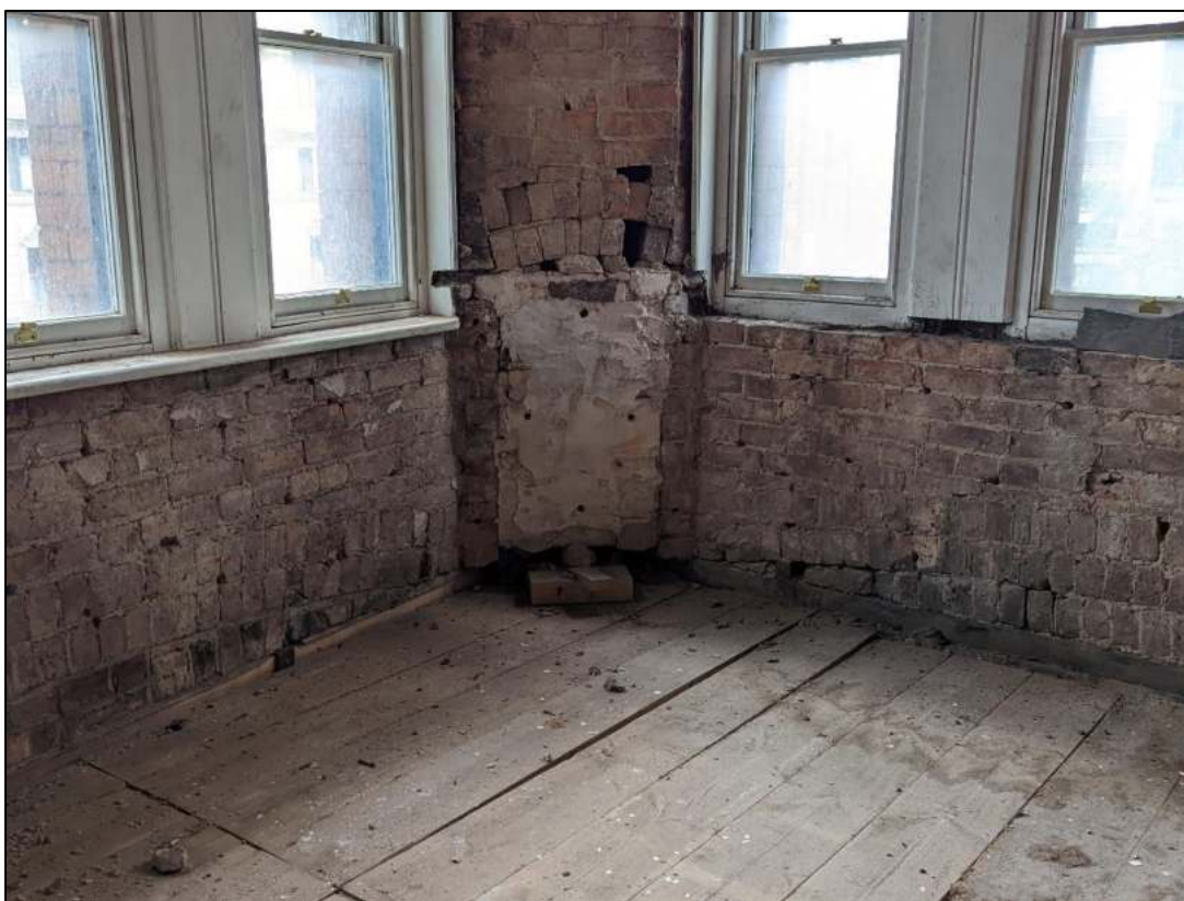
Plate 96: Blocked corner fireplace to northeast
