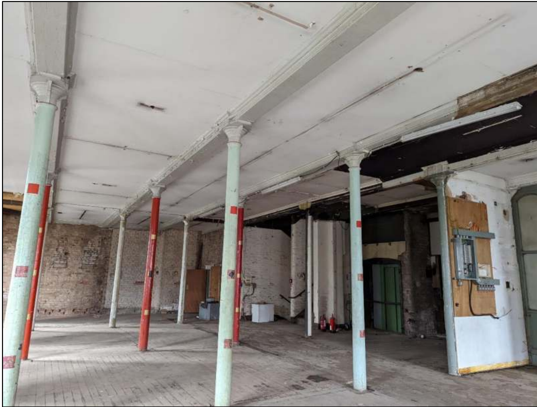
Plate 71: Lath and plaster ceiling
