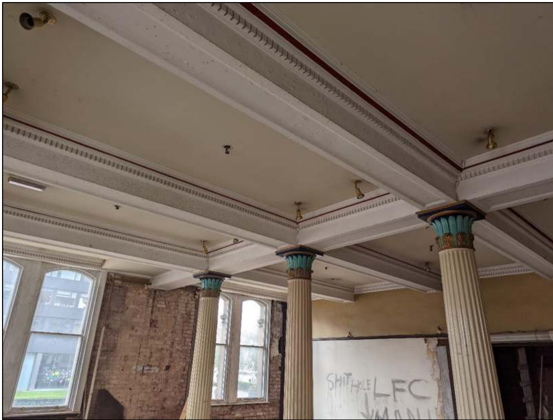
Plate 27: Stanchion capitals and ceiling
