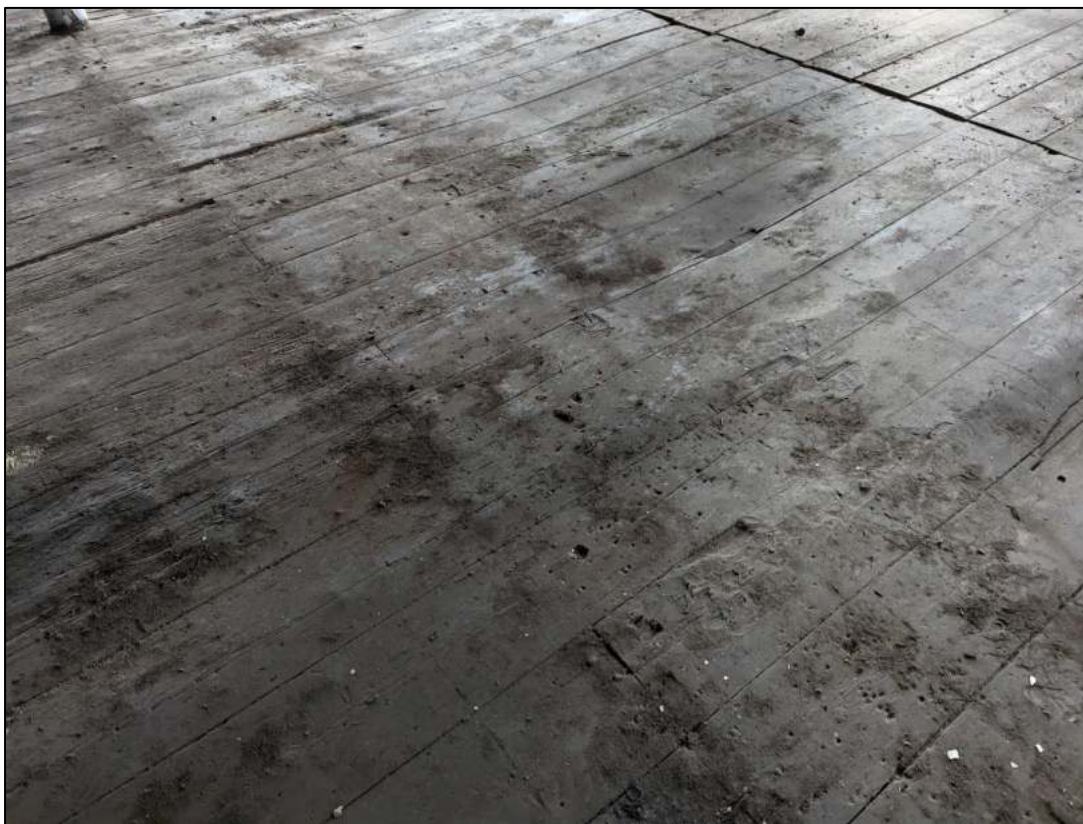
Plate 88: Original timber boards
