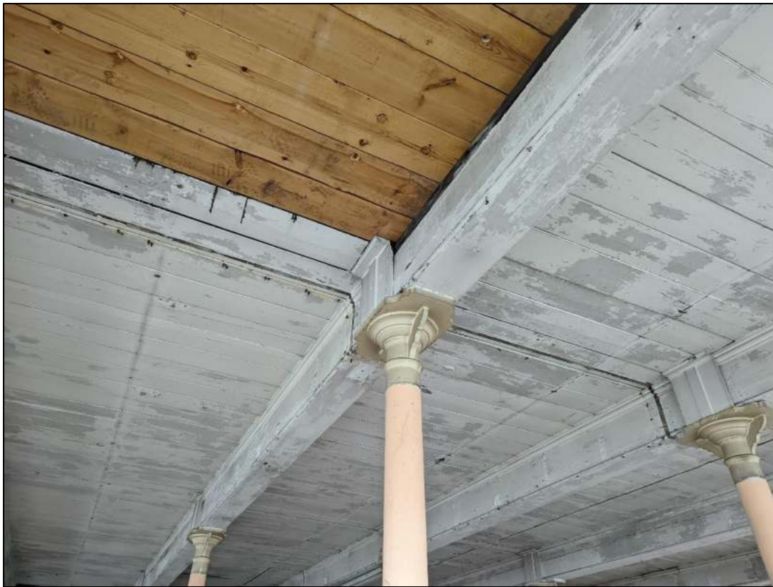
Plate 79: Ceiling showing original and modern timber boards
