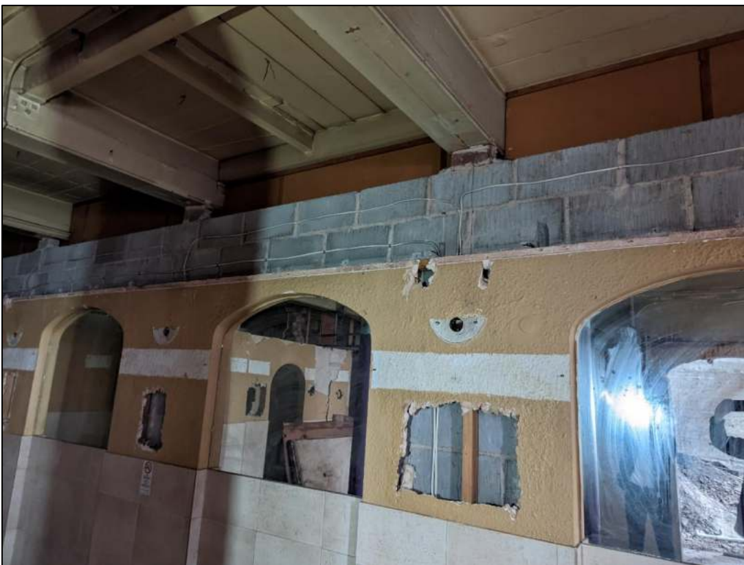
Plate 48: Inserted concrete block wall
