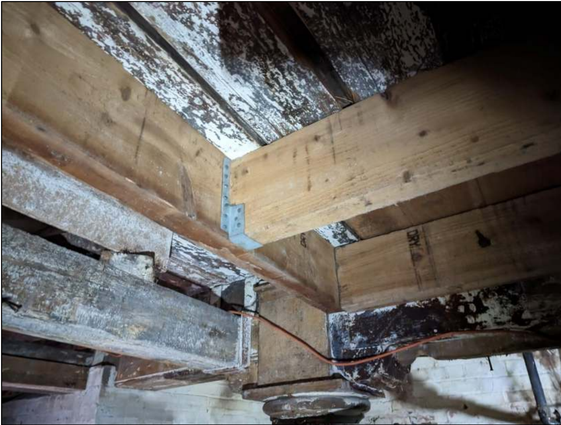
Plate 127: Inserted modern timber support
