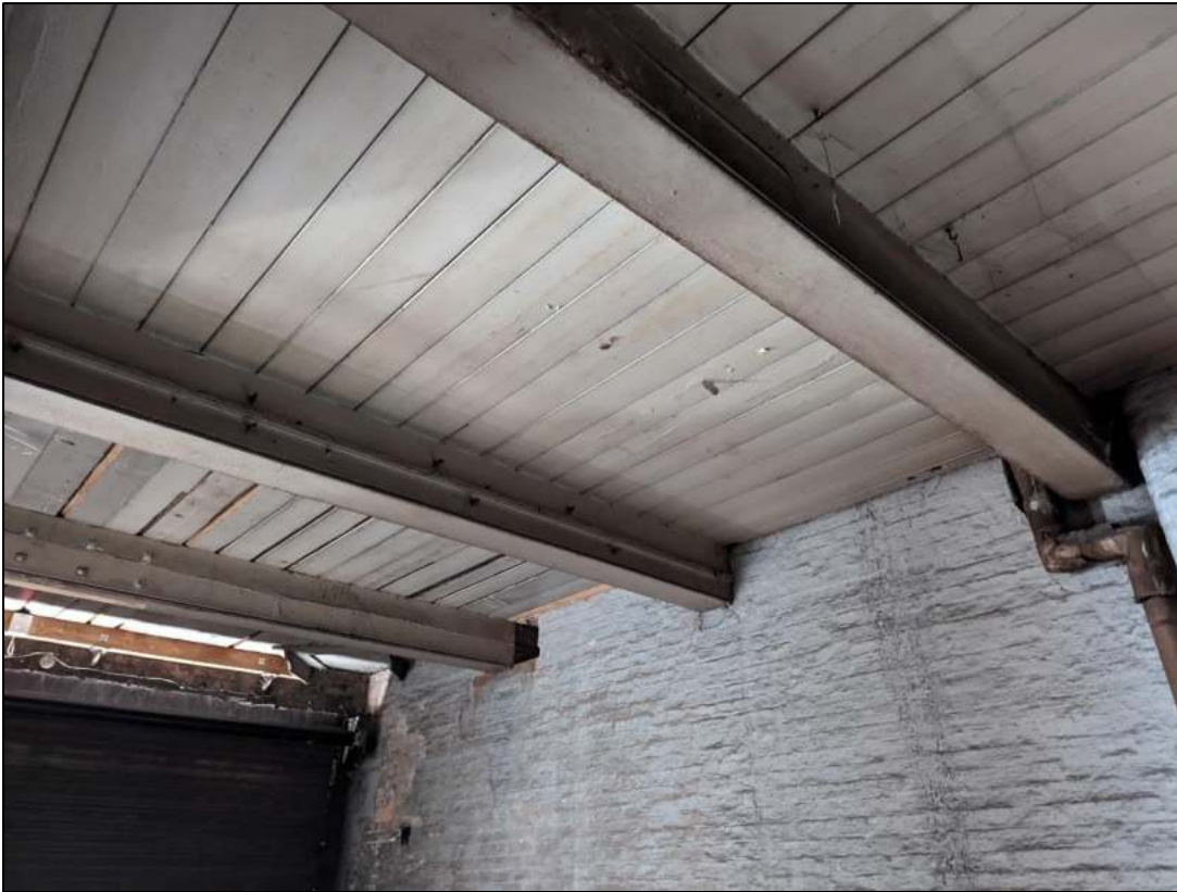
Plate 43: RSJ beams in loading bay
