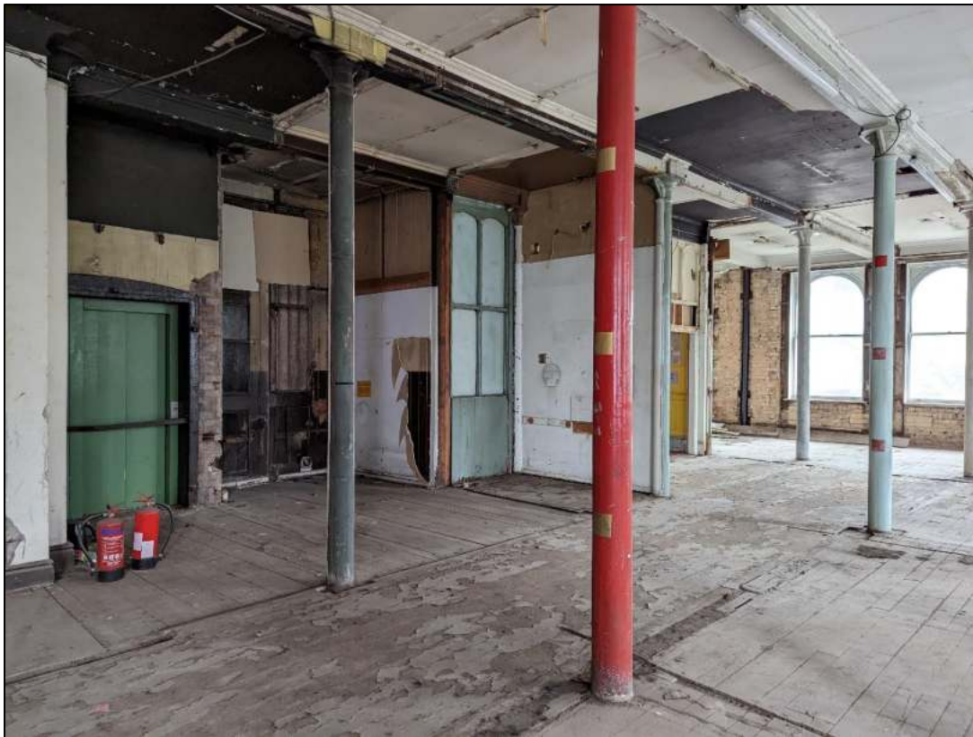
Plate 63: First floor showing lath and plaster walls
