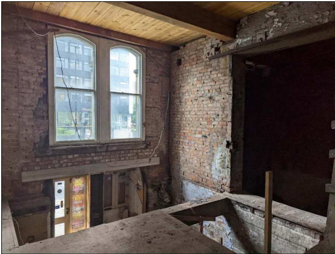
Plate 35: Area to south showing opening to loading bay
