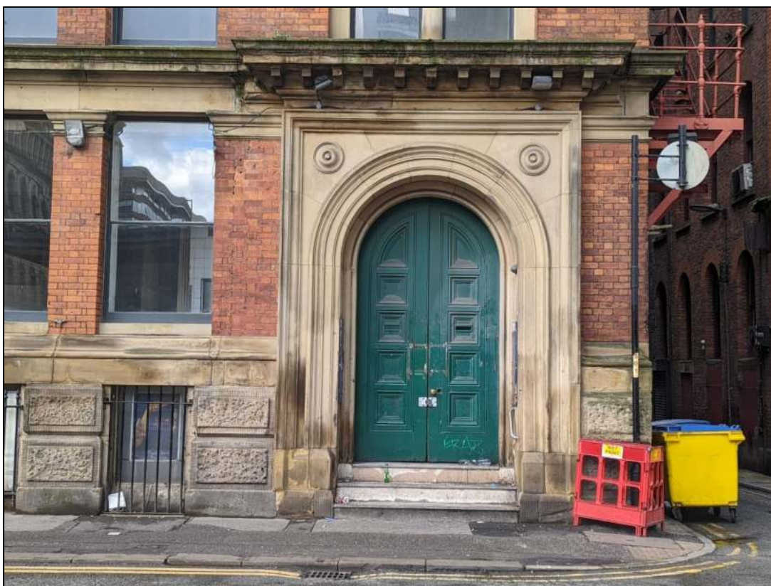
Plate 2: Detail of entrance
