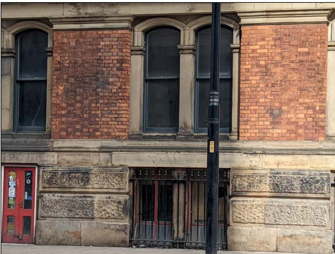
Plate 12: Ground floor windows and cellar lights below
