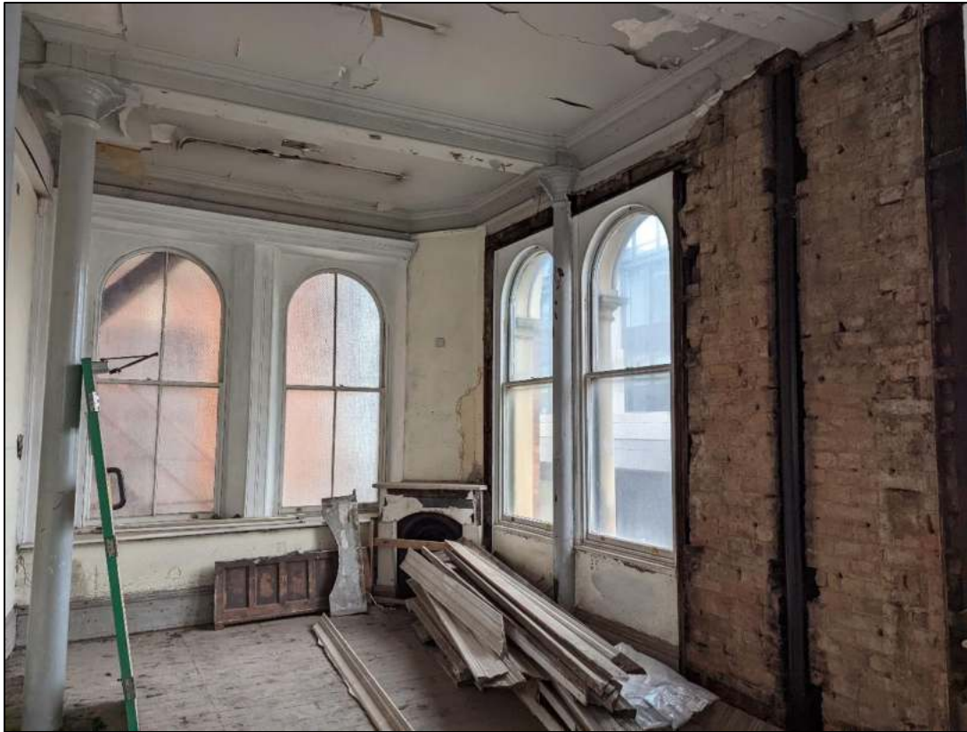
Plate 59: First floor showing original plaster
