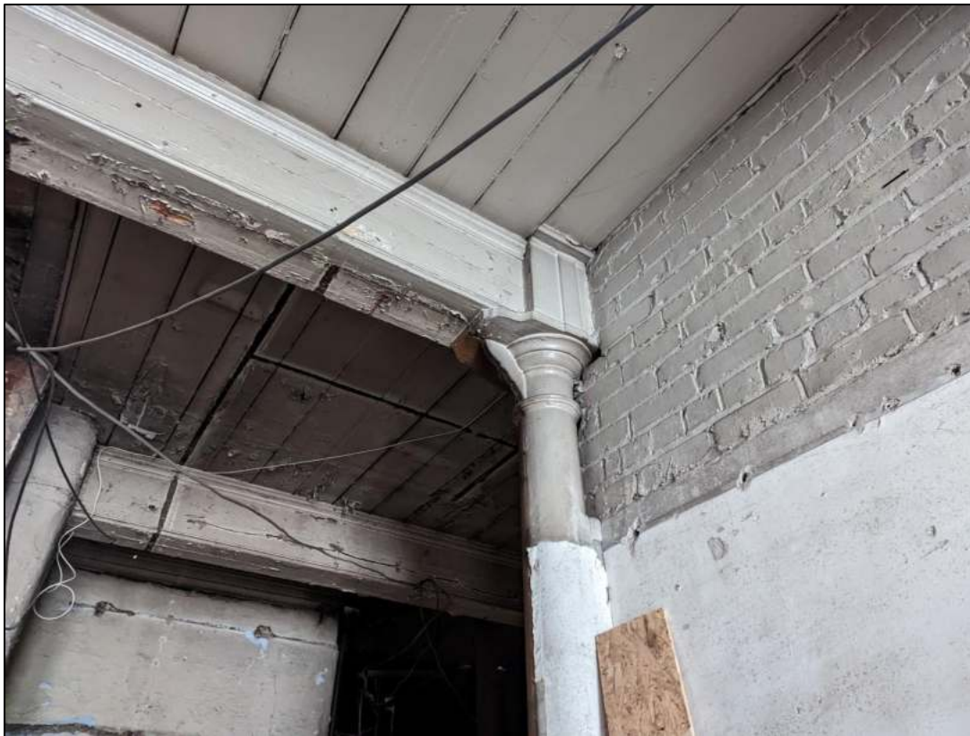
Plate 37: Cast iron stanchion , beam and ceiling boards next to early 20 th century wall
