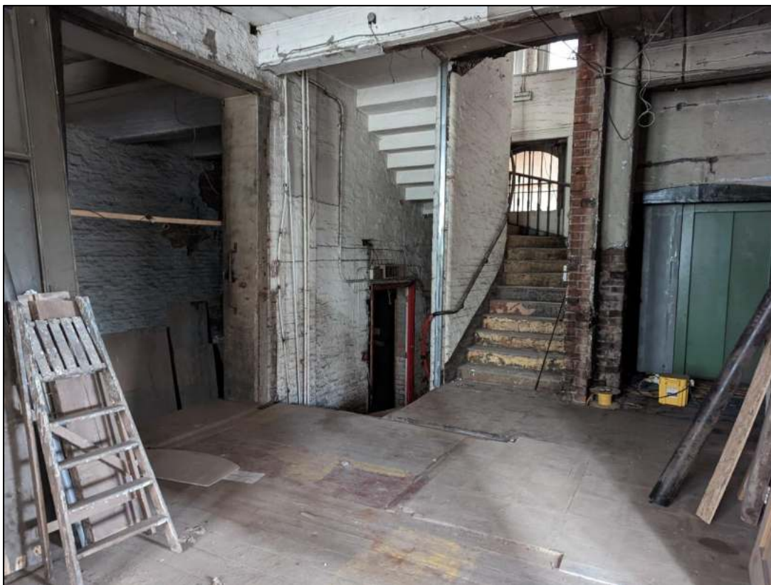
Plate 36: Area to south showing rear stairs
