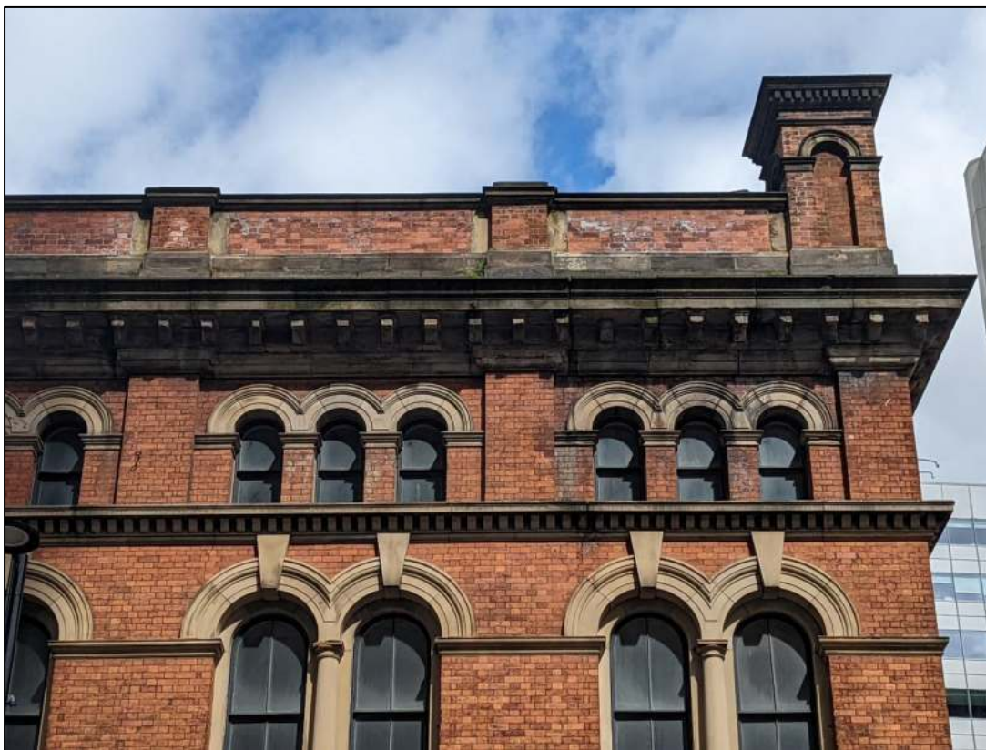
Plate 8: Second and third floor windows
