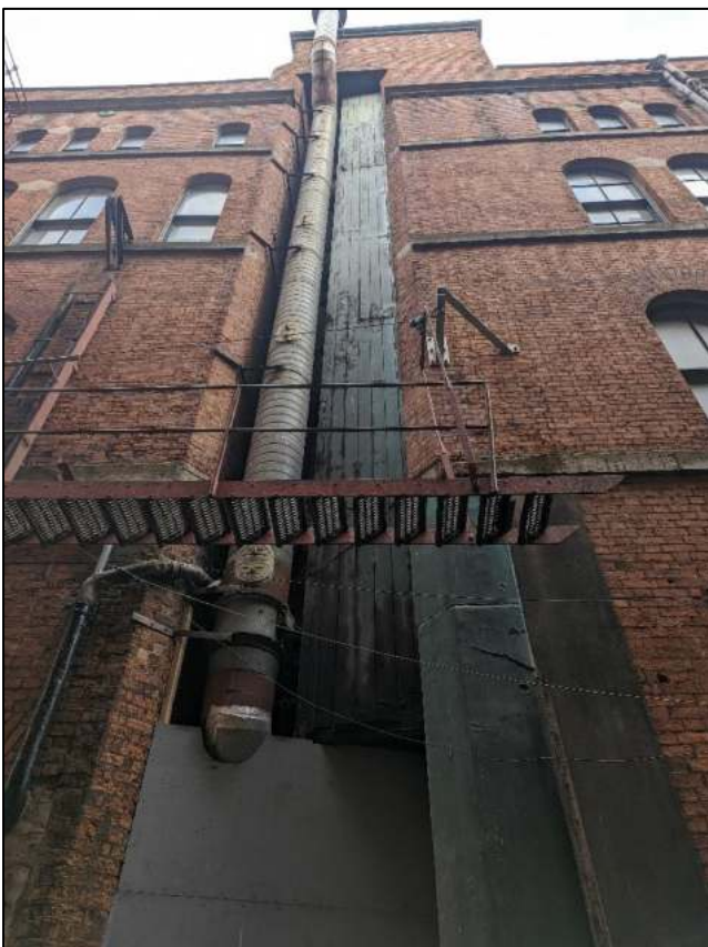
Plate 20: Recessed hoist shaft
