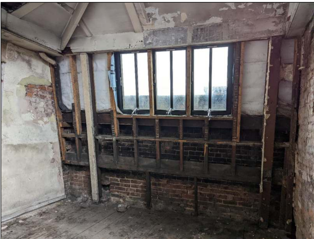
Plate 100: detail of inserted windows with timber framing
