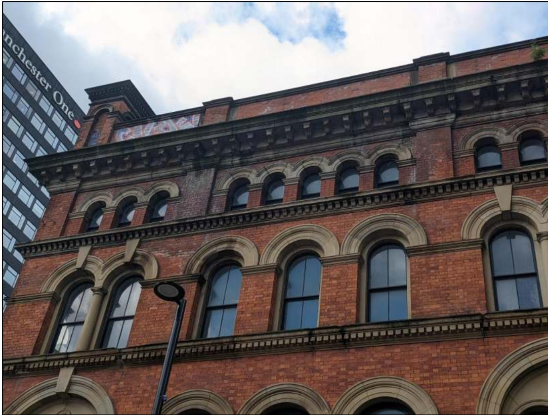
Plate 5: Second and third floor windows
