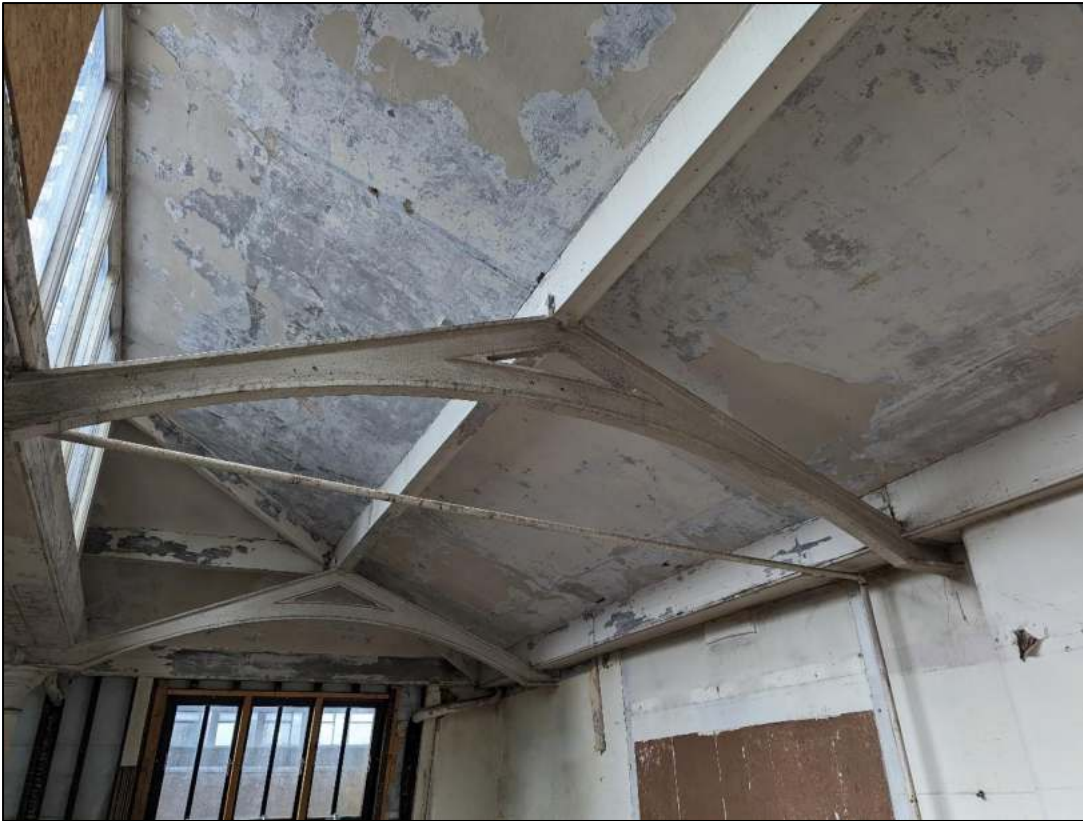
Plate 101: detail of cast iron trusses
