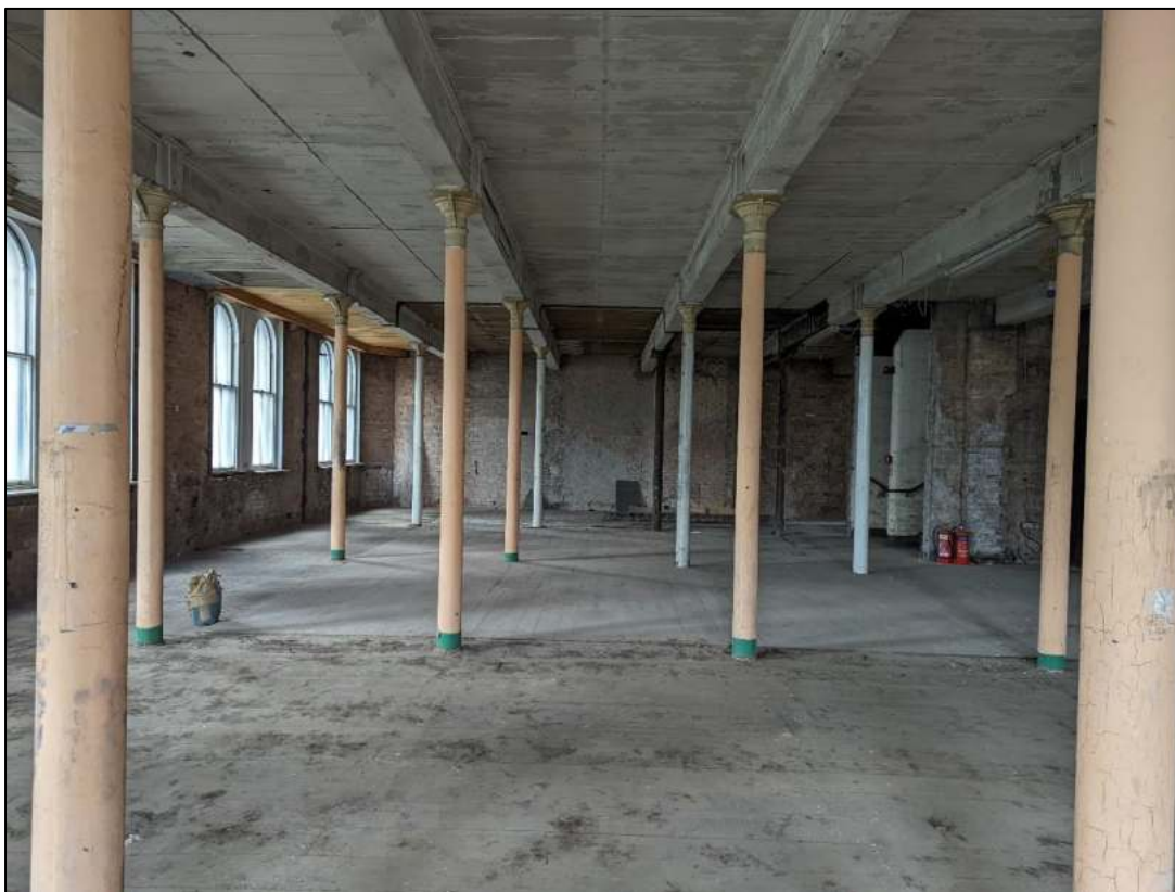
Plate 78: Second floor looking south
