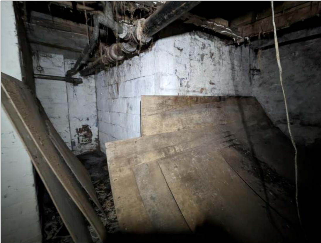
Plate 125: As above showing inserted wall
