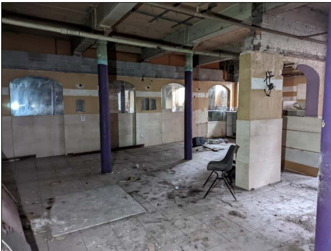
Plate 46: Lower ground floor showing modern fit out
