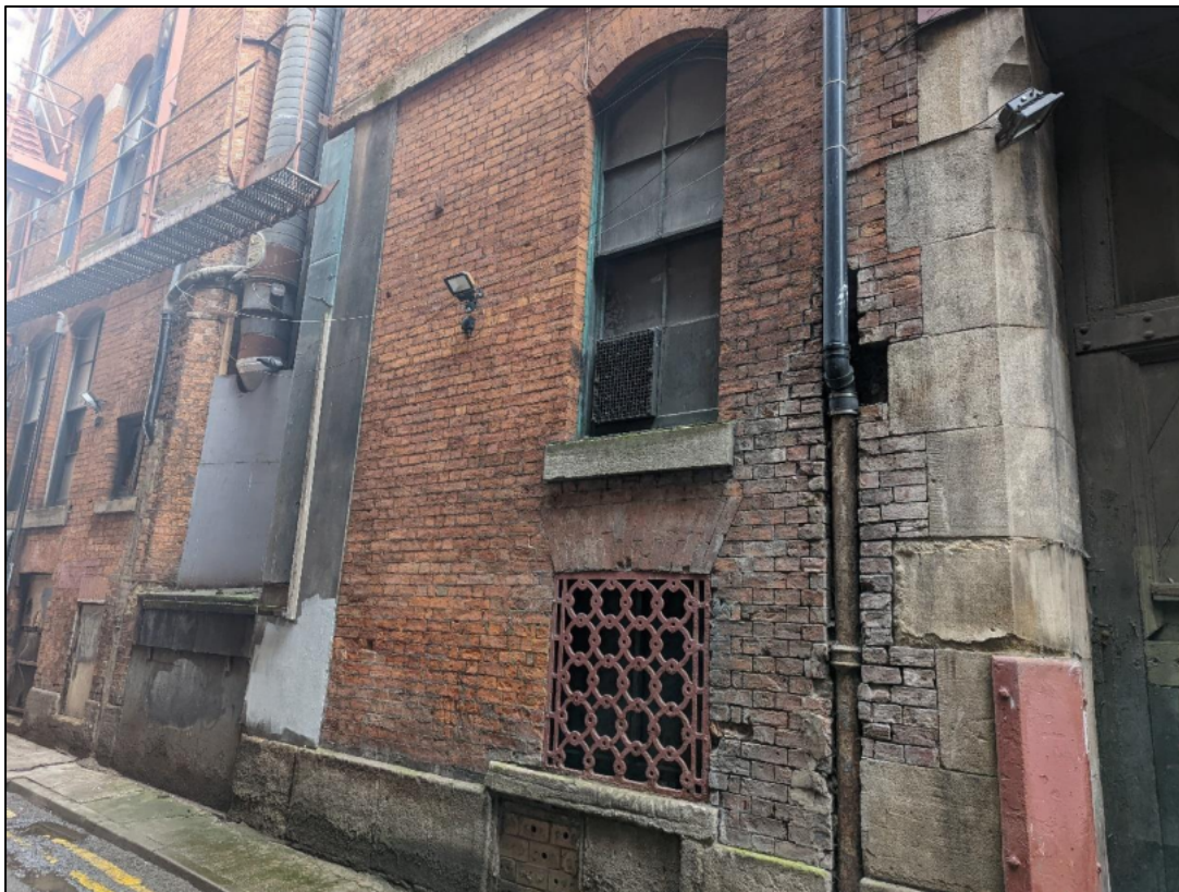
Plate 16: Ground floor bay 4
