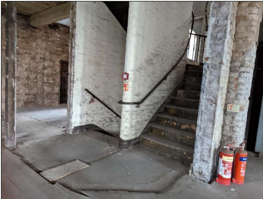
Plate 85: Base of staircase showing original timber with raised platform over
