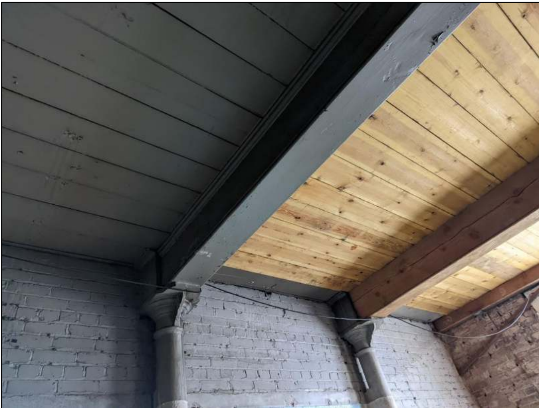
Plate 40: Original timbers and modern timbers in ceiling
