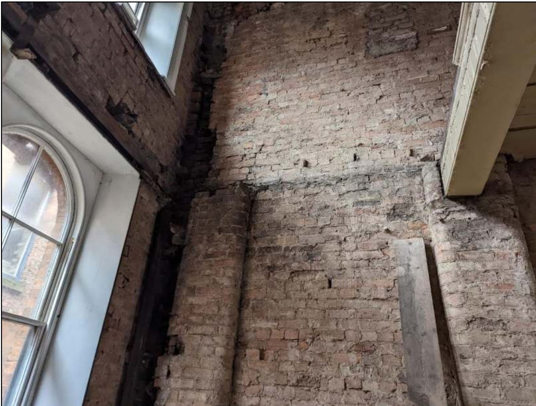
Plate 84: Removed ceiling detail
