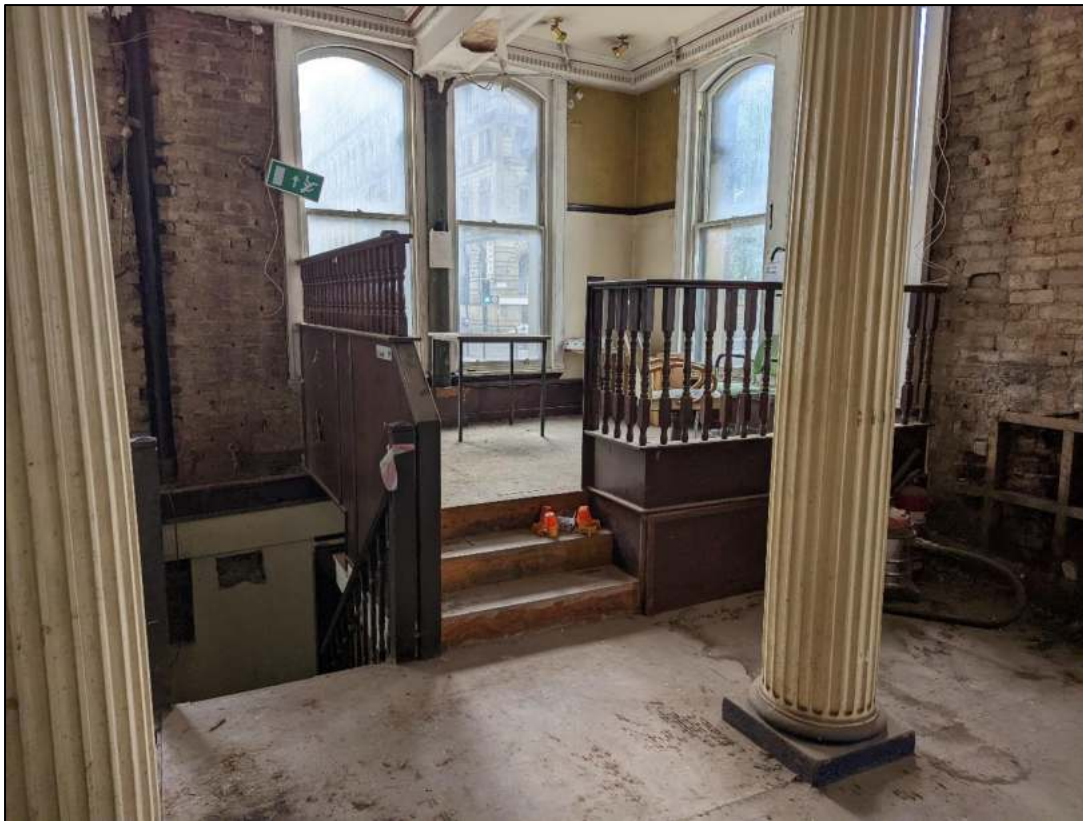
Plate 33: Inserted raised platform and staircase
