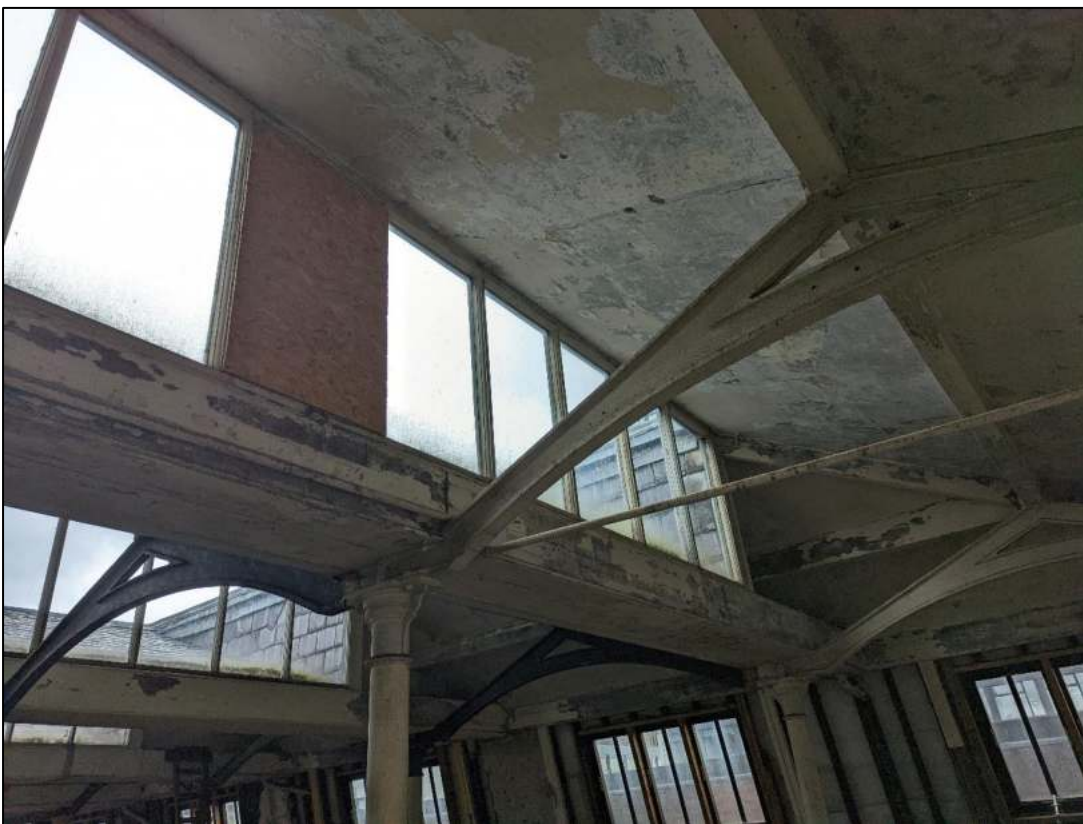
Plate 102: Northlights over timber beams
