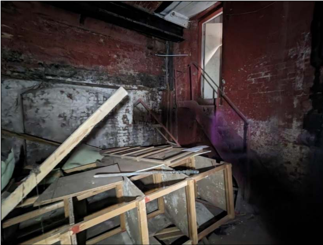
Plate 111: As above showing cast iron staircase
