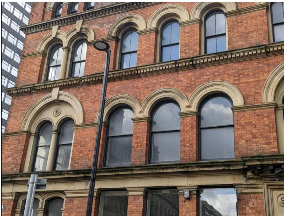
Plate 4: First and second floor windows
