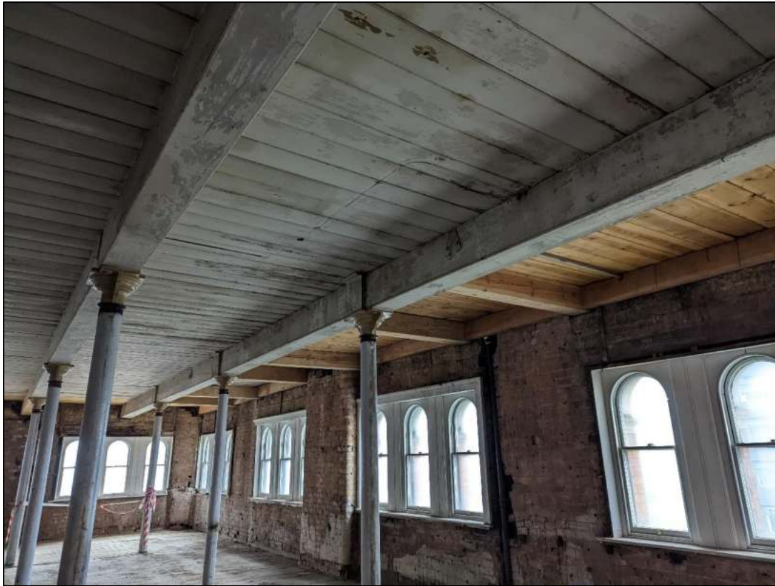
Plate 89: Ceiling showing original and modern timbers
