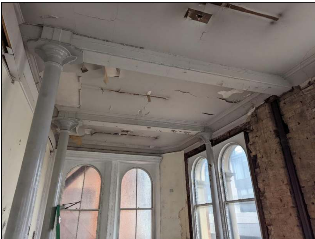
Plate 60: Ceiling showing cornice, beams and lath and plaster
