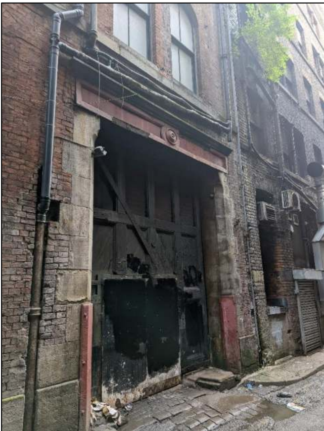
Plate 14: Loading bay to bay 5
