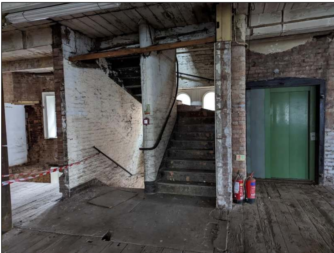
Plate 92: Staircase to fourth floor
