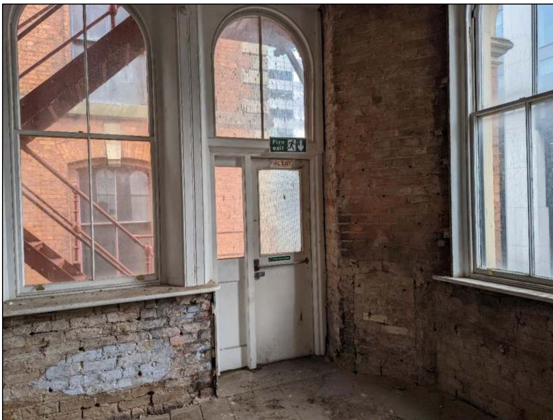
Plate 80: Inserted fire escape door in former window with blocked corner fireplace adjacent
