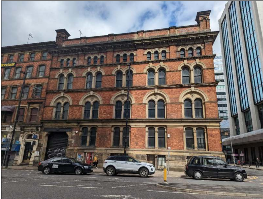
Plate 7: East elevation to Portland Street
