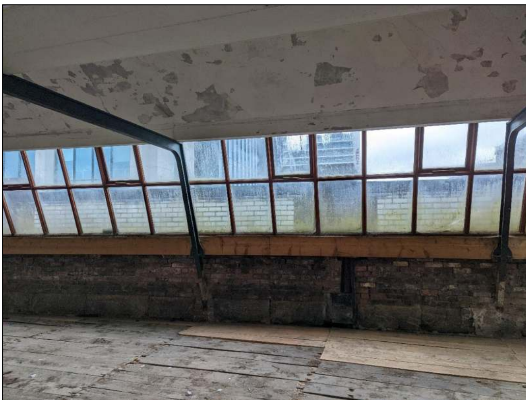
Plate 106: Inserted windows along north wall
