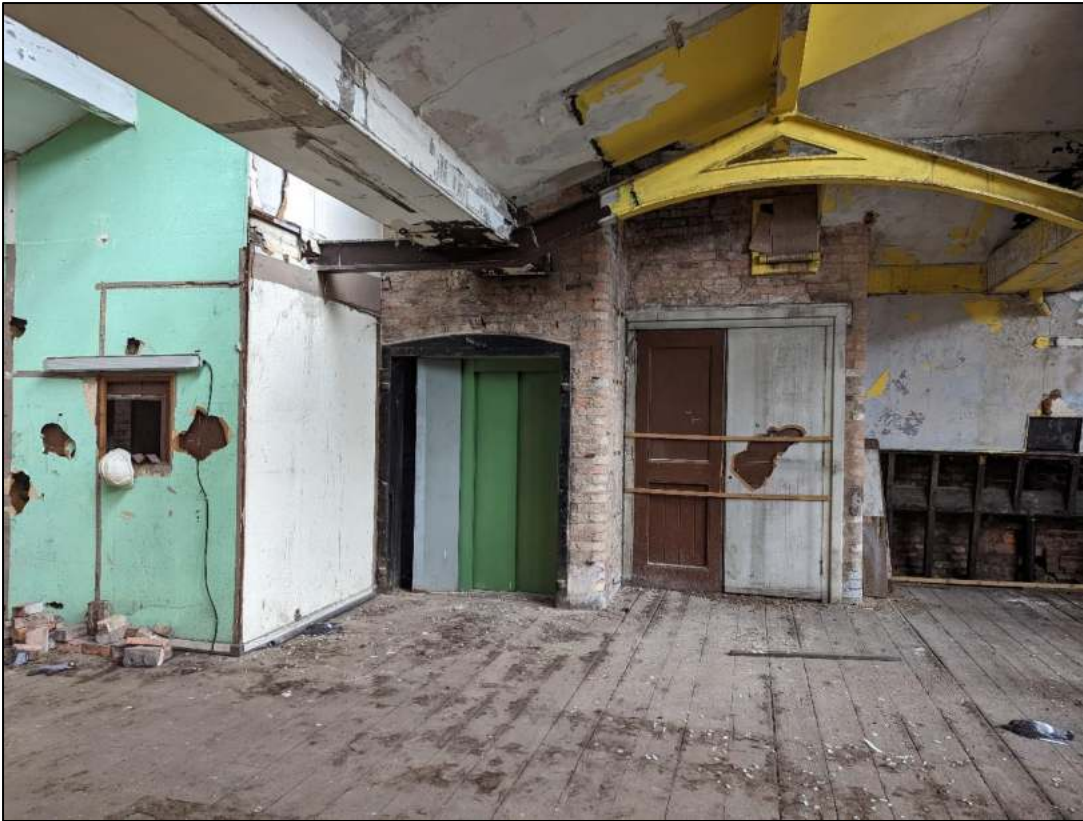
Plate 103: Lift and hoist
