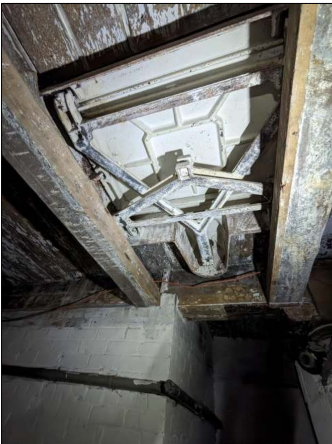
Plate 128: Metal hatch in ceiling
