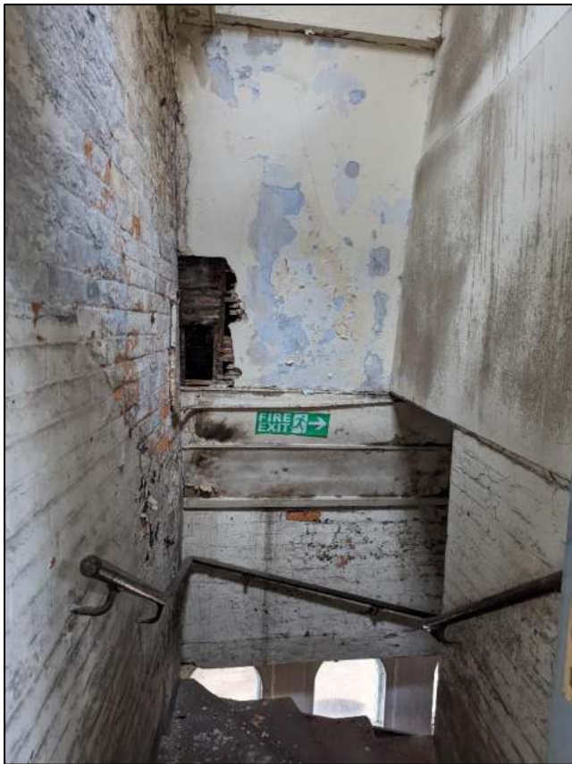
Plate 97: Staircase to fourth floor
