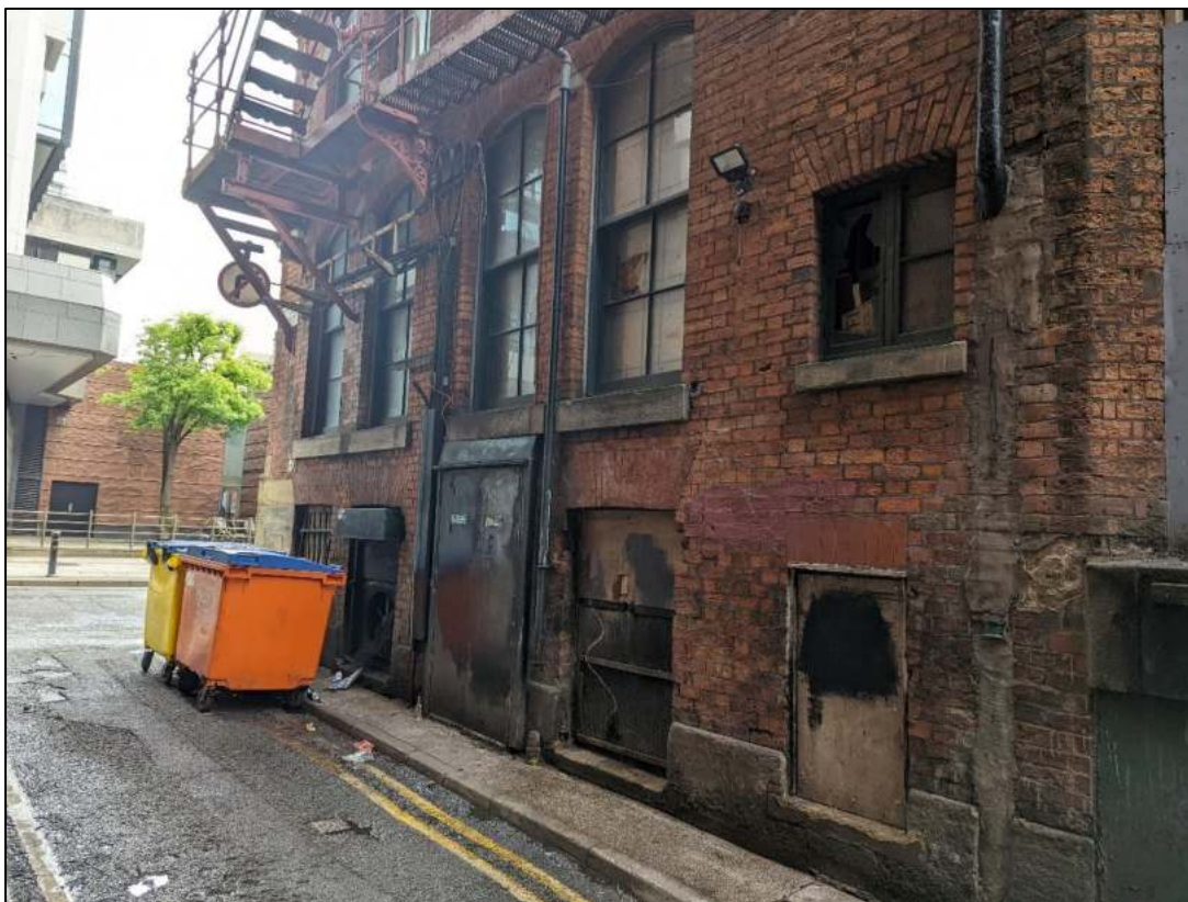
Plate 18: Ground floor to bays 1 - 3
