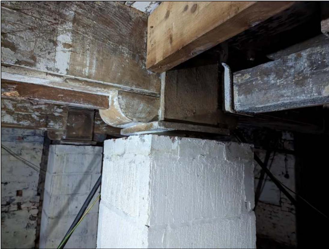
Plate 123: Concrete block around stanchion
