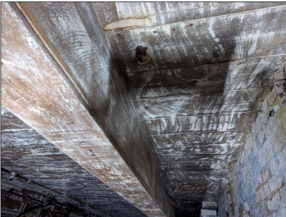
Plate 122: Timber boards of ceiling
