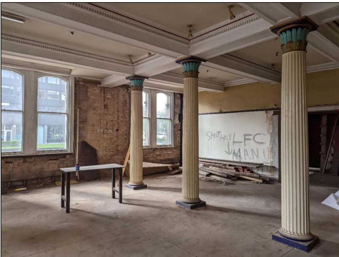
Plate 26: Former banking hall
