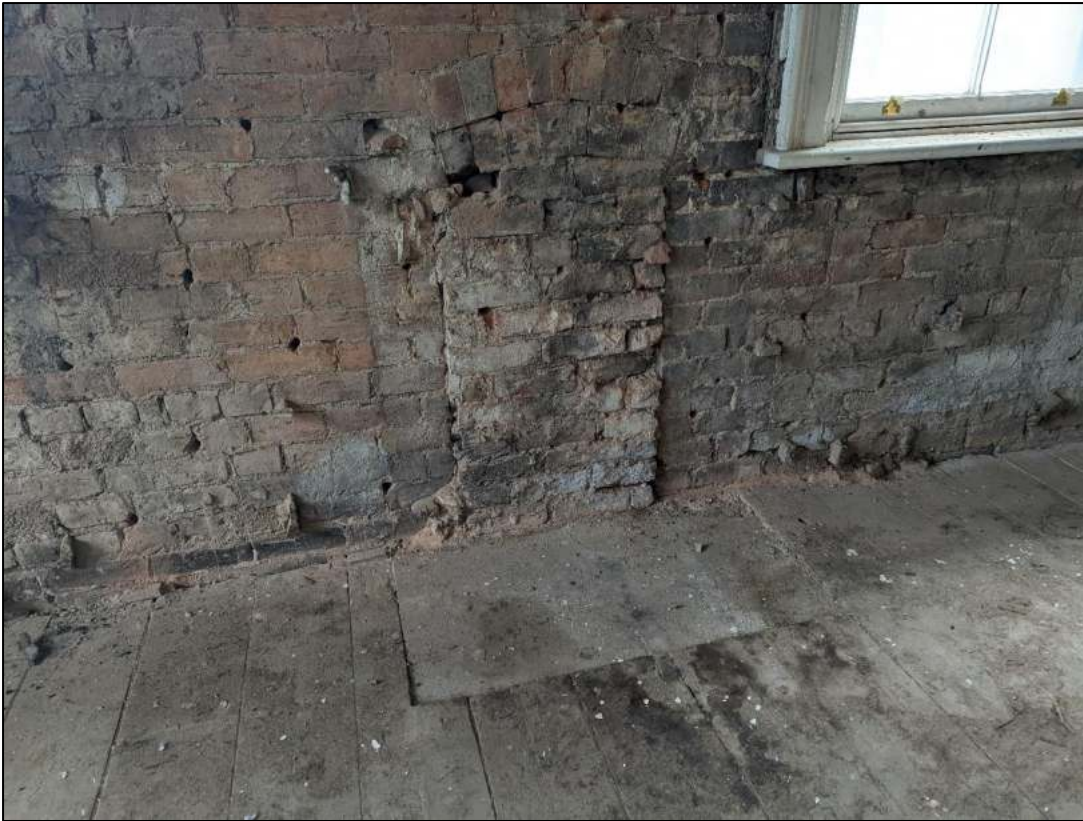
Plate 81: Blocked fireplace with hearthstone in east elevation
