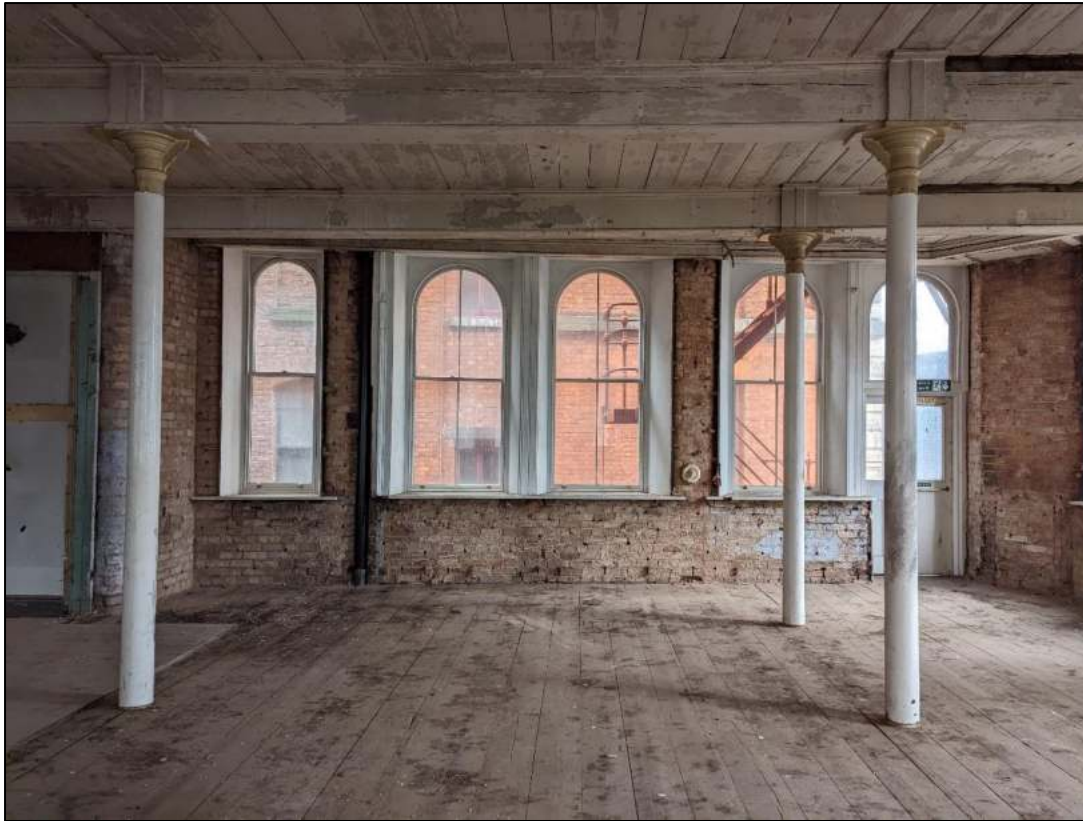
Plate 77: Window details showing timber floor and beams
