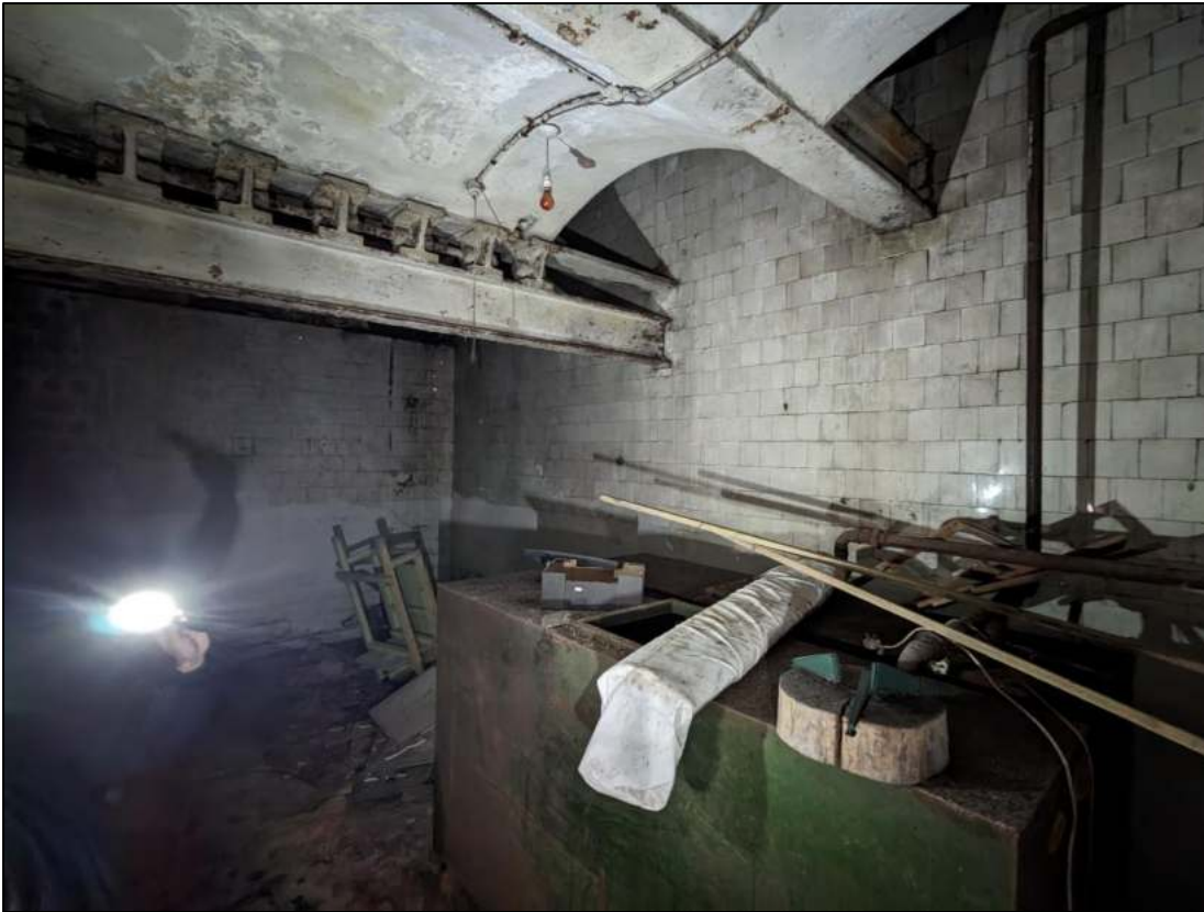
Plate 117: East end of basement showing tiled walls
