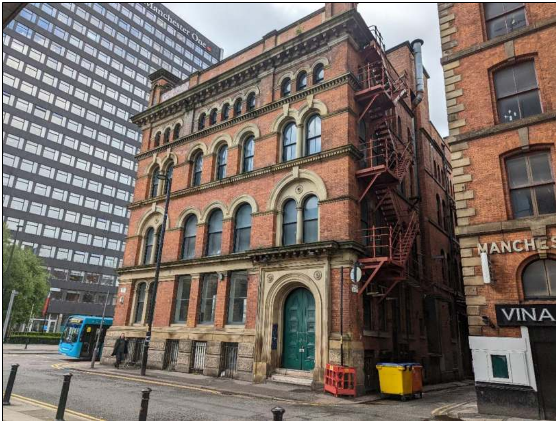
Plate 1: North elevation to Charlotte Street
