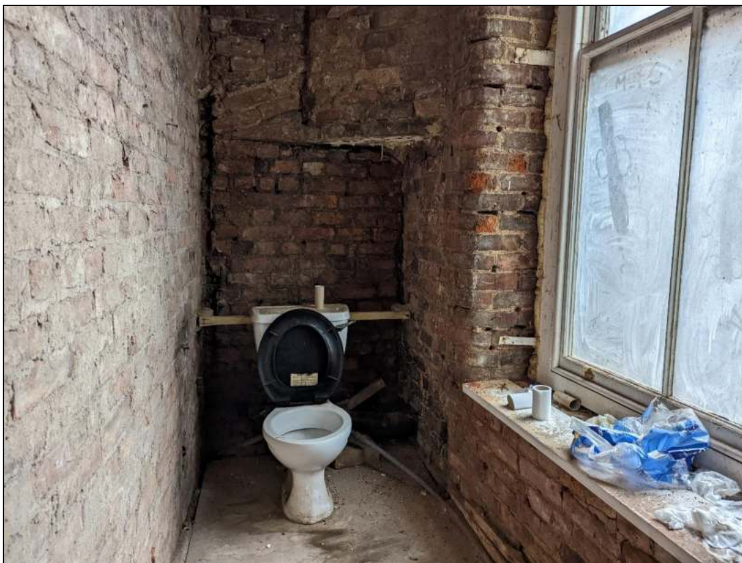
Plate 66: Inserted toilet in place of corner fireplace
