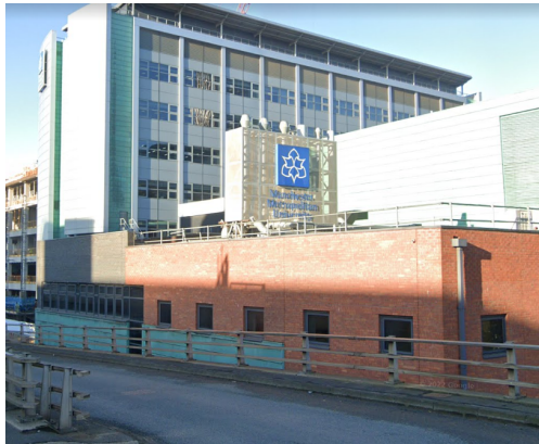
Existing Sign to be Replaced
