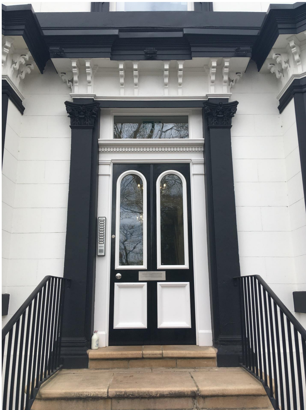
Plate 24: Front Door and entry stairs. Door frame and surrounds repaired and restored as part of conversion of building to flats
