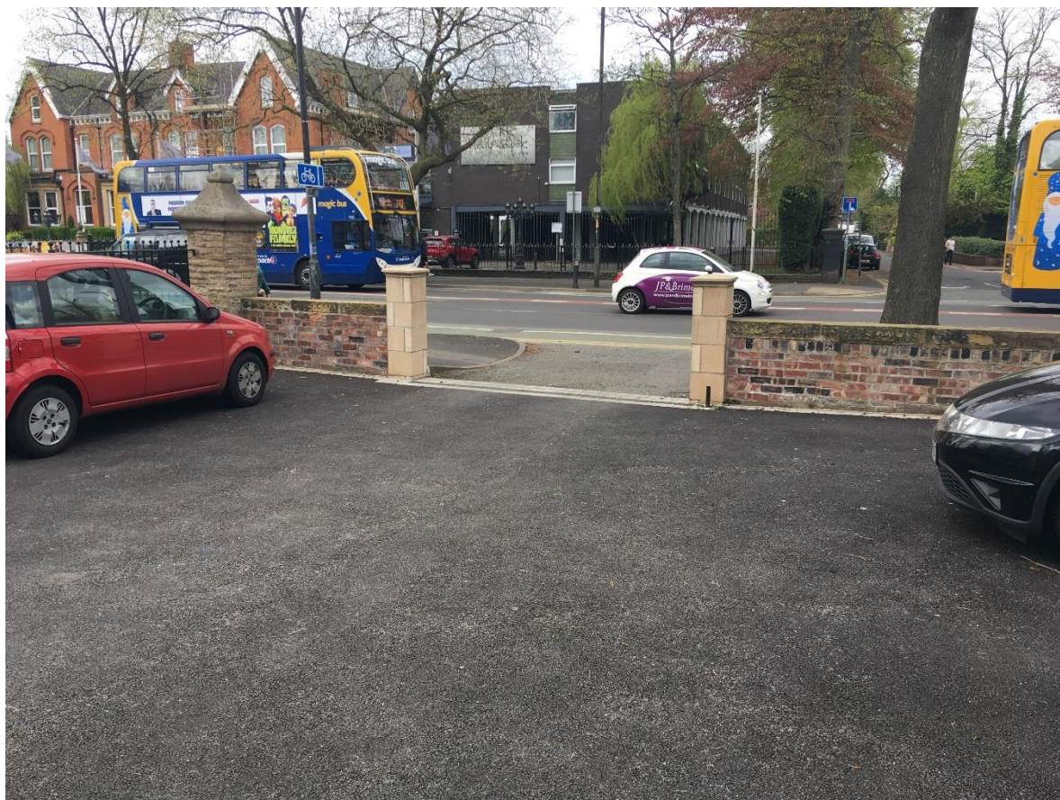
Plate 25: Rebuilt Entrance Piers and tarmacadam parking area
