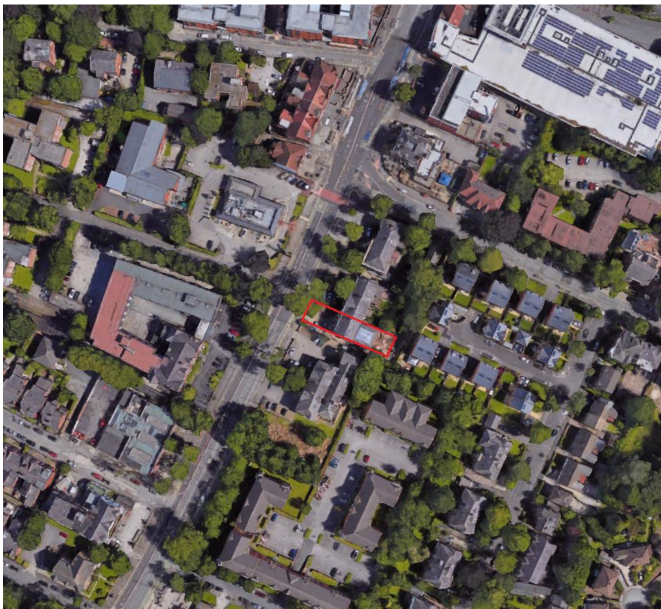
Figure 1: Aerial view of 363 Wilmslow Road (outlined in red).
