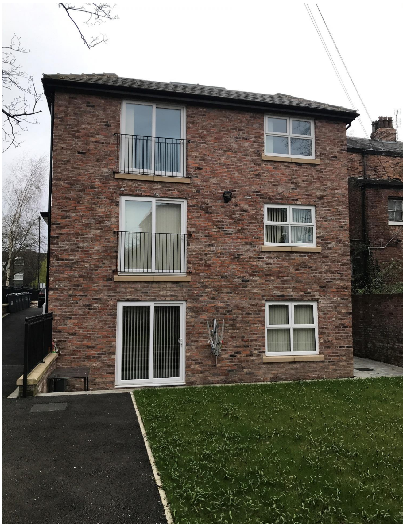
Plate 23: Rear extension from the east subject of the 2019 appeal.
