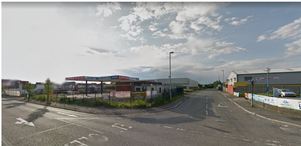
Streetview picture of the site from 2012 showing the remnants of the former Filling station canopy
