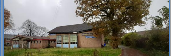
The Greenbrow Road elevation of the social club that occupies the application site
