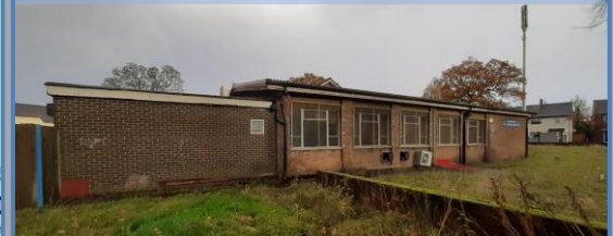
The Newall Road elevation of the social club
