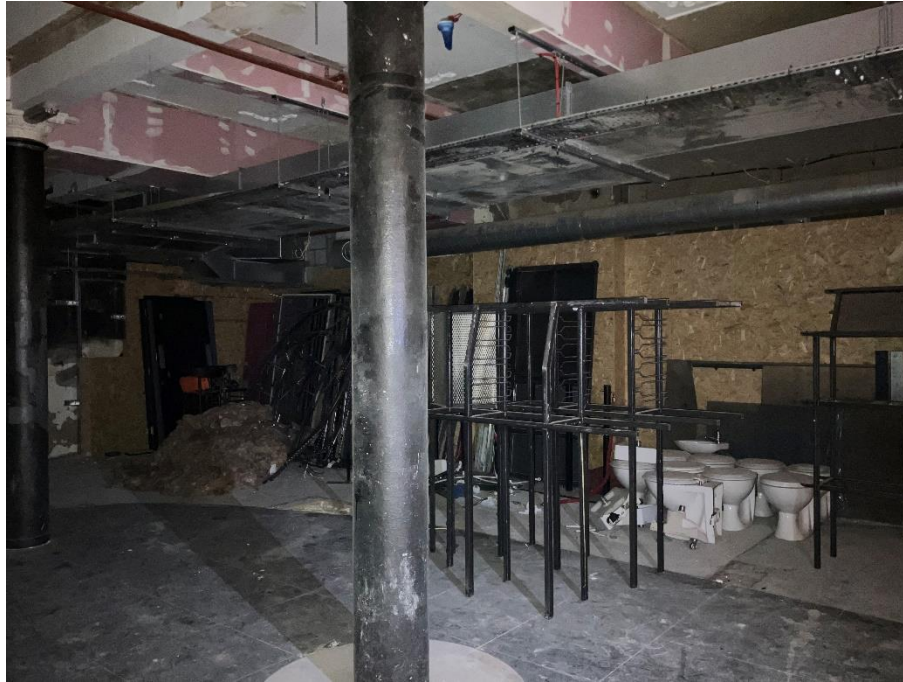
Figure 3 - Main basement interior (RJP, April 2023)
