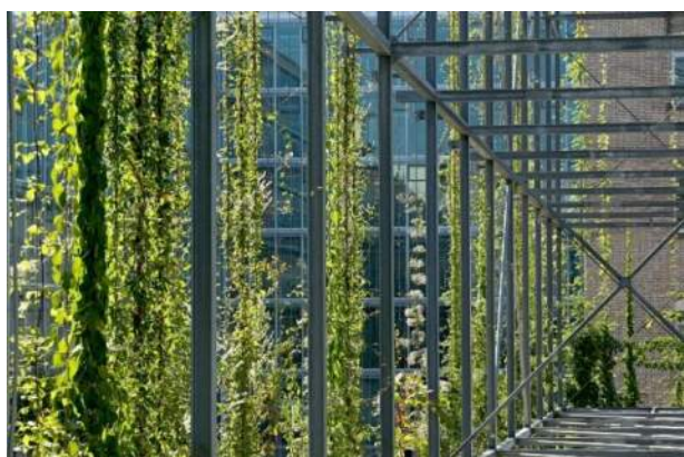
Figure 6—5 Cable green wall (MFO Park, Zurich)
