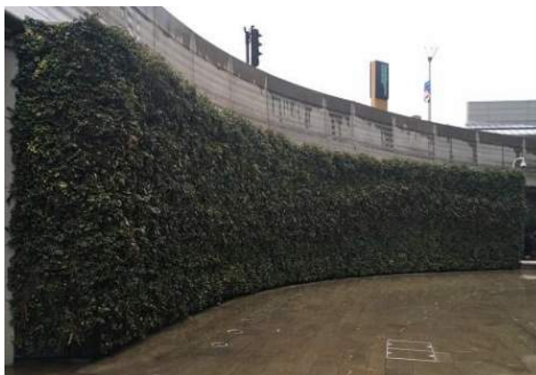
Figure 6—6 Modular green wall (Paddington, London)
