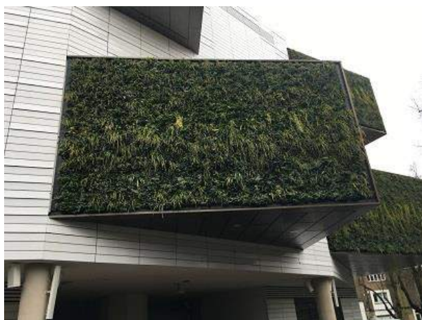
Figure 6—7 Modular green walls (Lord's Cricket Ground, London)
