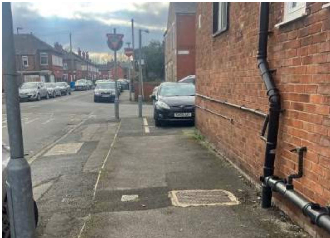
Photo 3—Allanson Road side of existing structure, showing service hatches.
