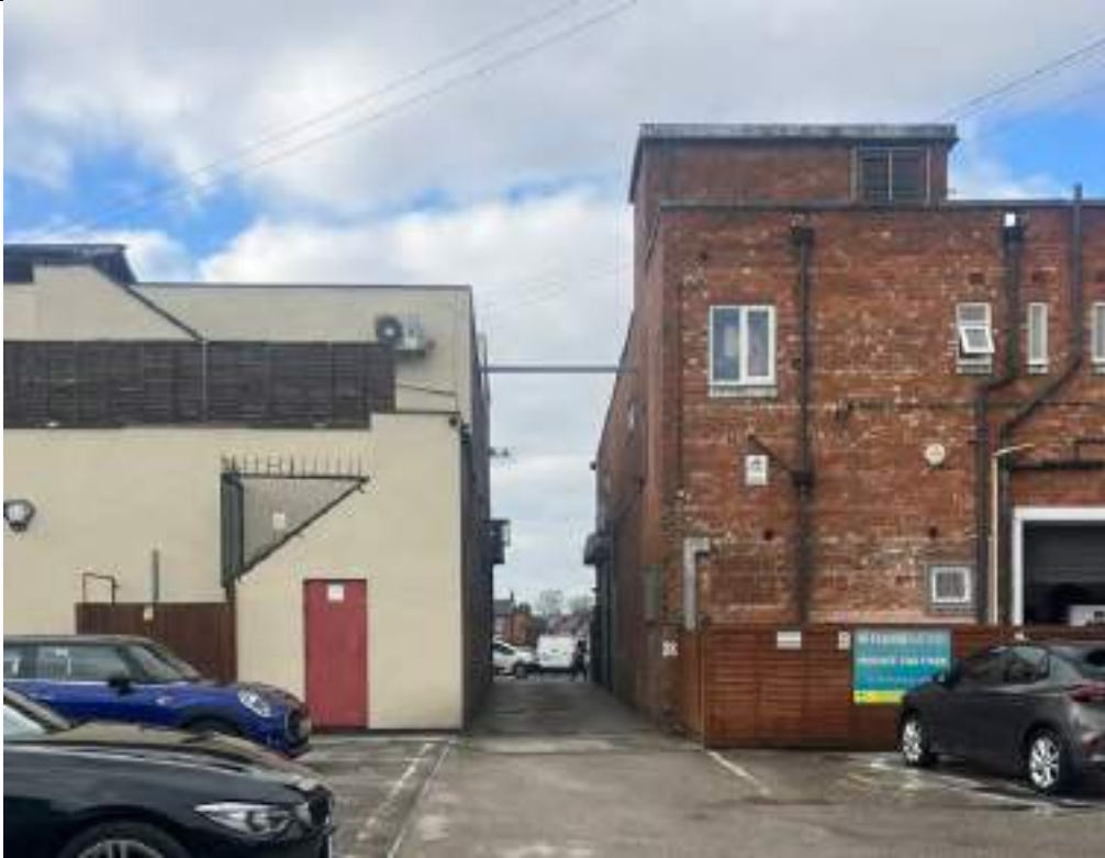
Photo 8—Rear view of alley between 317-319 Palatine Road, and 315 Palatine Road, from Allanson Road.
