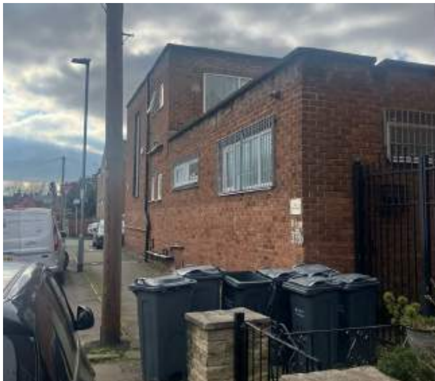
Photo 5—Rear corner and gated alley behind Allanson Road side of structure.
