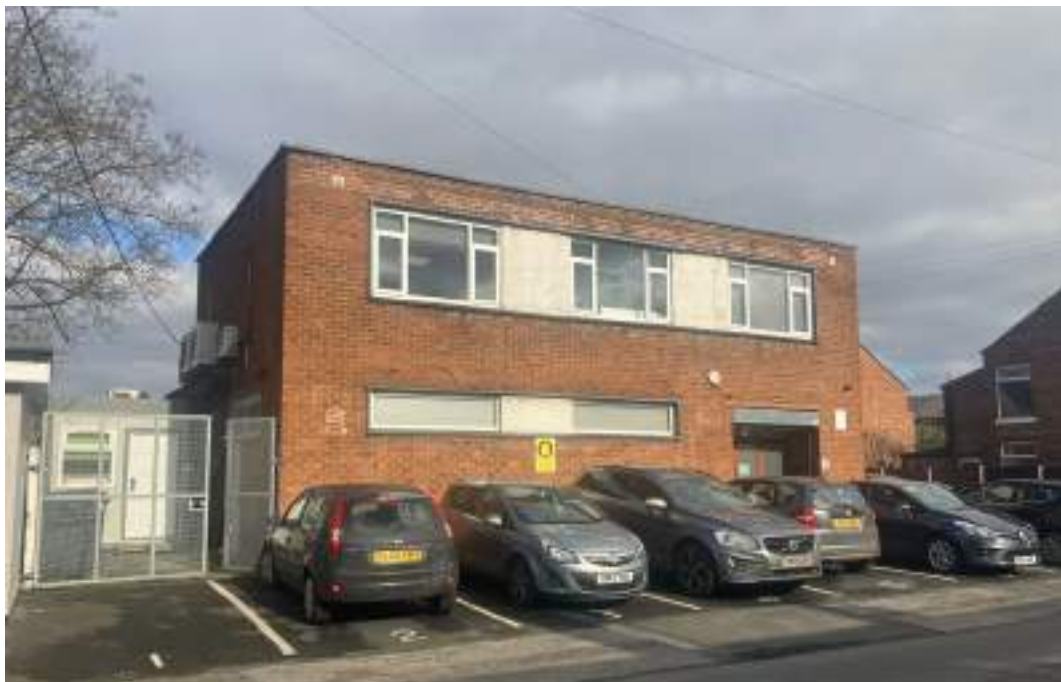
Photo 1—Existing building and car park on Brett Road.
