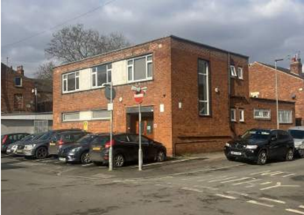
Photo 2—Existing building and car park on Brett Road.
