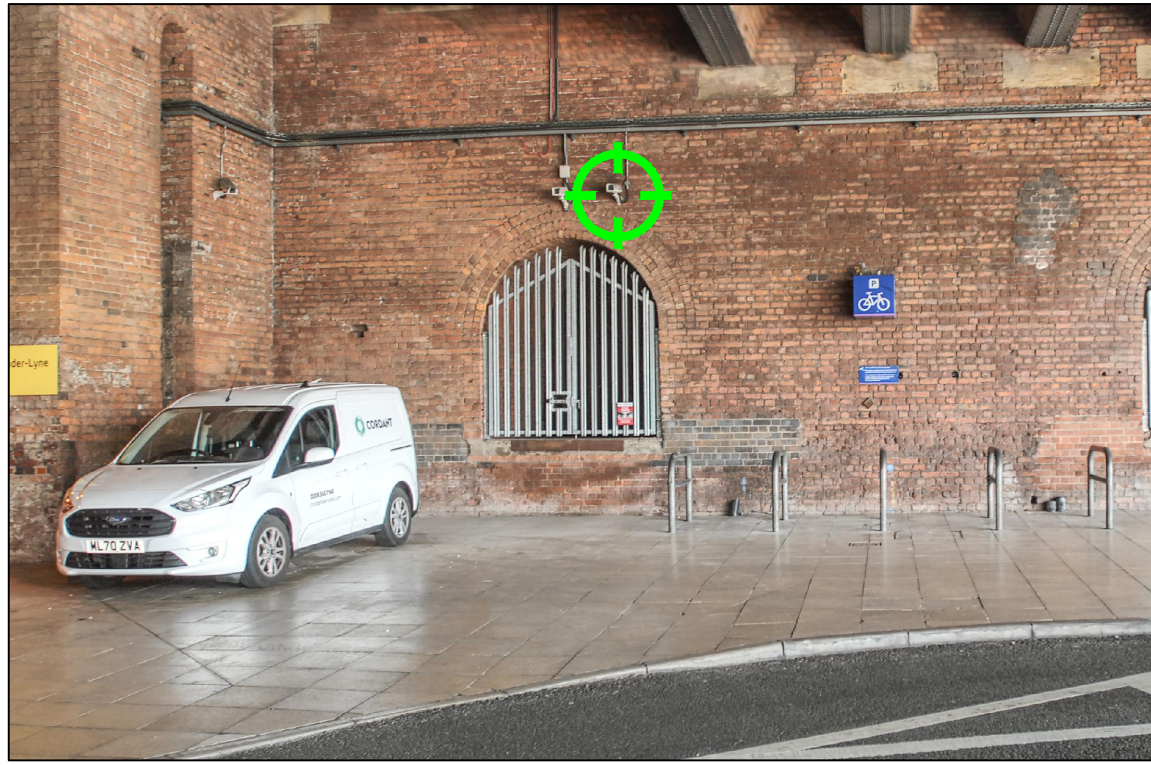
PERSPECTIVE VIEW D - EXISTING APPLIES TO CAMERAS 24295 AND 24296
