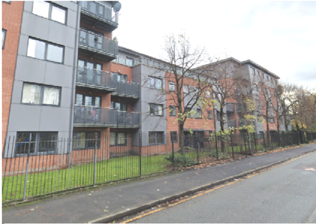
Fig 3.2.1a Apartment block less than 200m away on Lloyds Street with steel railings
