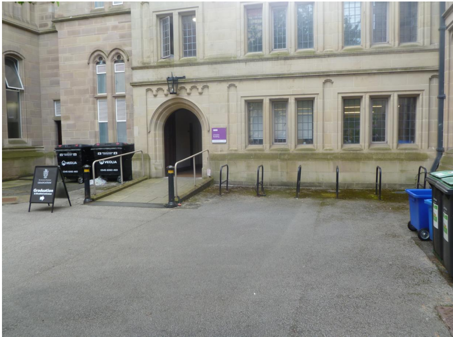
Figure 5.2: Existing ramped entrance to the rear of the Christie building
