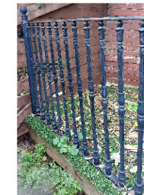
Image of existing cast iron railing
