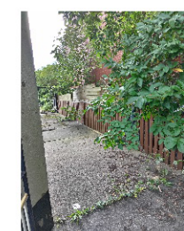
Image of existing wooden fence
