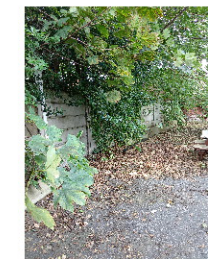
Image of existing concrete fence
