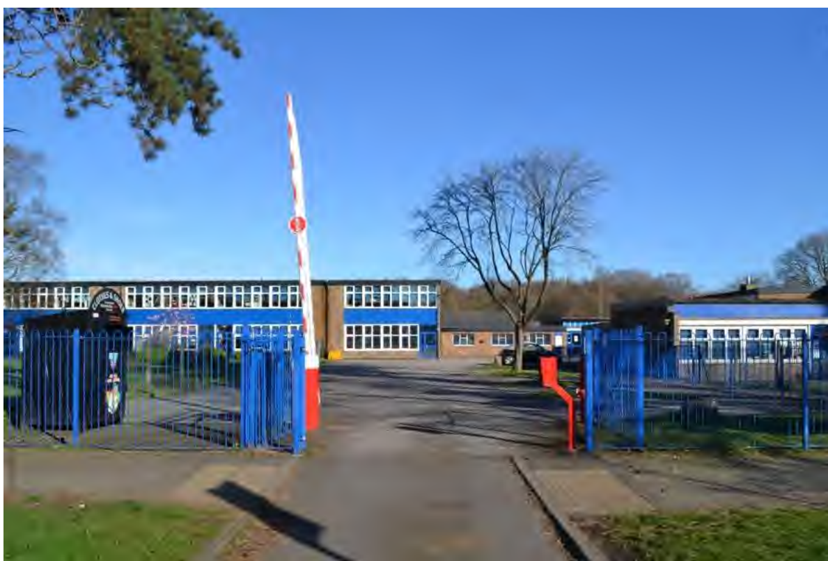
Plate 24: Sightline through the western vehicle entrance towards the school.
