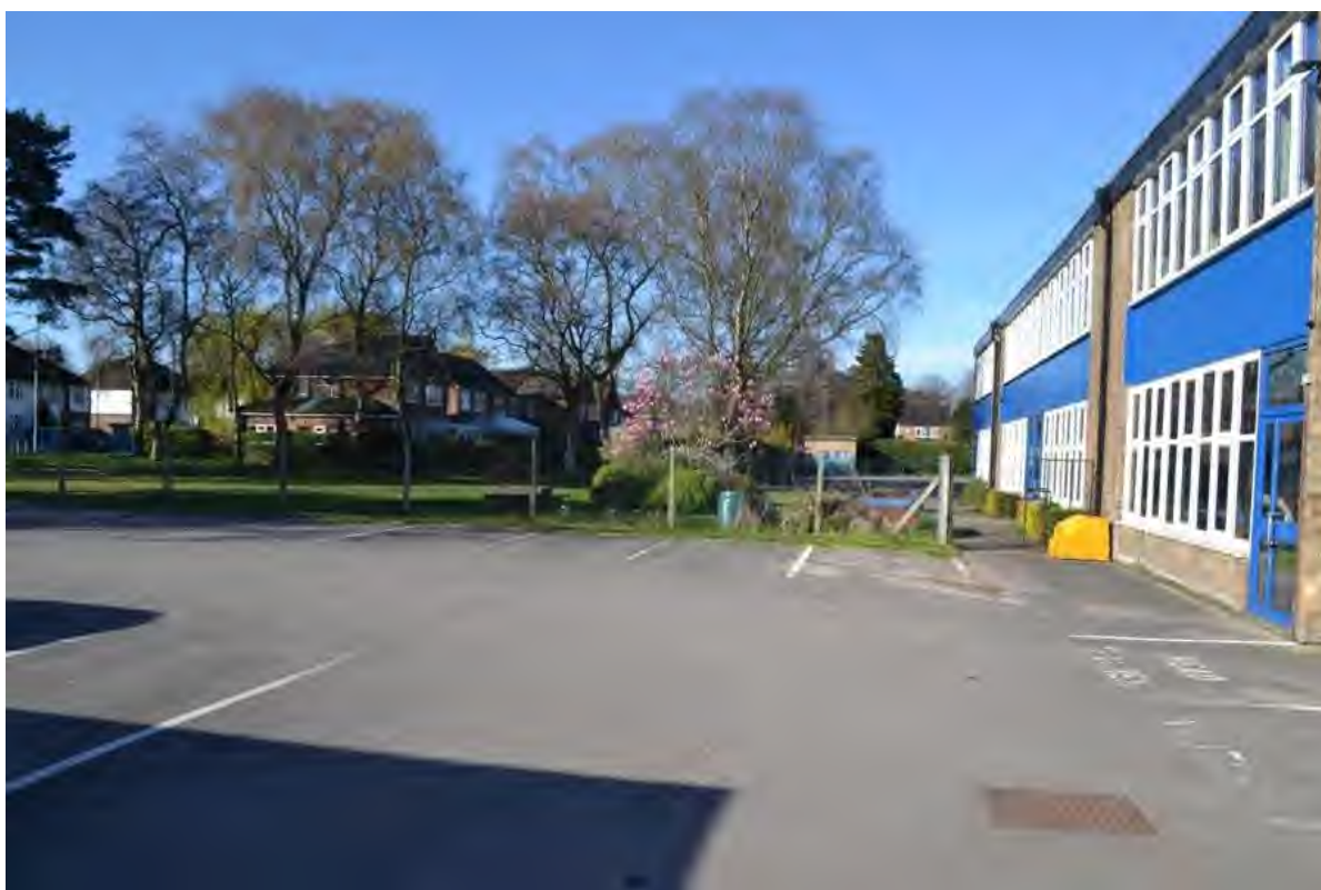
Plate 30: Sightline to the west along the front façade of the main bloc of the school
