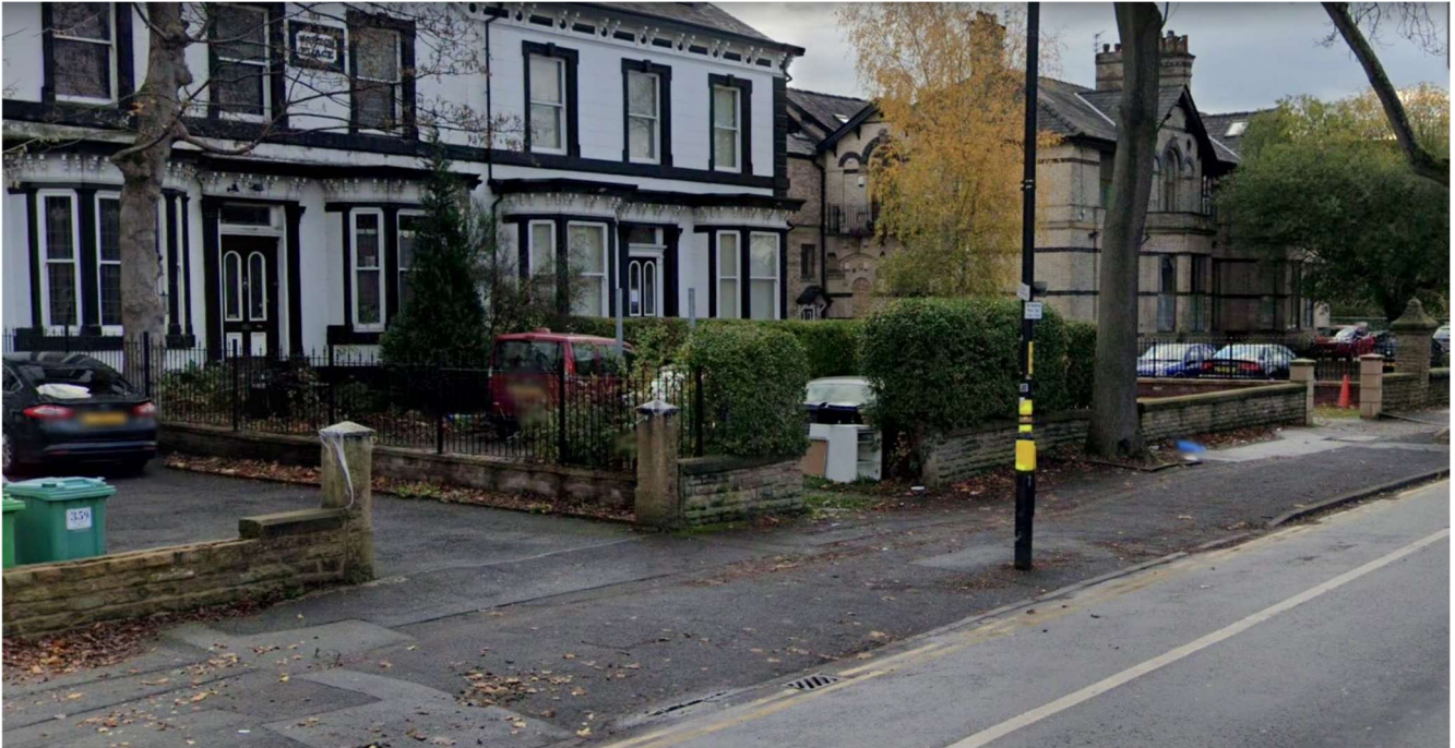
Fig 29. The original stone gateposts to the front of 359 Wilmslow Road and to the far right the modern artificial stone gateposts to the front of 363 Wilmslow Road
