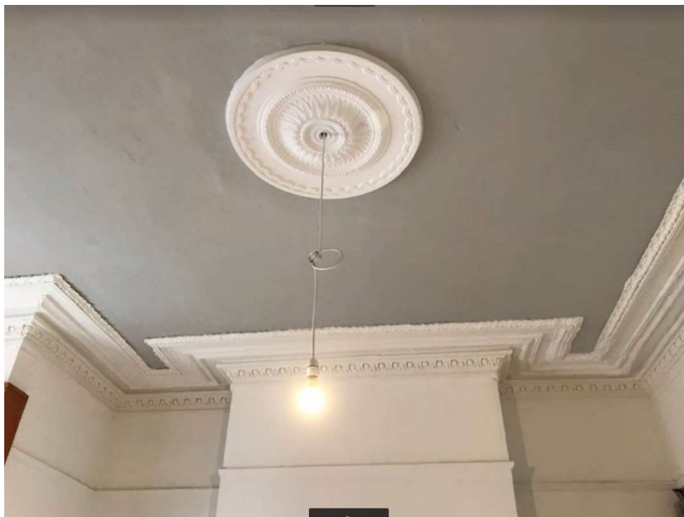
Fig 4. Internal decorative cornice and picture rail to 359 following restoration.
