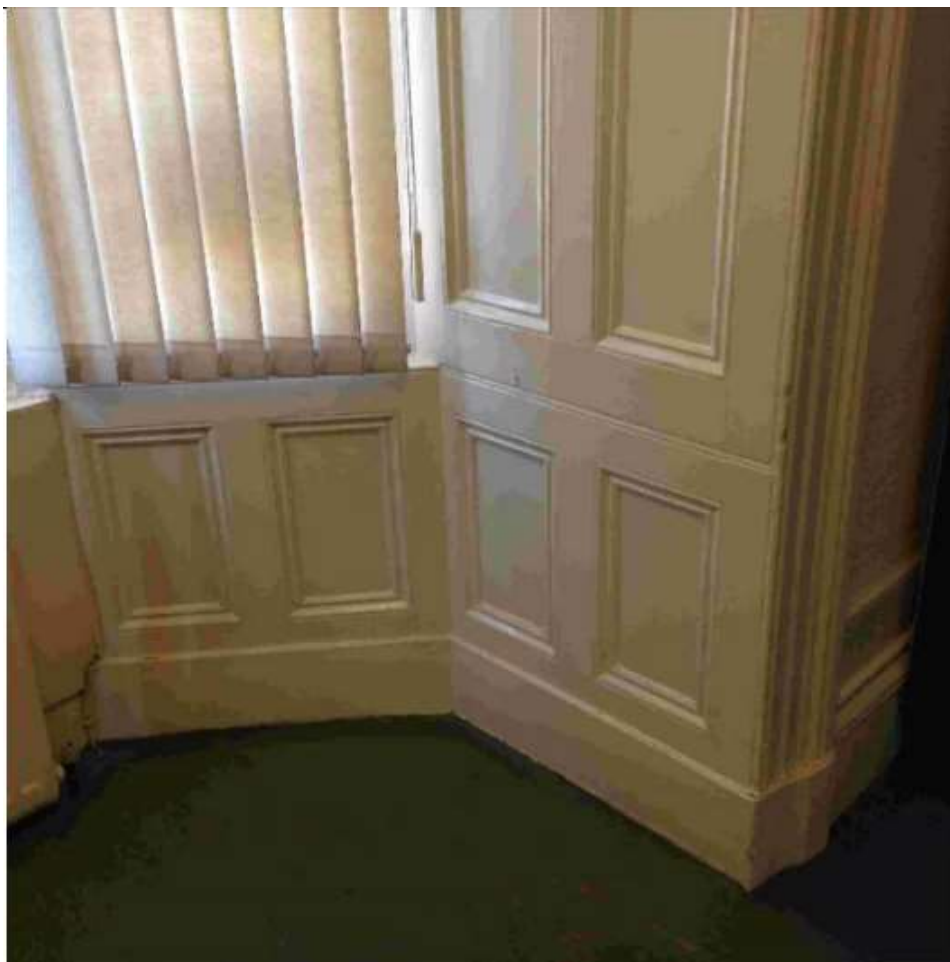
Fig 19. Internal front room to 363 showing prior to works original timber panelling (now removed).
