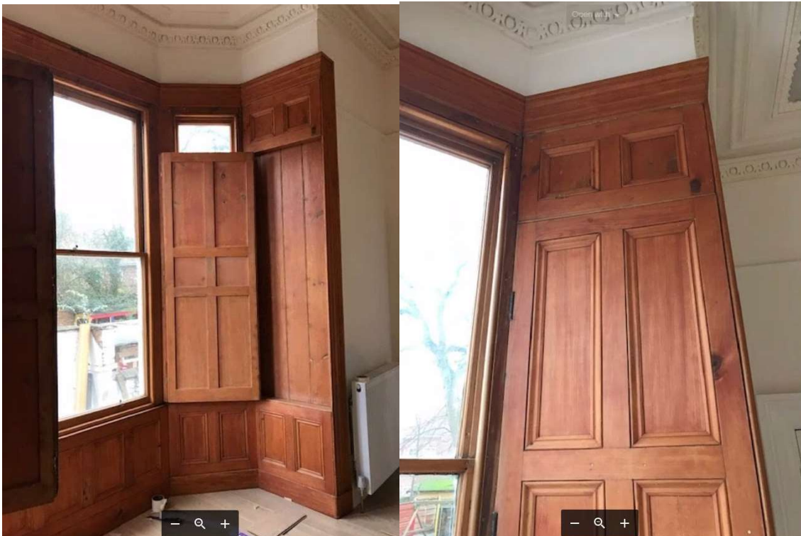
Fig 22 and 23. Internal room at 359 Wilmslow Road showing fully restored timber panelling and working shutter.
