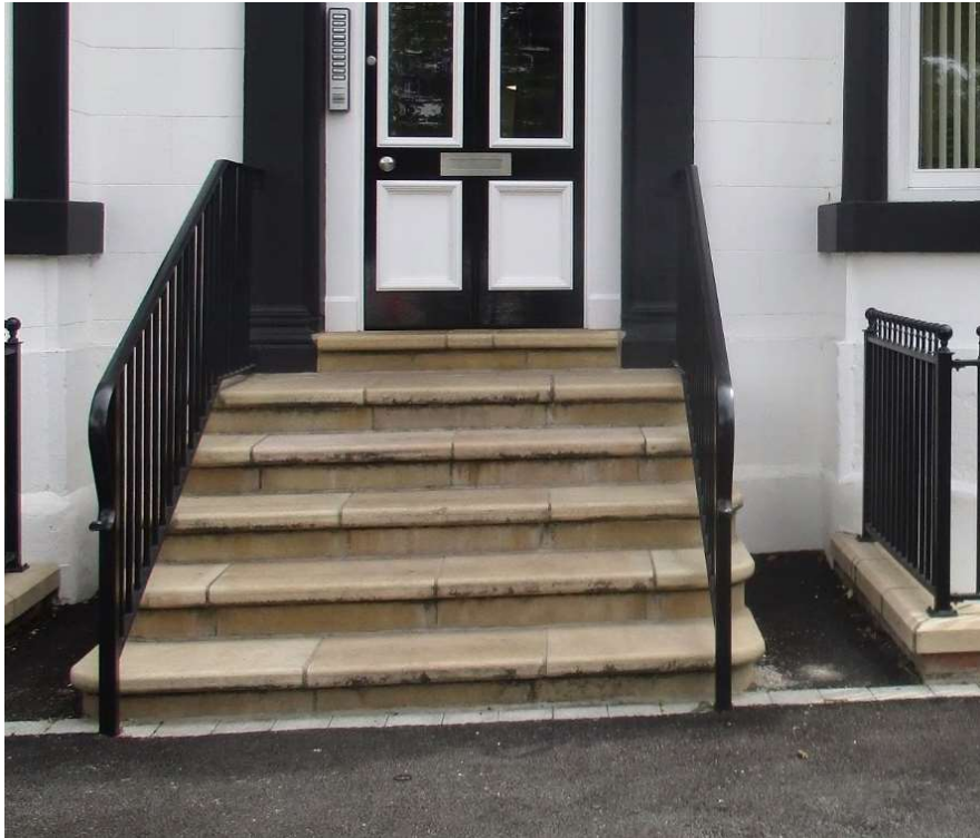
Fig 9. Existing front entrance showing new steps and handrail with joints visible.
