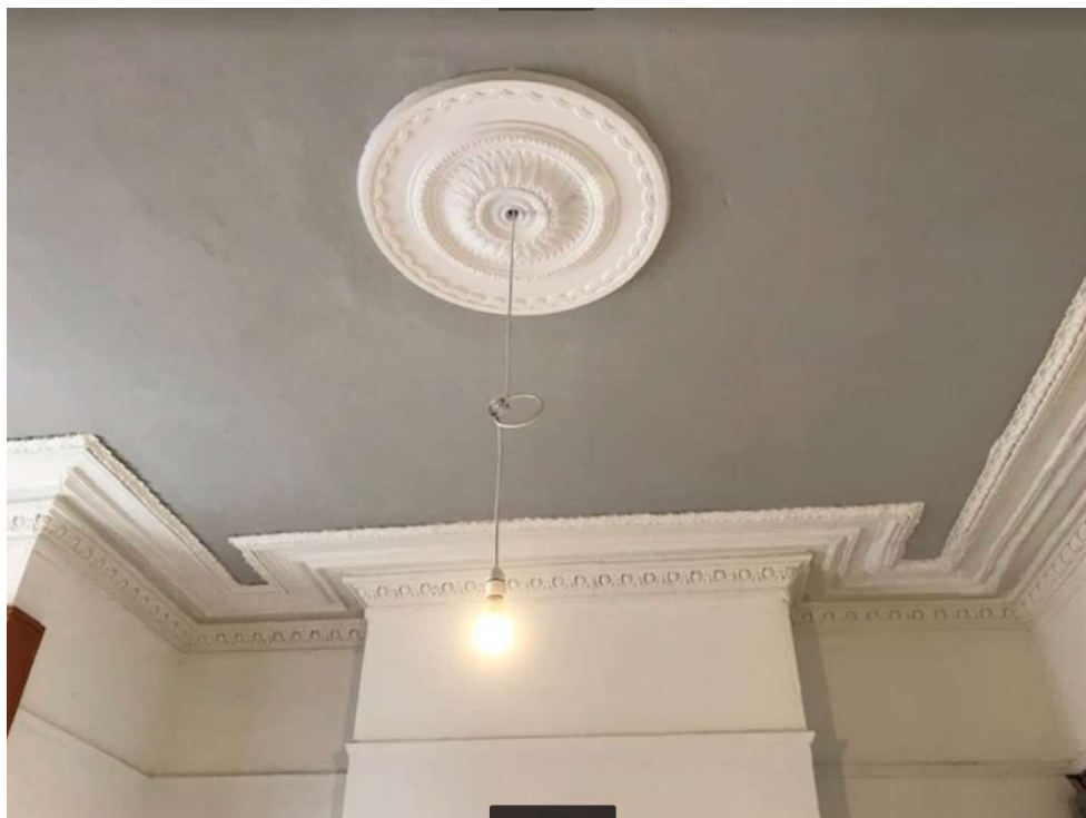
Fig 25. Internal decorative cornice and picture rail to 359 following restoration.
