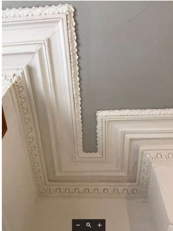
Fig 24. Internal decorative cornice to 359 following restoration.
