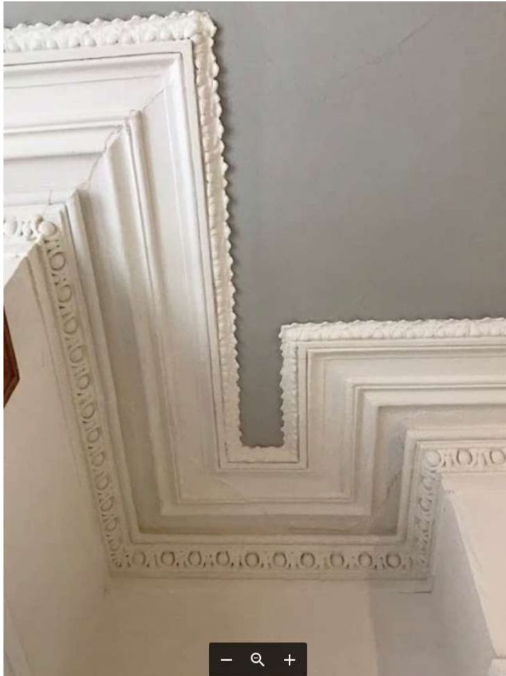
Fig 3. Internal decorative cornice to 359 following restoration.
