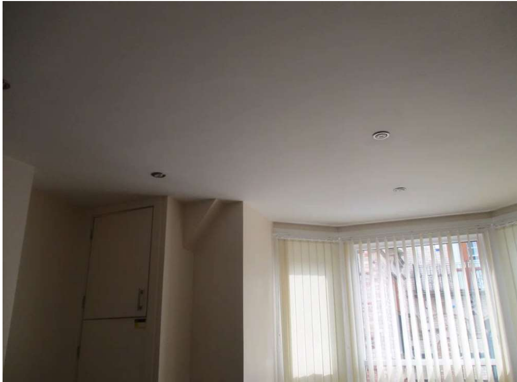
Fig 6. Internal side room of 363 with bay window showing lowered ceiling and loss of original height, cornice and timber panelling.
