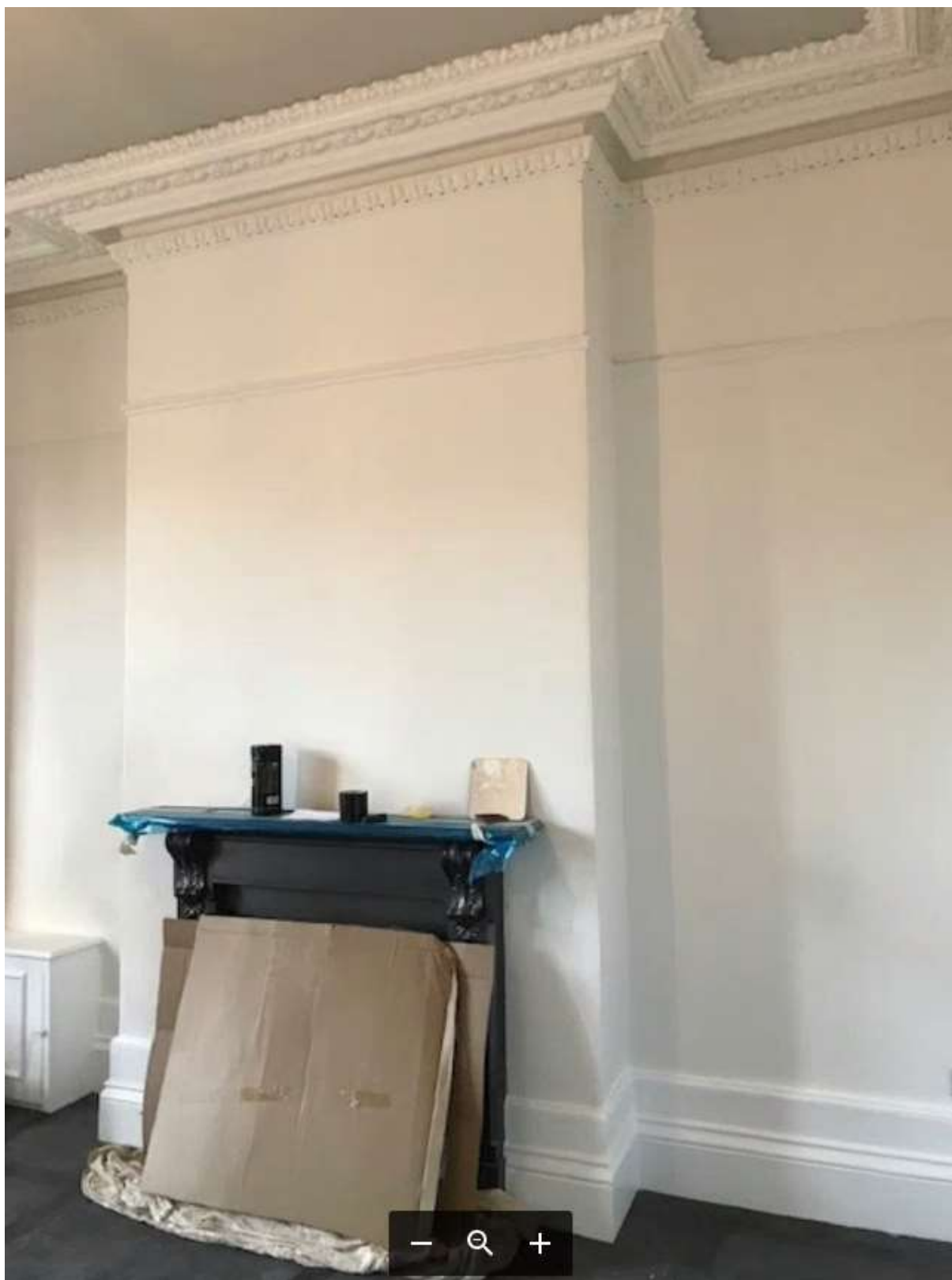
Fig 26. Internal decorative cornice, picture rail and skirting to 359 following restoration.
