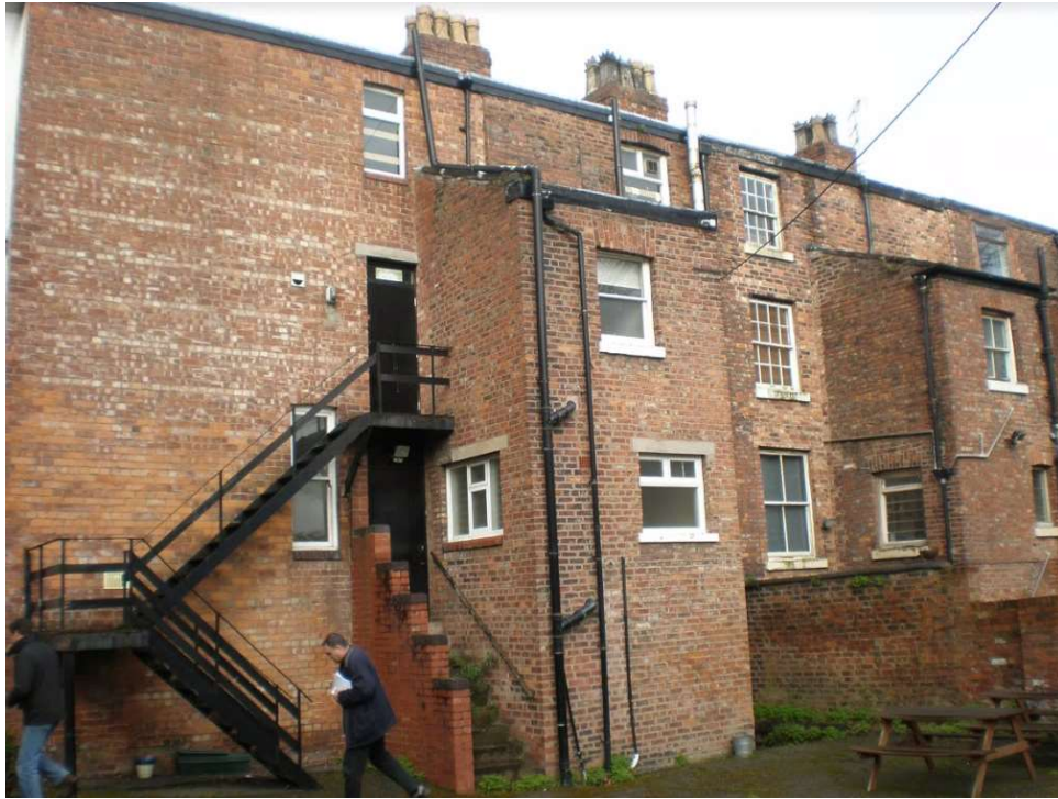
Fig 16c. The rear of No.363 taken in March 2014 prior to the unauthorised removal of the outrigger. Noting that the scale of the lean-to was the same as 361 and 359 as is the scale of the windows.
