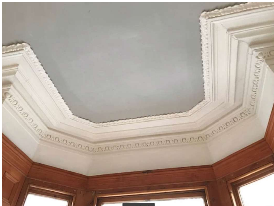
Fig 2. Interior room of 359 Wilmslow Road showing restored decorative cornice and restored timber panelling and shutters.
