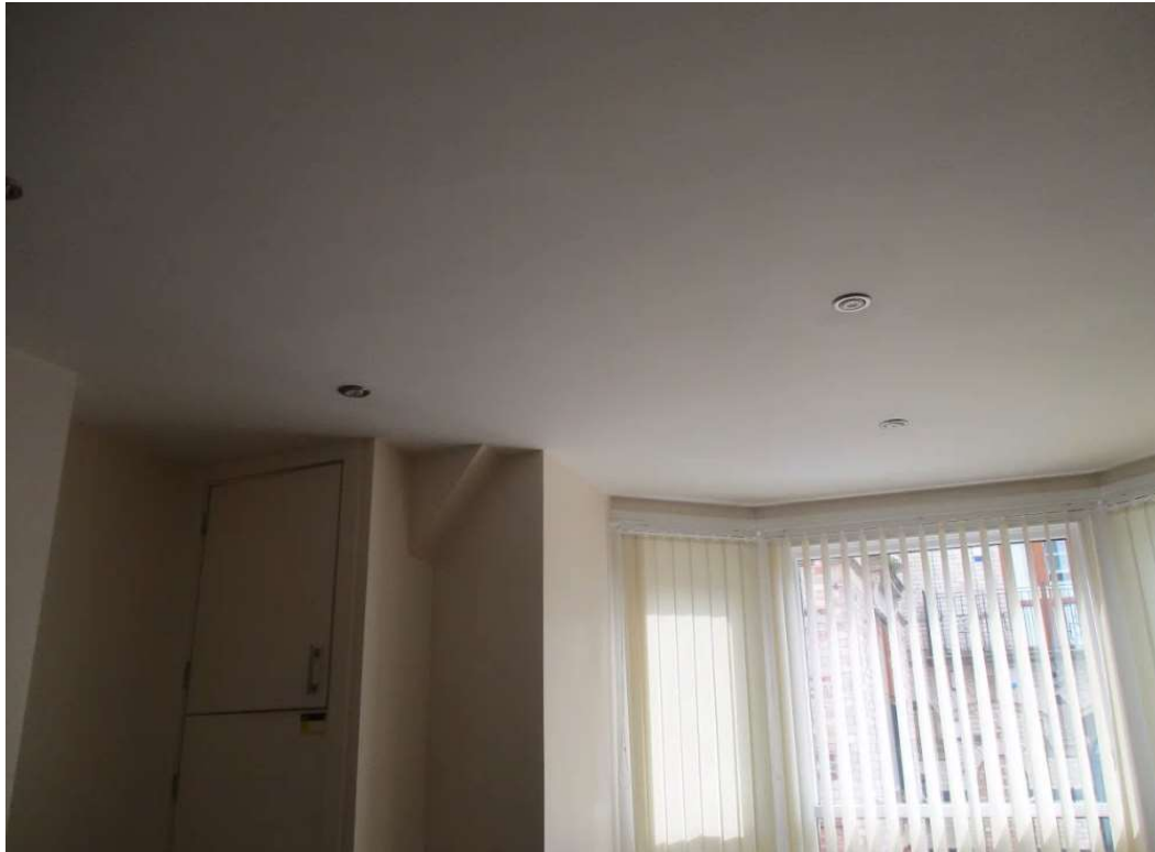
Fig 29. Internal side room of 363 with bay window showing lowered ceiling and loss of original height, cornice and timber panelling.
