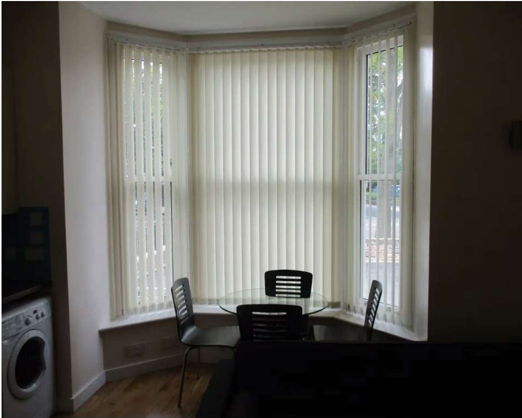
Fig 27. Internal front bay window to No. 363 showing removal timber panelling and lowered ceiling and subsequent loss of detailing and features.
