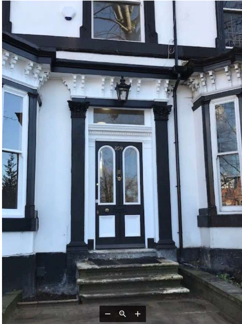
Fig 11. Front entrance of No. 359 showing the natural stone steps and authenticity and aesthetic value of the complete entrance design.
