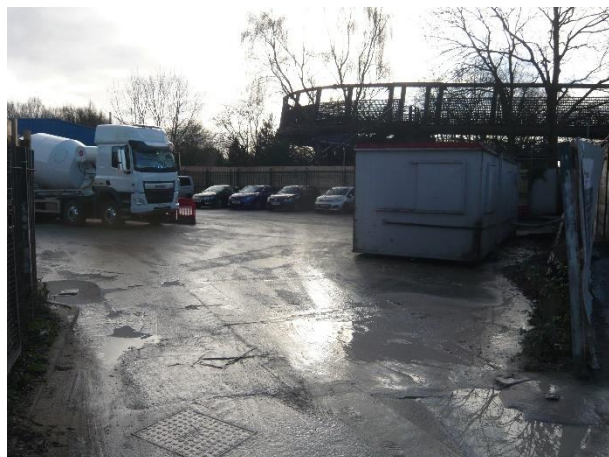
Photo 1: Hard standing at concrete batching plant
