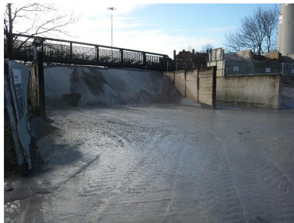
Photo 2: Hard standing at concrete batching plant
