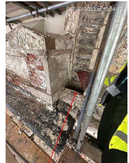
Section of ply cover removed.
