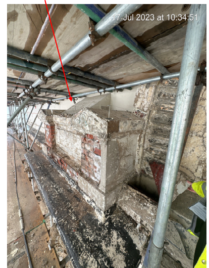
Projection with ventilation cover.
