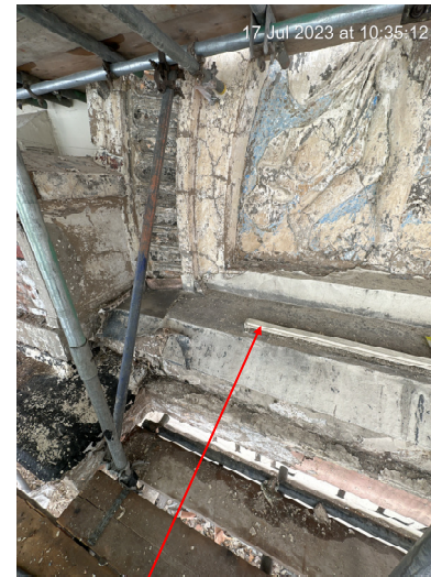
A built-in box gutter with a deteriorating ply cover.
