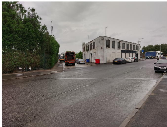
Site from junction of Redgate Lane and Copping Street
