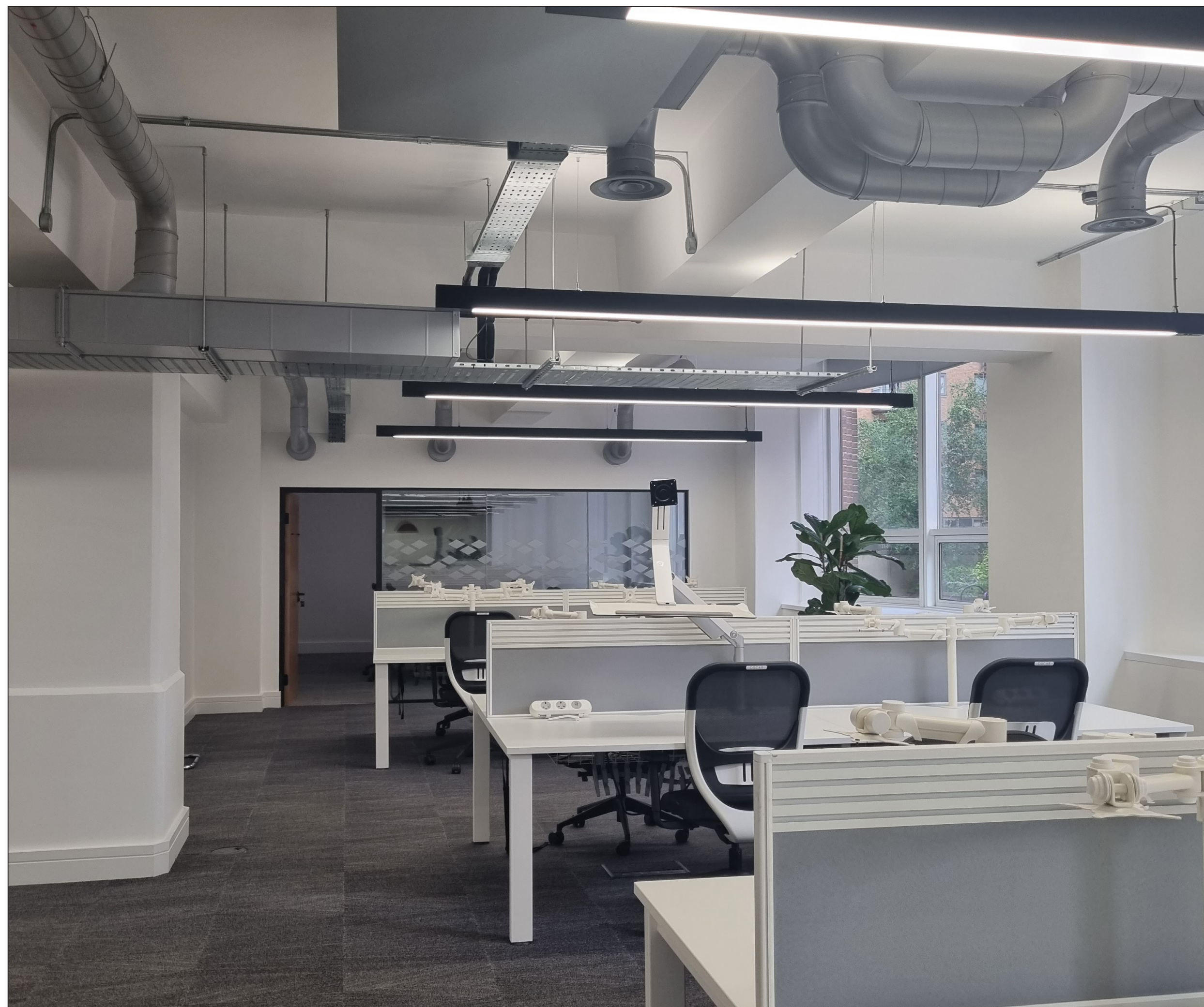
Internal view of existing space, first floor, showing columns.
