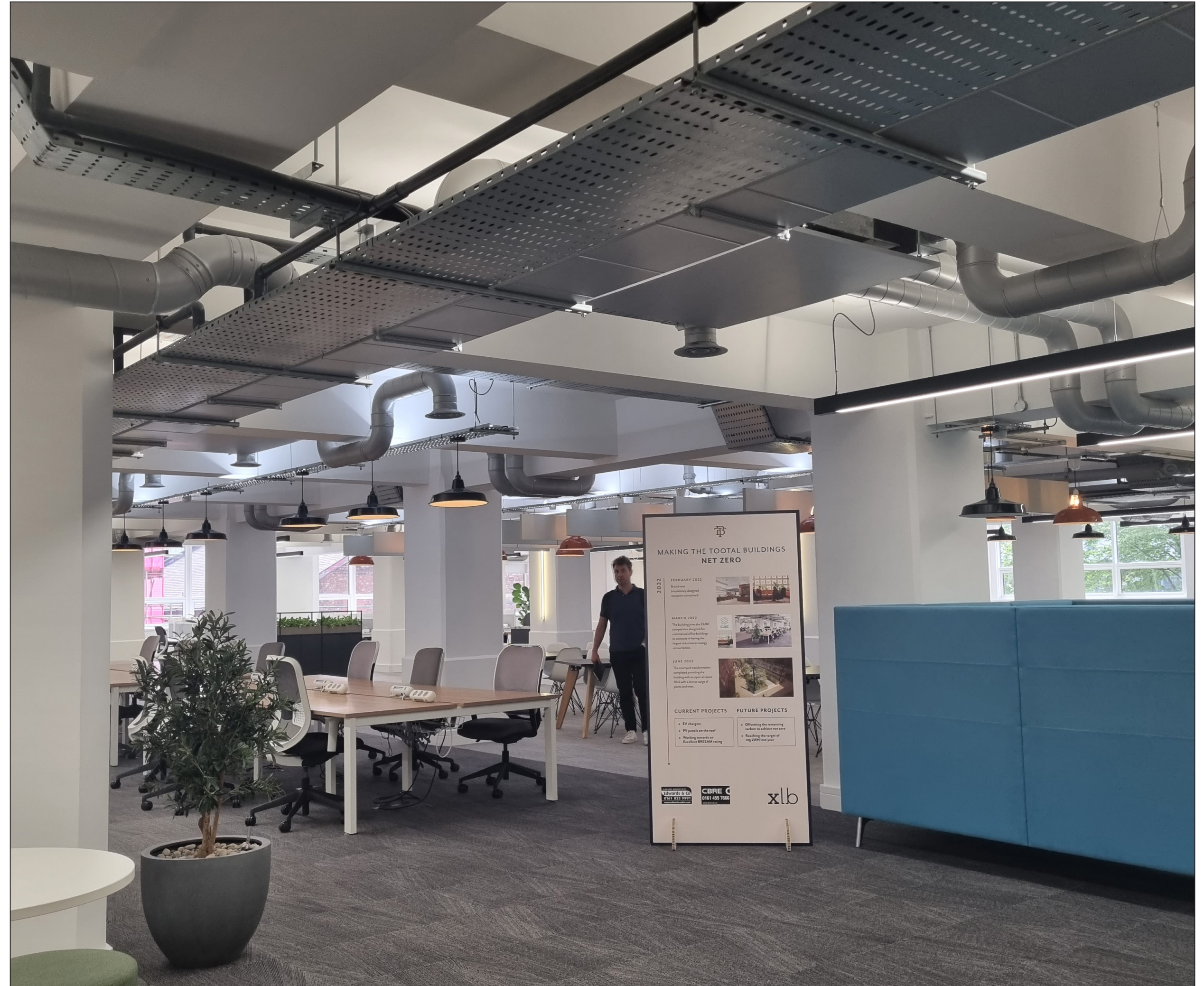
Internal view of existing space, first floor, showing M and E arrangement.
