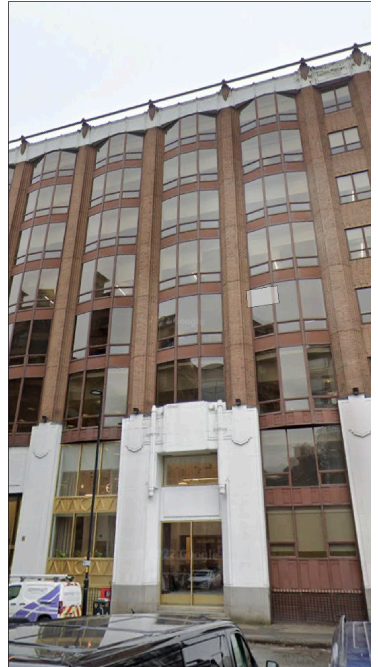
Photograph of exterior of Lee House, main entrance.
