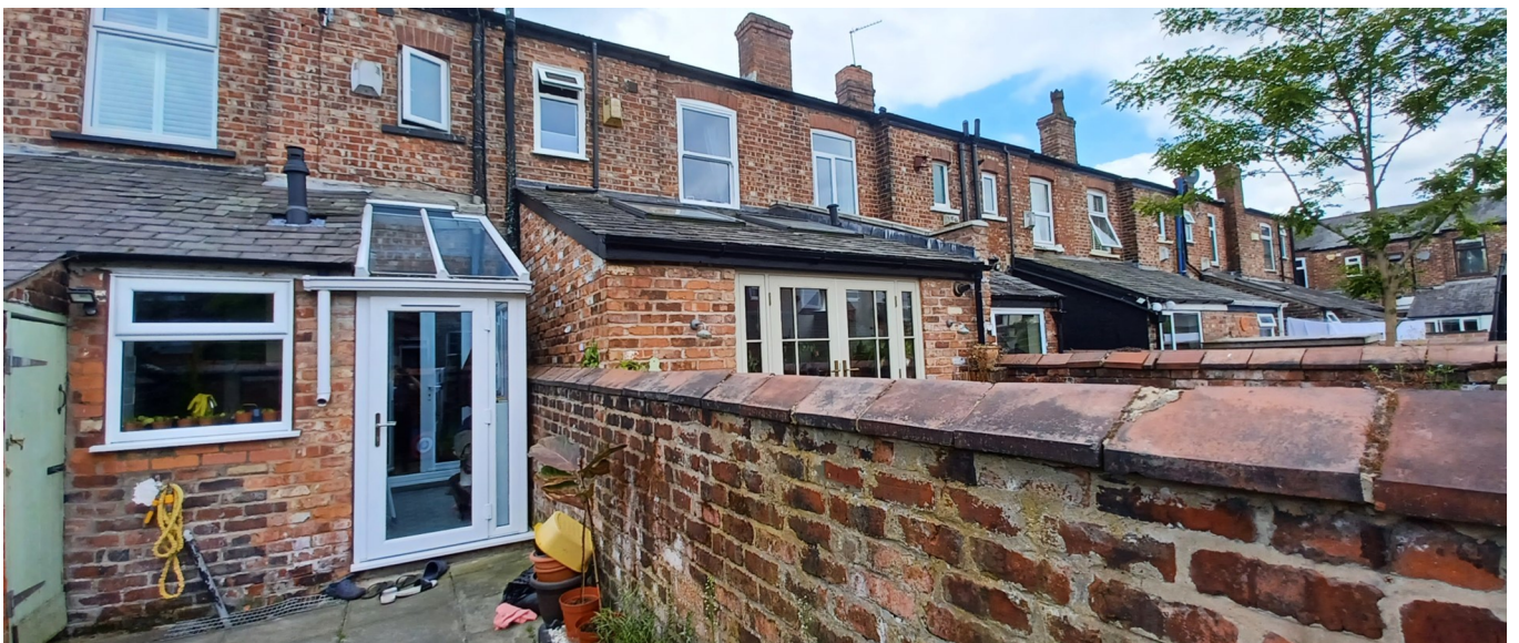
Figure 3. Similar rear extensions along Eleanor Road.
