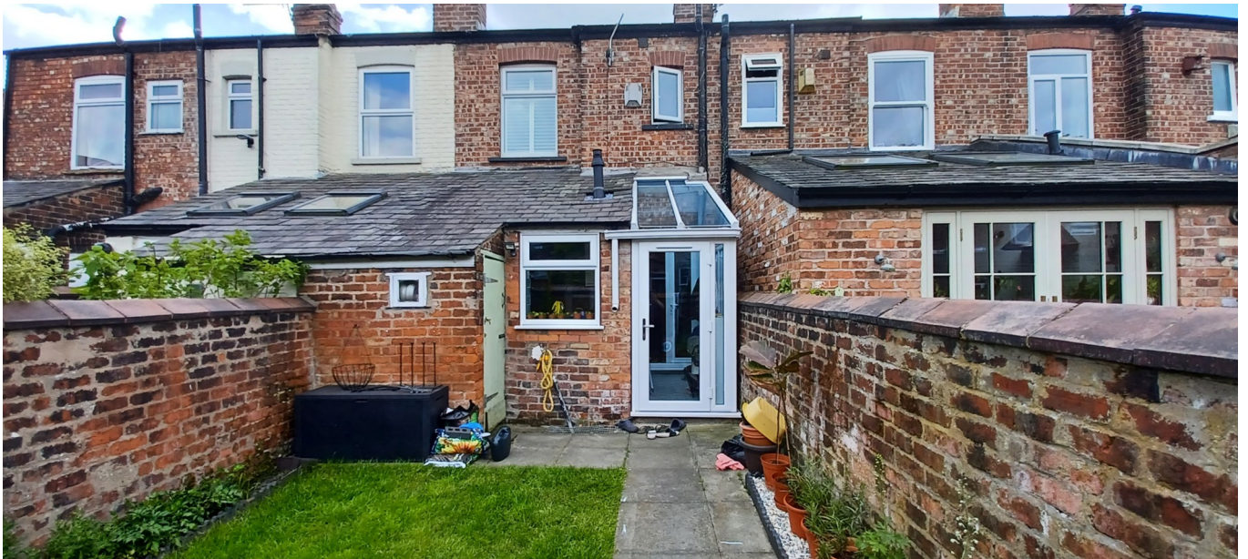
Figure 2. Rear of property.
