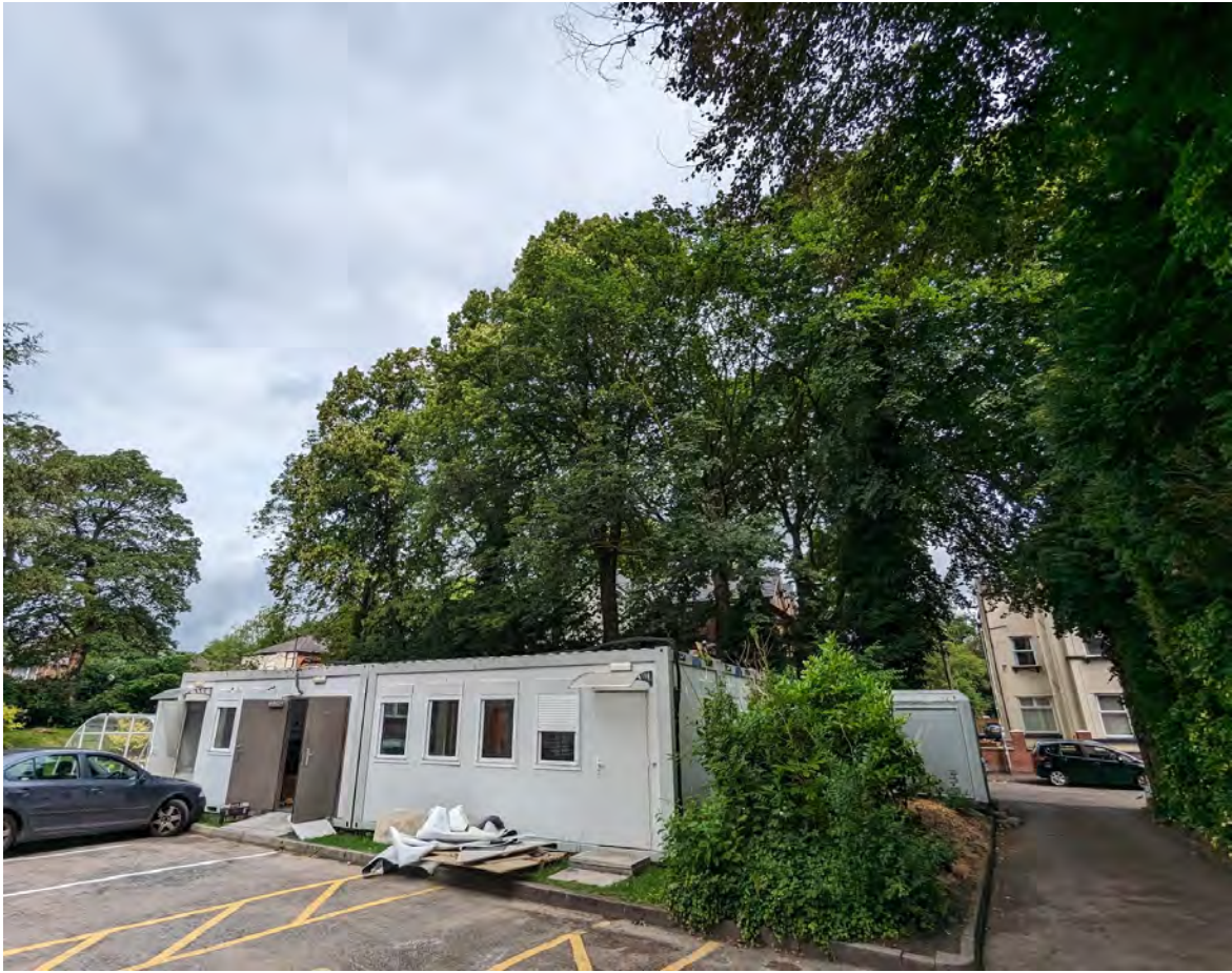
Photographic plate showing T7 to T19 located directly behind the recently implemented modular classrooms.
