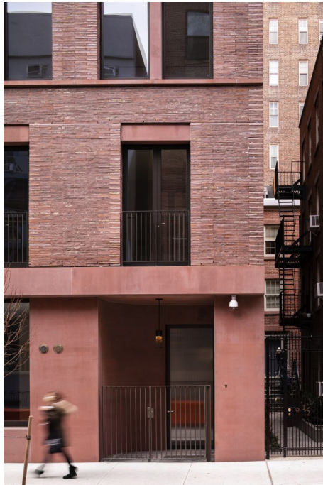
Matching red sandstone and brick detail
