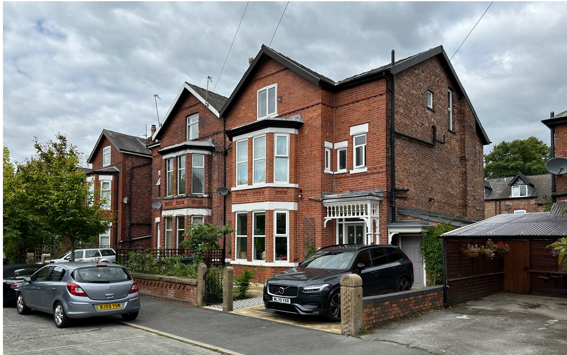
Existing site photograph
